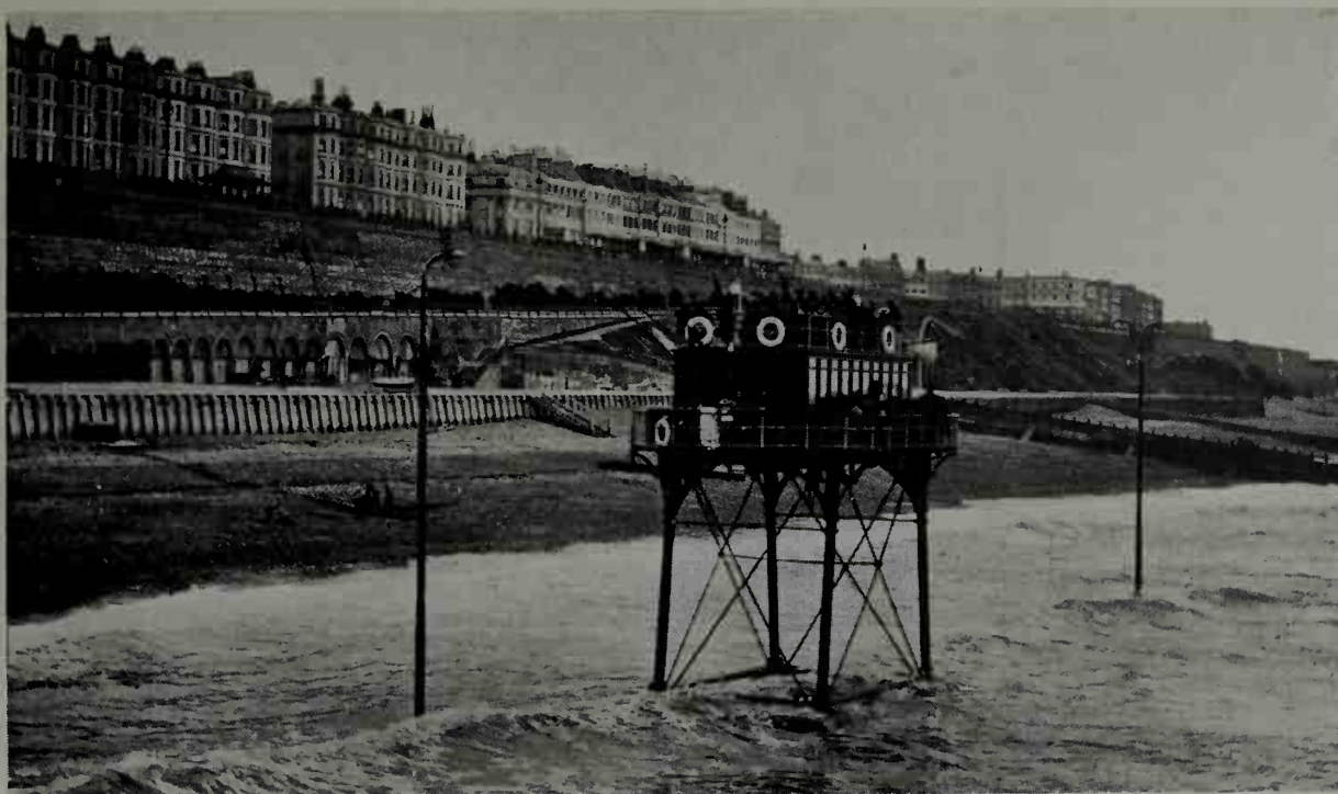
198. Briefly at the end of last century, Volk's Electric Railway in Brighton ran a line on the beach itself, between the tidemarks, from the Banjo Groyne to Rottingdean. The car ran on parallel tracks and was served by two wires like the trolleybus of later years. Like a ship, it carried a lifeboat.
