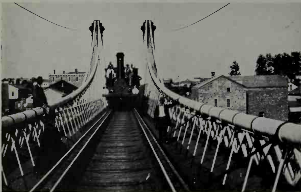
125. Mid-Victorian Canada: A view along the international suspension bridge at Niagara in the 'sixties. It was laid with mixed gauge, and a special light locomotive of the broad-gauge Great Western Railway of Canada took the cars across.
