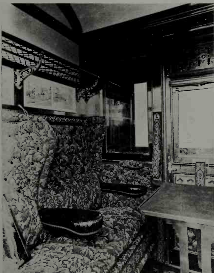
160. A Great Central corridor first-class of 1899. Noteworthy were the semi-elliptical false roof, the generous armrests, and the well-meant but clumsy arrangement of the table across the door on the corridor side.
