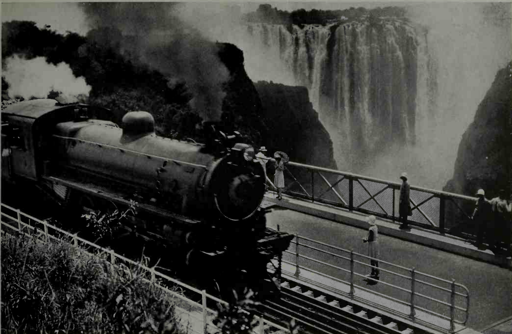
226. There are many larger bridges than that of the Rhodesia Railways across the Zambesi, but few in a more terrific situation. This view was taken in the late nineteen-twenties, just after the addition of a motor road beside the single-track railway. The single steel arch is 500 ft long, and the height above the water 420 ft.
