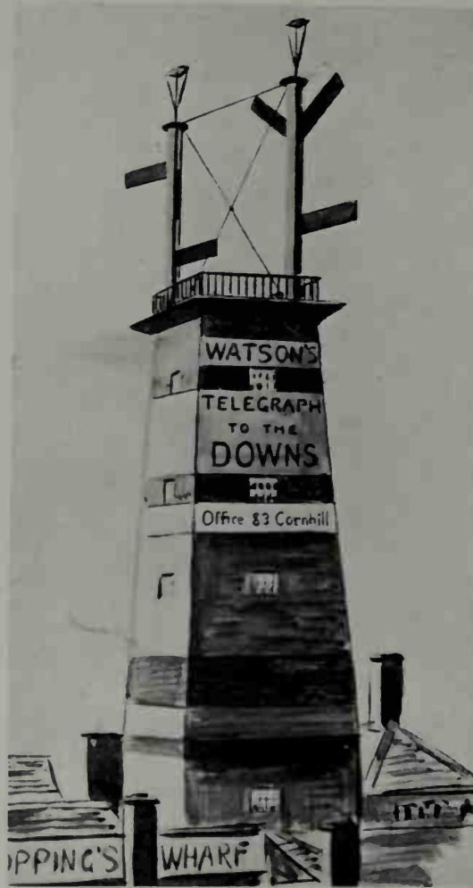
23-5. Primitive railway signalling was by police hand signals, though the semaphore was already well-known, invented by Chappe in the late eighteenth century as an early form of telegraph (the oldest was either the smoke signal or the drum). In the middle is Watson's semaphore telegraph station near London Bridge. It was destroyed in the Tooley Street fire of 1843. On the right is one of Gregory's first railway semaphores on the London and Croydon Railway at the beginning of the eighteen-forties.
