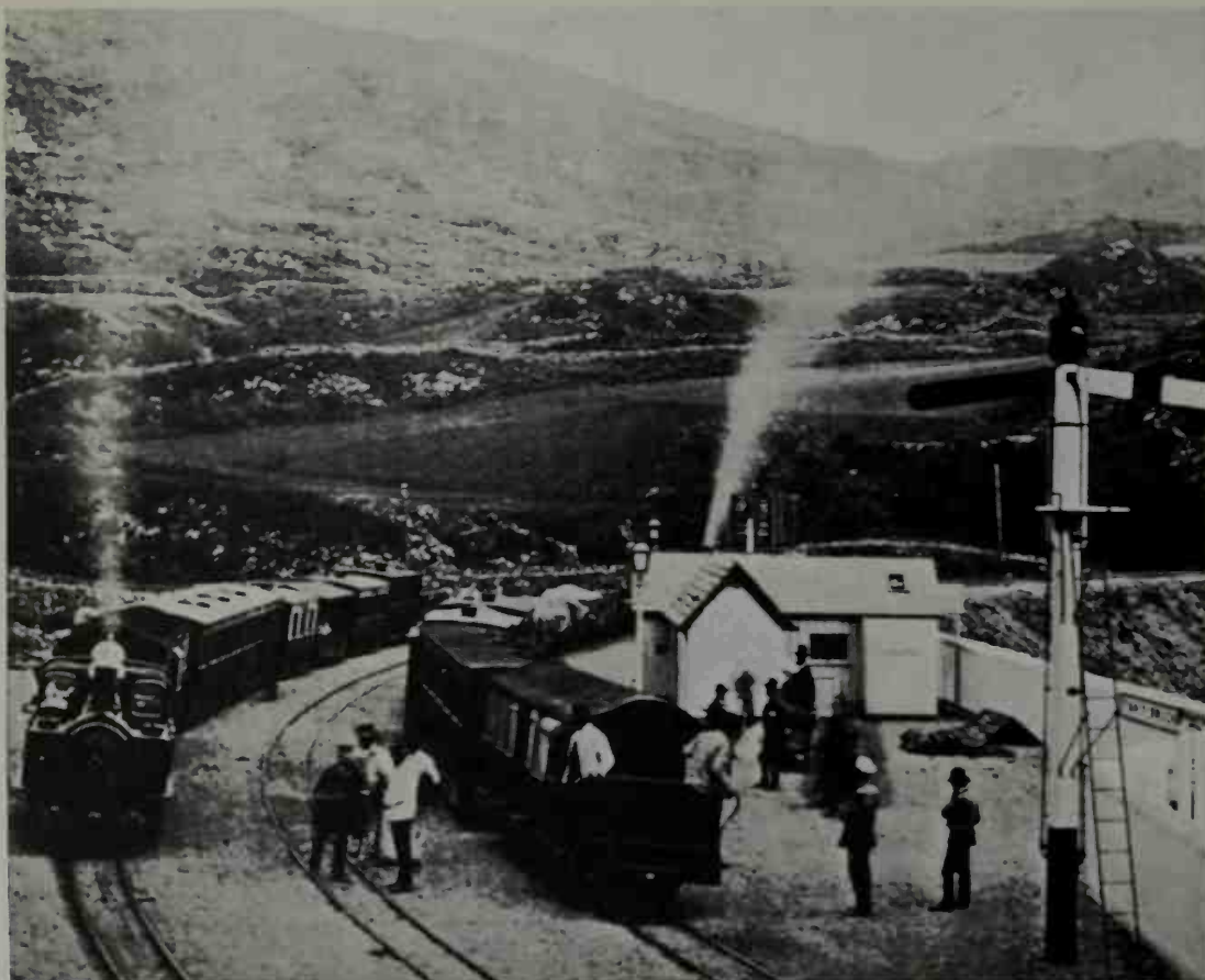
168-9. Narrow-gauge: Britain's oldest public narrow-gauge railway (1 ft. 11½ in.), between Portmadoc and Blaenau ffestiniog, was opened in 1836, and was worked by horses and gravity until 1863. The left view shows trains crossing at Tan-y-bwlch in the 'seventies, with a double Fairlie locomotive ( James Spooner ) on the left. On the right is a summer idyll on the Tal-y-llyn Railway (1865) with a disputant—a lady.
