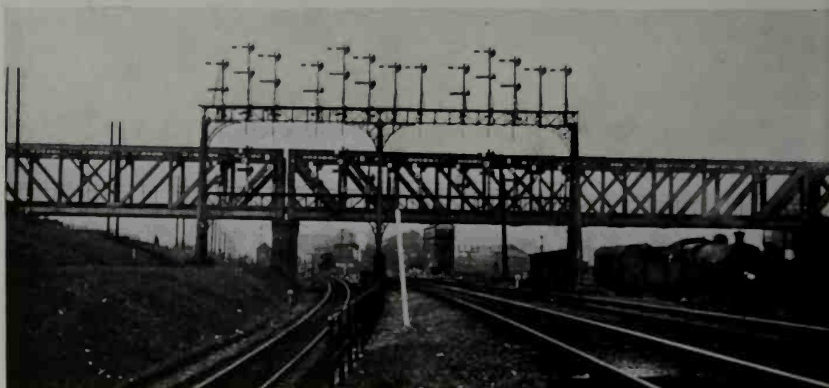
378. Signal gantry at the south end of Rugby, London and North Western Railway. The semaphores were duplicated, in two ranges, owing to interference by the bridge carrying the Great Central main line.
