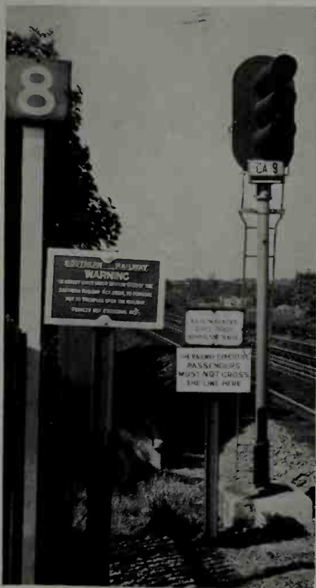
381-3. Colour-light signalling, separate from the use of semaphores, is an idea of some antiquity, but automatic electric installations on a large scale belong to our own time, like the signalling of road crossings. On the left is the up starter at Wivelsfield on the Brighton main line; in the centre are up starters at Brighton; on the right is a bracket signal at Bristol Temple Meads. Unlike semaphores, they are not photogenic. Light, shade, steam and the skill of Mr. Heiron make the right-hand view, in which a British Railways standard 4-6-0 heads an up fast goods.
