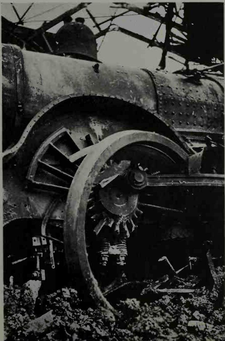
357. (Left) Not every locomotive will survive a high explosive bomb that comes through the boiler and firebox, and bursts under the crank axle. This old T9, ex-London and South Western, did so at Fratton on January 12, 1941. Dugald Drummond's locomotives, it has been said, were built like battleships. The only sure way to destroy one was systematically to take it to pieces and then break up those.
