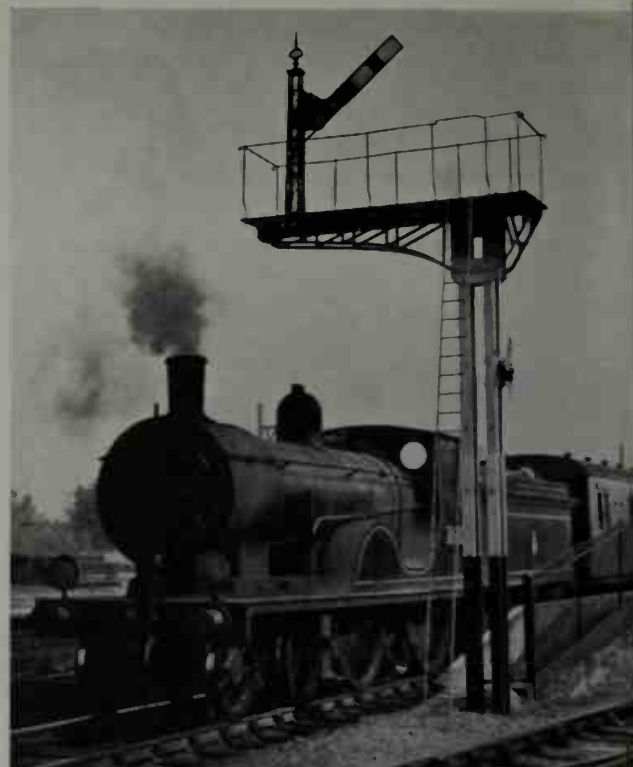
376-7. From earliest days, British signalling methods and equipment led the world. This was the old manual signalbox at Liverpool Street on the Great Eastern, which contained 165 levers, controlled the most intensive traffic in the world, and was worked by three men. Later semaphores work in the upper quadrant, except on the former Great Western lines. This is in the Southern Region at Farnborough North.
