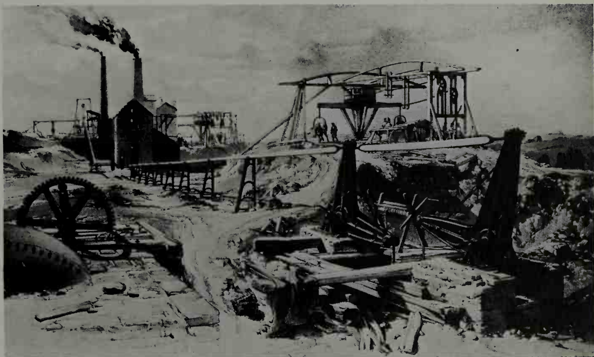
29. In the construction of Kilsby Tunnel on the London and Birmingham Railway, the works encountered a quicksand, and the contractor died of shock. Robert Stephenson took over. This view shows the steam pumps he installed to deal with the flooded workings. Beyond is a large horse-gin for haulage.
