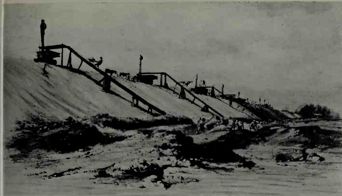
28. London and Birmingham Railway: Boxmoor Cutting being excavated. Horse-gins pulled the barrows to the top while the navvies steered, an extremely hazardous process.
