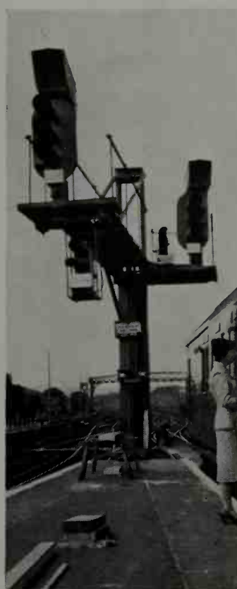
381-3. Colour-light signalling, separate from the use of semaphores, is an idea of some antiquity, but automatic electric installations on a large scale belong to our own time, like the signalling of road crossings. On the left is the up starter at Wivelsfield on the Brighton main line; in the centre are up starters at Brighton; on the right is a bracket signal at Bristol Temple Meads. Unlike semaphores, they are not photogenic. Light, shade, steam and the skill of Mr. Heiron make the right-hand view, in which a British Railways standard 4-6-0 heads an up fast goods.
