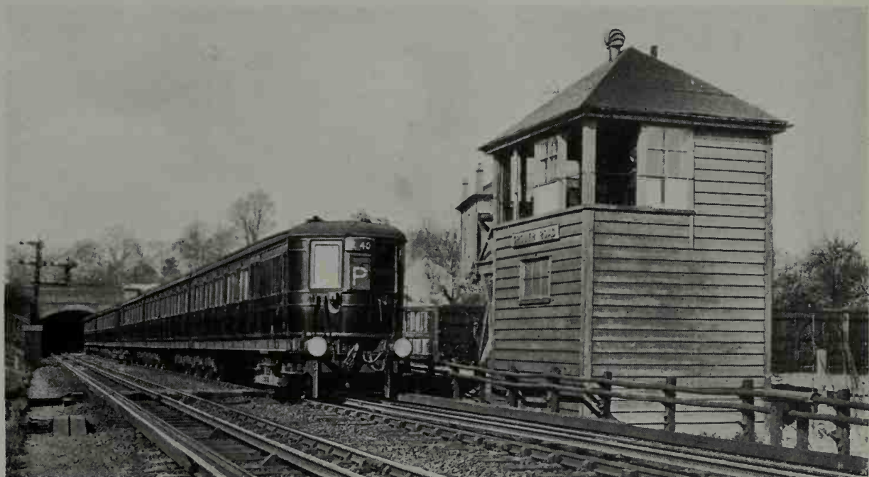
304-6. First of the Southern companies to electrify a steam line was the London, Brighton and South Coast, which used alternating current with overhead conductors, on the South London line in 1909, and subsequently on the Crystal Palace group of lines. The London and South Western, from 1915 onwards, used d.c. with third-rail contact, and the middle view shows one of its trains at that time, between East Putney and Southfields. The fourth-rail return was for the accommodation of underground electric trains off the District Railway, which had been running over the L.S.W.R. since 1905. The South Western's system was eventually adopted for all the Southern Railway. The lower view was taken at Ascot in 1938 and shows one of the L.S.W.R. Drummond tank engines with its austere successor.
