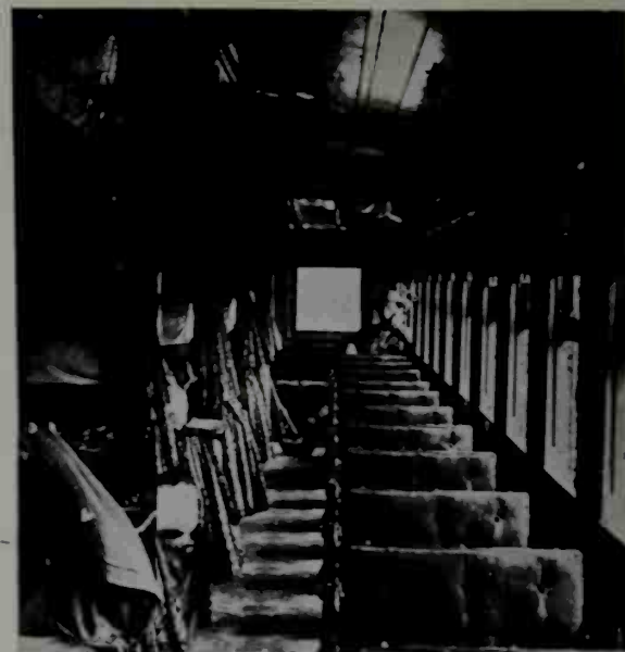
126. Before it patronised Mr. Pullman, the G.W.R. (C.) had its own ideas about sleeping cars, which it ran in the night trains across Ontario. The cars were made as wide as possible, with three tiers of berths on one side of the aisle, and ordinary day-coach seats on the other.
