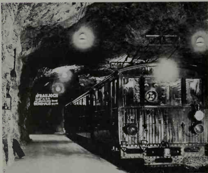
277. The Abt system, unlike that of Riggenbach, employed two parallel racks with the teeth staggered, and was widely adopted on Swiss mountain railways, including the Jungfrau Railway. This, at Jungfraujoch, has the highest station in Europe, 11,340 ft. above sea level.
