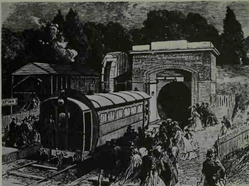
103. Deep level: The Metropolitan Railway was but a year old when experiments were begun with what, in later years, has been called a tube railway. In 1864, at the Crystal Palace, such a line was demonstrated, with the car puffed through the tube like a pellet, under air pressure. It was at least a brave attempt, and the principle was used for conveyance of mailbags by the Pneumatic Dispatch Company.
