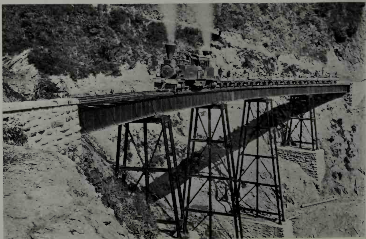
220. In Central America, the Mexican Railway was British. For many years it used Fairlie double-bogie engines on its mountain division. One of the earliest, a very obvious wood-burner, is here shown on a construction train.
