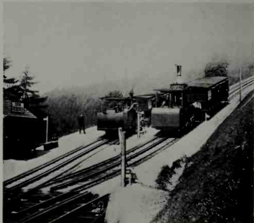
276. Most famous of mountain railways built on the Riggenbach system was the Vitznau-Rigi Railway by Lake Lucerne, partly opened in 1871 and, throughout, in 1873. Vertical boilers were used for the earlier locomotives. This view of Freibergen station, with trains crossing, shows one engine rebuilt and the other with the old boiler, also the sector table used instead of points.
