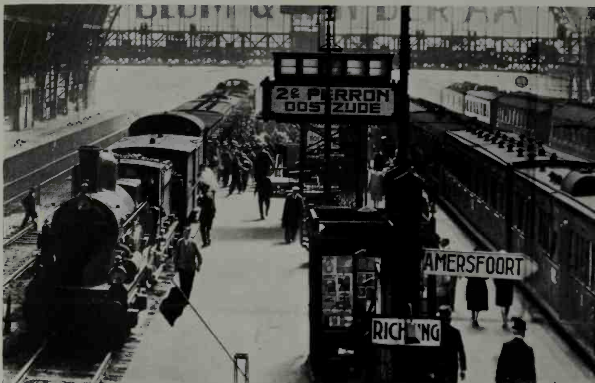
247. Amsterdam Central: High platforms and the old Beyer Peacock seven-footer bespeak English influence; the flat-roofed side-door carriages could be nothing but Old Dutch. This view was taken in 1929.
