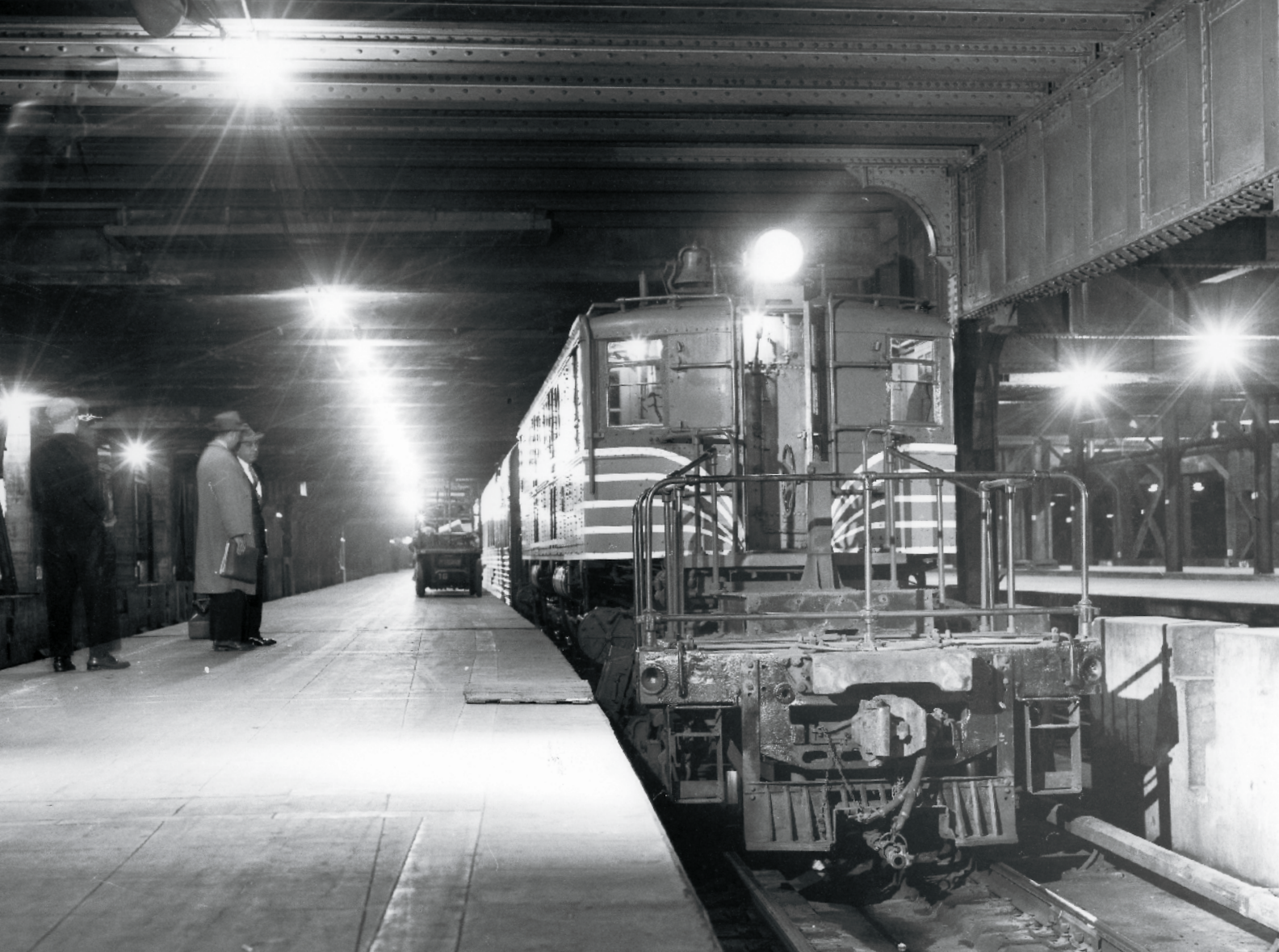
Across town from and many vertical feet below the elevated West Side freight line, P-2 electric 235 waits at Grand Central with train 65, the Advance Commodore Vanderbilt for Chicago. Long-distance trains stopped using the terminal when the West Side Connector opened in 1991.
