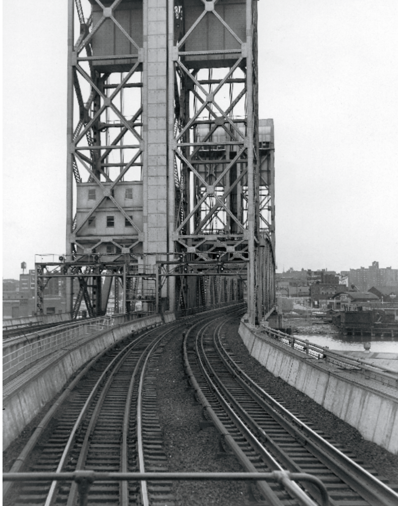
The Central's new Harlem River lift bridge was only about a year old when Shaughnessy's train crossed it on April 13, 1957. It replaced an 1893 swing span.
