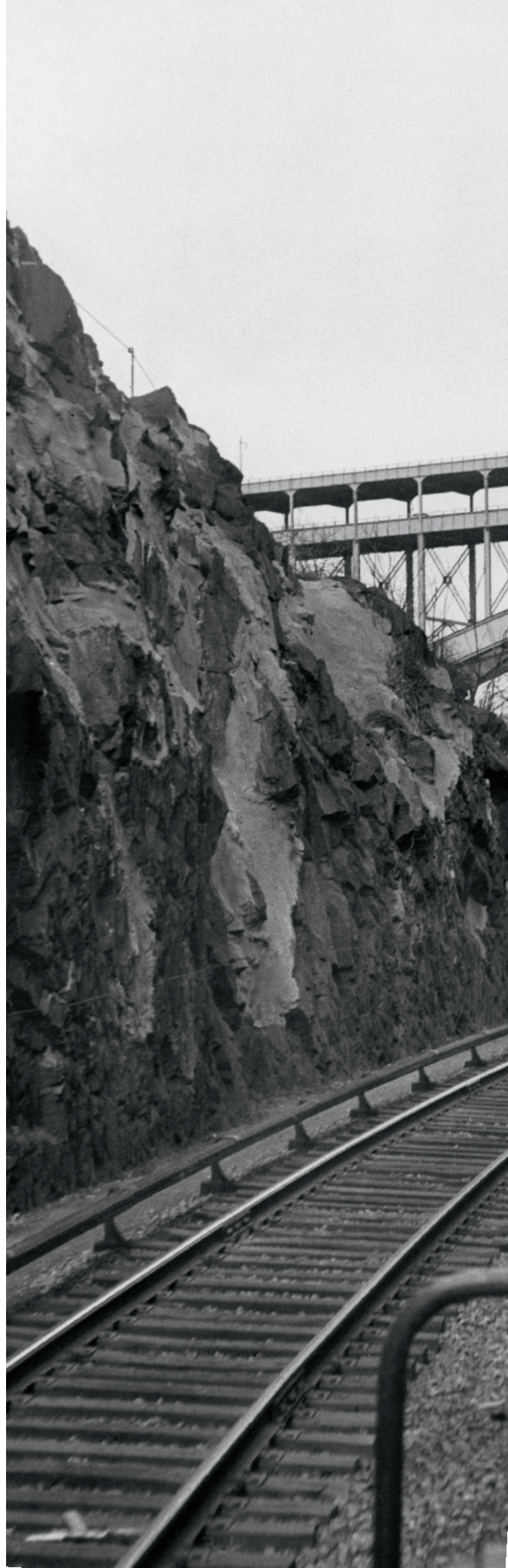
The Central's new Harlem River lift bridge was only about a year old when Shaughnessy's train crossed it on April 13, 1957. It replaced an 1893 swing span.
