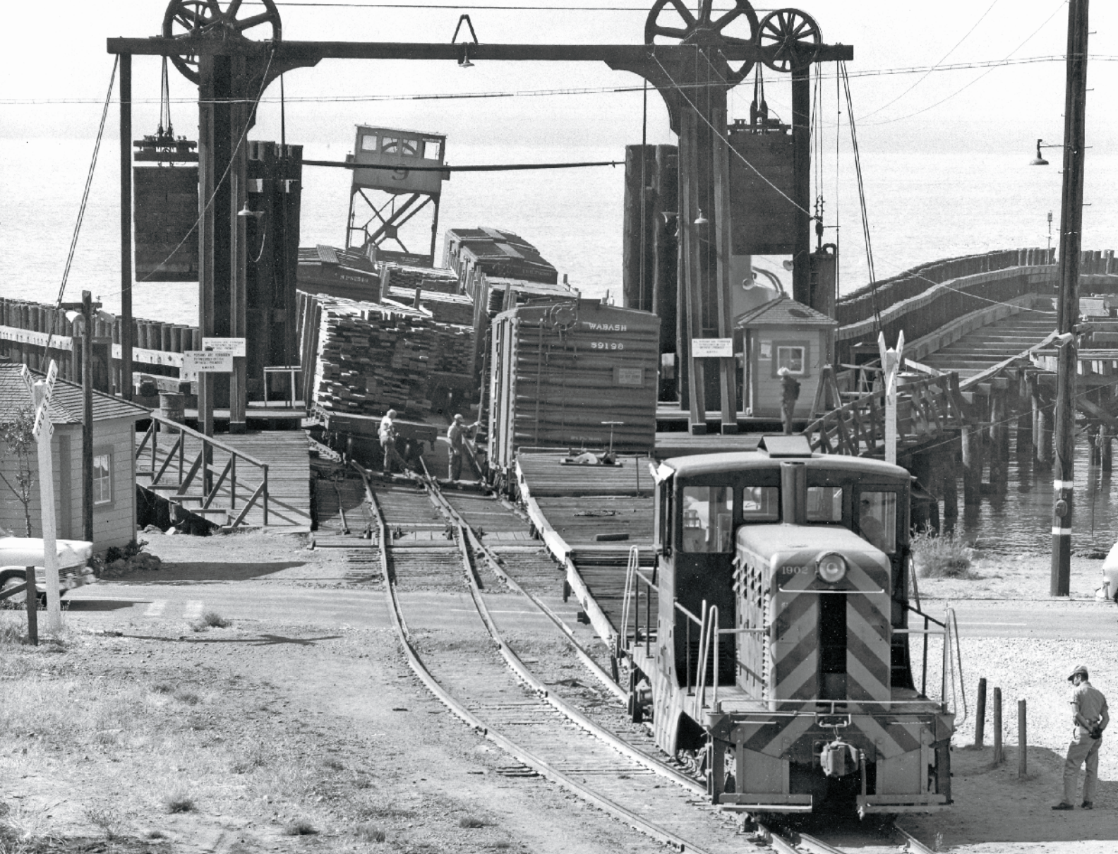
Like Western Pacific and Santa Fe, Southern Pacific also floated freight cars across San Francisco Bay. In the mid-1950s at Tiburon — in Marin County north of the Golden Gate Bridge — GE 44-tonner No. 1902 loads a barge at the slip of SP subsidiary Northwestern Pacific.
