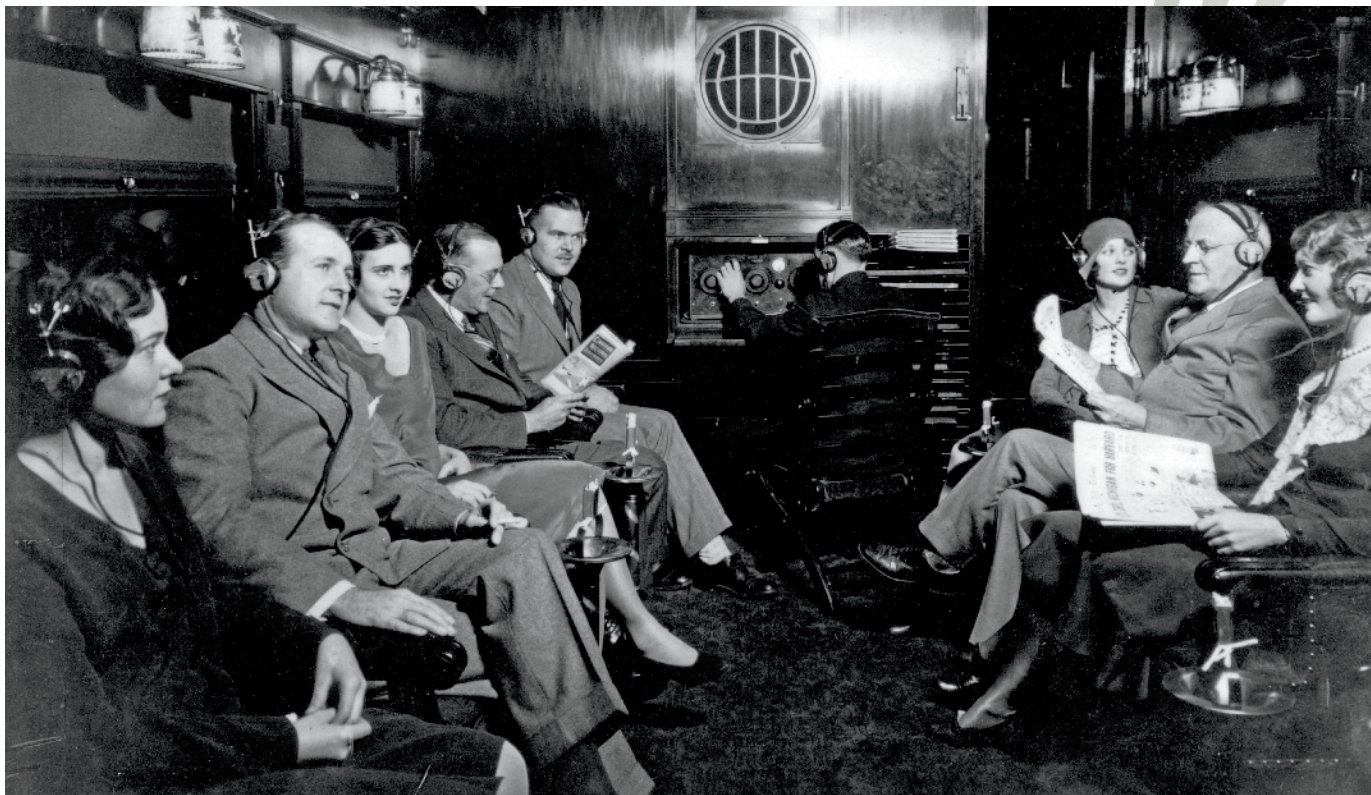
Observation-lounge cars assigned to 16 CNR name trains were fitted with receiving equipment, speakers, and headsets so passengers could listen to radio broadcasts during their journey — a unique attraction in radio-crazy 1929. An employee operated the receiver console.
