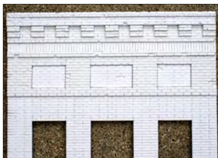
6. Brick cornice and corbels were applied, and mortar lines brought around the corners.
