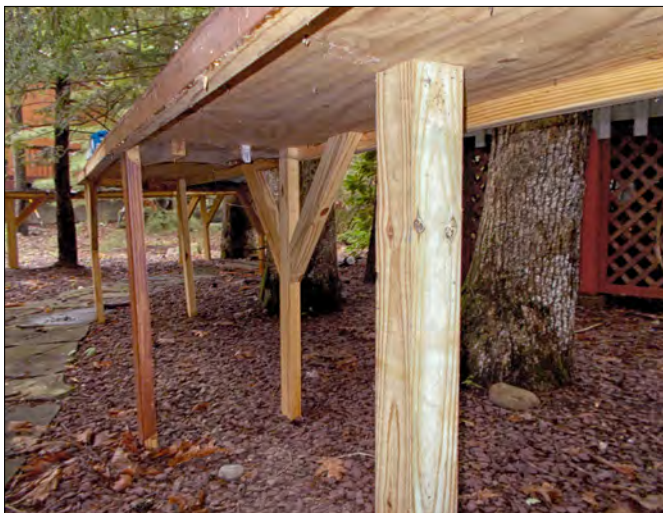
The underside of the tables, showing the construction. Gravity alone keeps everything in place; the railroad is not anchored to the ground.
