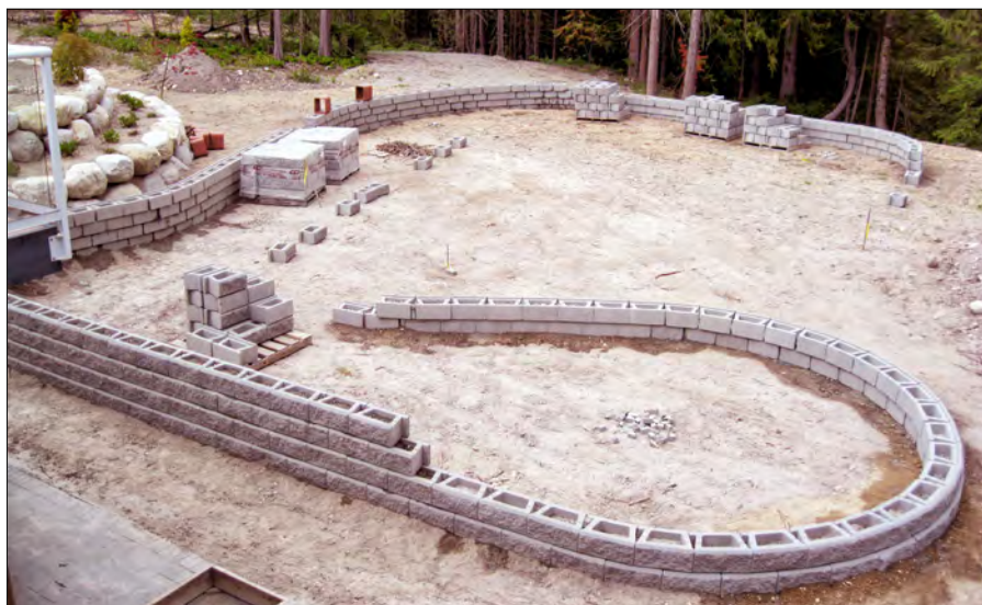
3. An overall view of the railway 21 days into construction in August 2011. The red chimney flues form the tunnel liner. Level stacking blocks form a solid foundation for the easy-reach railroad bed on the perimeter. PHOTO BY PAUL GARRETT
