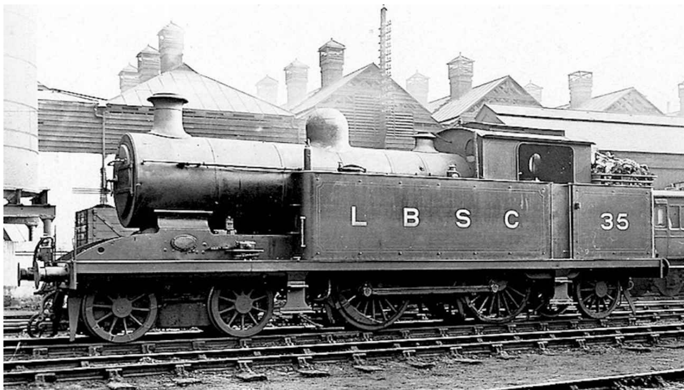
The last numerical member of the I2 class was N° 35, which is seen at Brighton depot with the abbreviated version of the owning companies name – having the ampersand and the R removed. By this time the brakes, which had previously been fitted to the bogie, had been removed. (Author's Collection)
