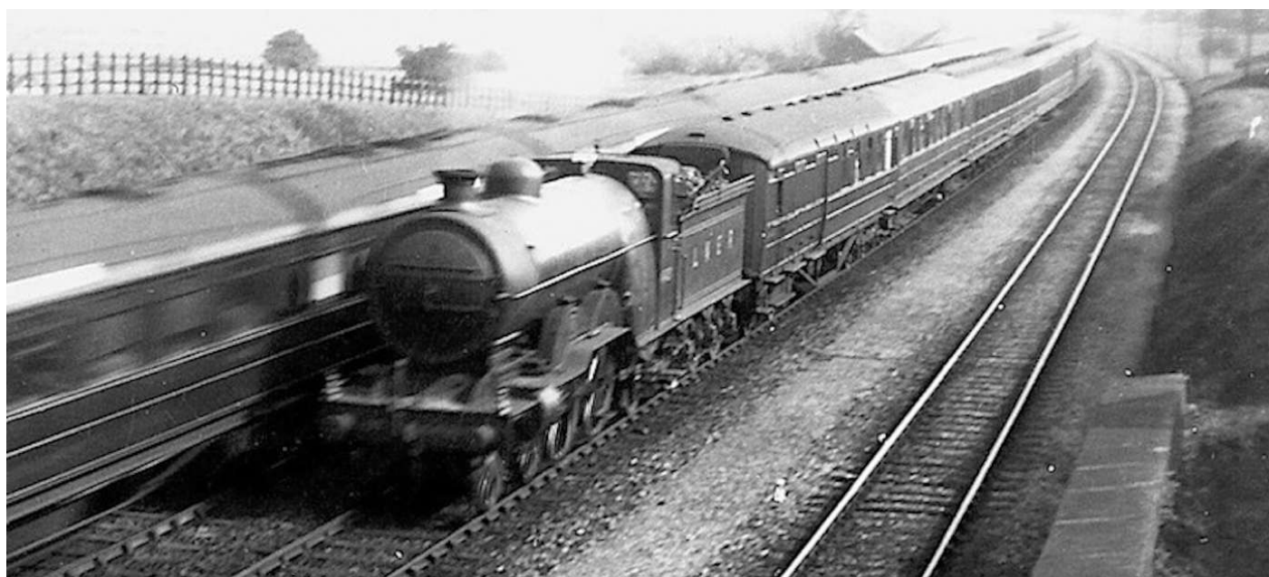
Although ten small boiler Atlantics were built in 1903, the major effort in constructing engines for use on express passenger engines was confined to those of the 'big-brother' version – the large boiler Atlantics, of which ninety-four examples were built between 1902-10. Here is a large boiler Atlantic doing what it was designed to do – working a heavy teak-bodied express passenger service at speed. (Author's Collection)
