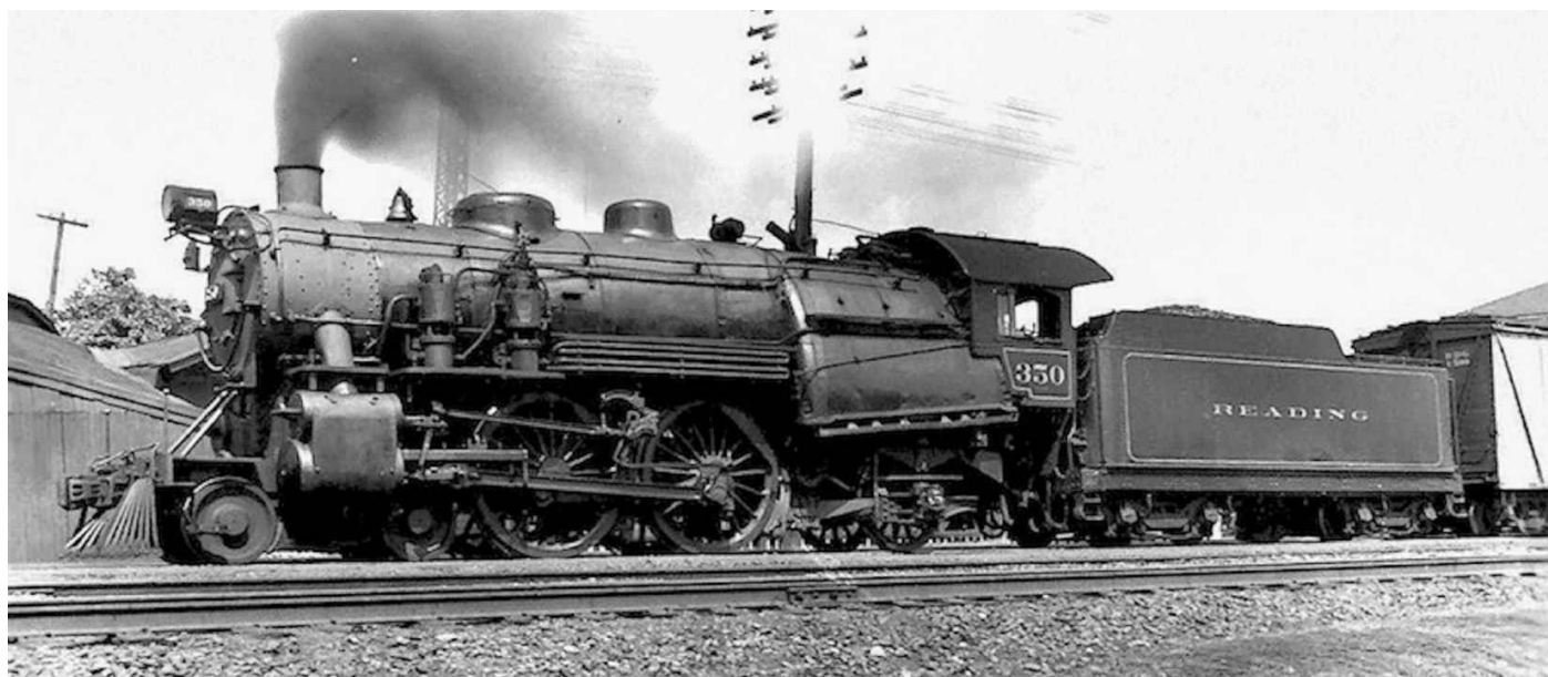
In the early 1890s , many American railroads adopted the 4-4-2 Atlantic wheel arrangement, as these engines provided a fast and reliable service to such places as Atlantic City and New Jersey. Here is N° 350, a 4-4-2 Atlantic built for the Pennsylvania-Reading Seashore Lines. The photo shows the 4-4-2 Atlantic wheel arrangement and the wide Wooten style firebox, which gave inspiration to the GNR Atlantics. (Author's Collection)
