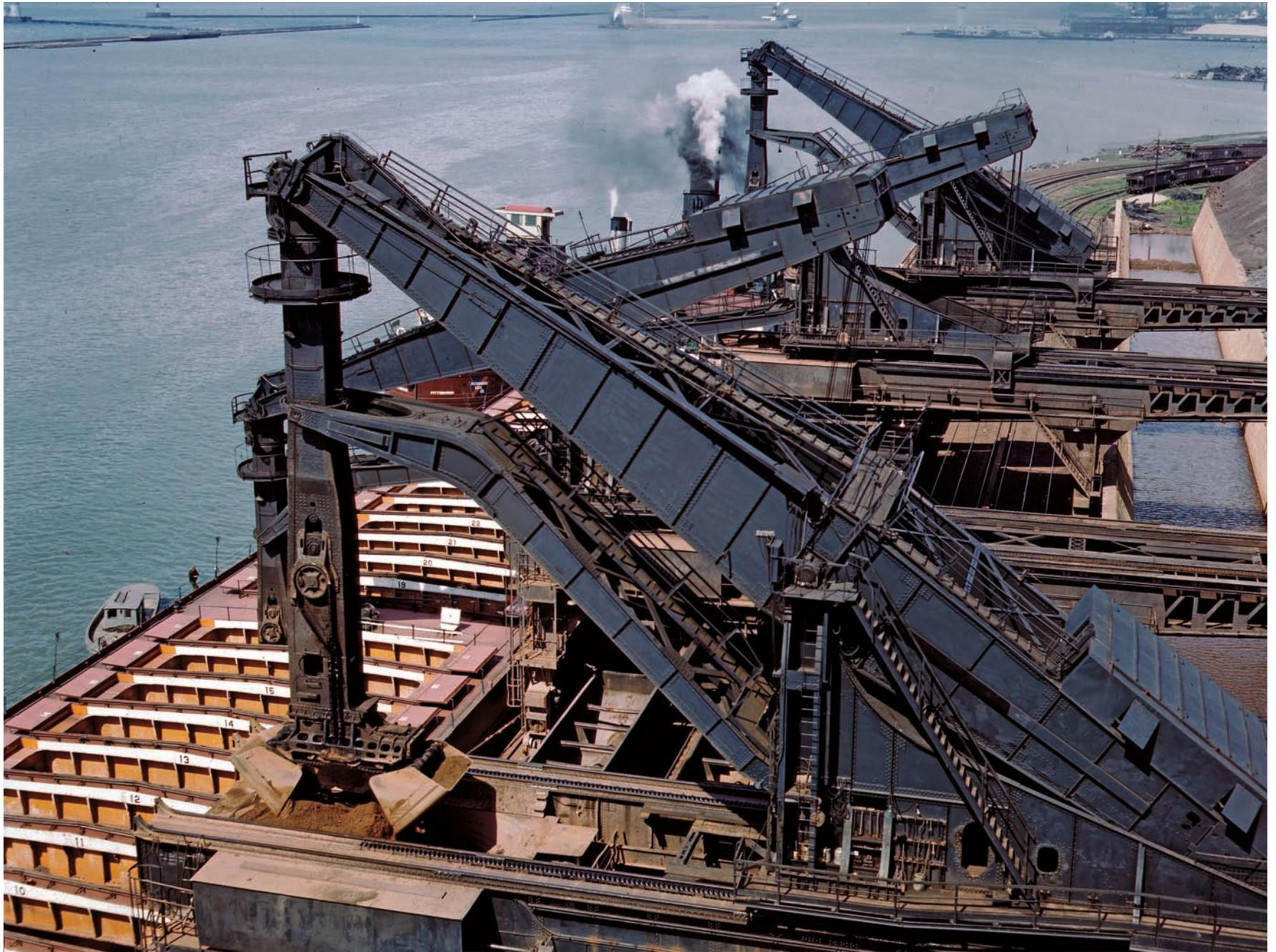
159 Pennsylvania Railroad ore docks, unloading ore from a lake freighter by means of "Hulett" unloaders, Cleveland, Ohio. May 1943.
