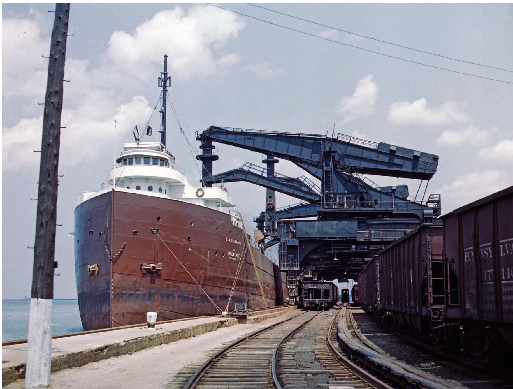
158 Pennsylvania Railroad ore docks, unloading ore from a lake freighter by means of "Hulett" unloaders, Cleveland, Ohio. May 1943.
