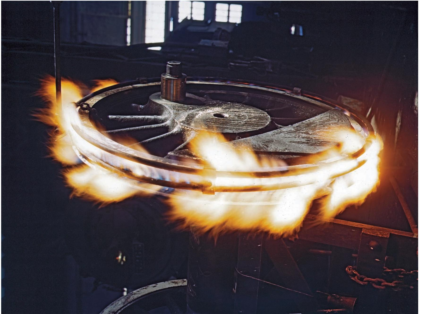
**155** Retiring a locomotive driver wheel in the Atchison, Topeka & Santa Fe Railway locomotive shops, Shopton, near Fort Madison, Iowa. The tire is heated by means of gas until it can be slipped over the wheel. Contraction on cooling will hold it firmly in place. Santa Fe Railroad. March 1943.
