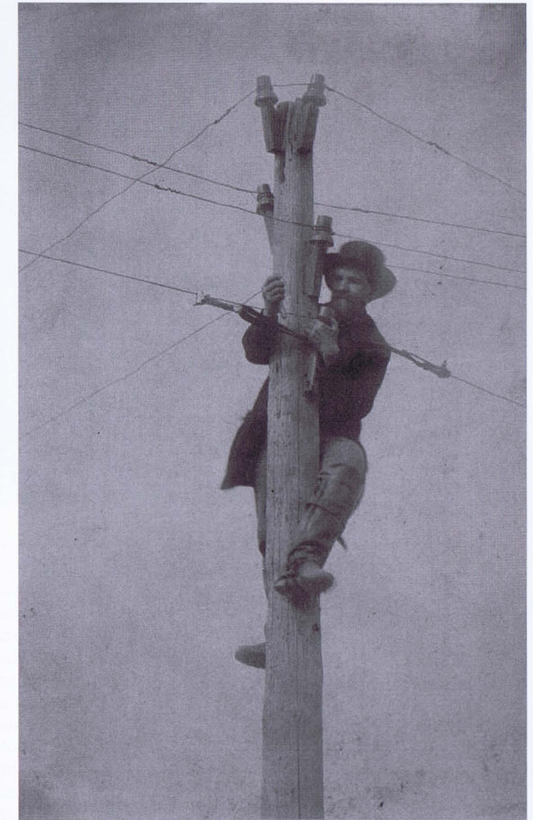
A Union telegraph lineman at work; the job of repairing fallen or cut lines was often dangerous, since if it was attempted within sight of the enemy it attracted sharpshooters. Although the figures are not precise, it is estimated that the telegraph employees working in the field suffered about the same casualty rate as front-line combat soldiers. (LC)
