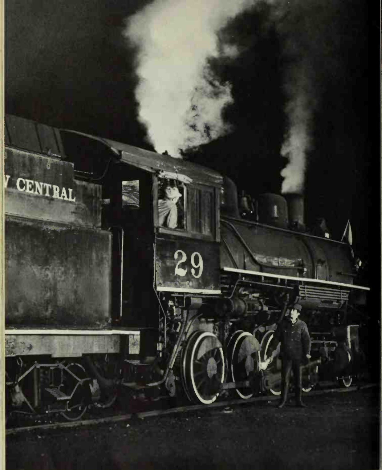
The engineer leans from his side of the cab and talks to the brakeman. The fireman's seat was on the other side. Both watched the track ahead. RON ZIEL
