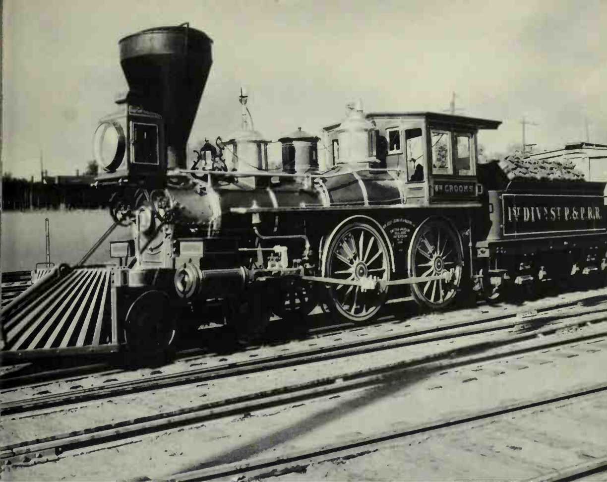
The wedge-shaped cowcatcher attached to the engine pushed wandering animals out of the train's path. P. & P. R. R.
