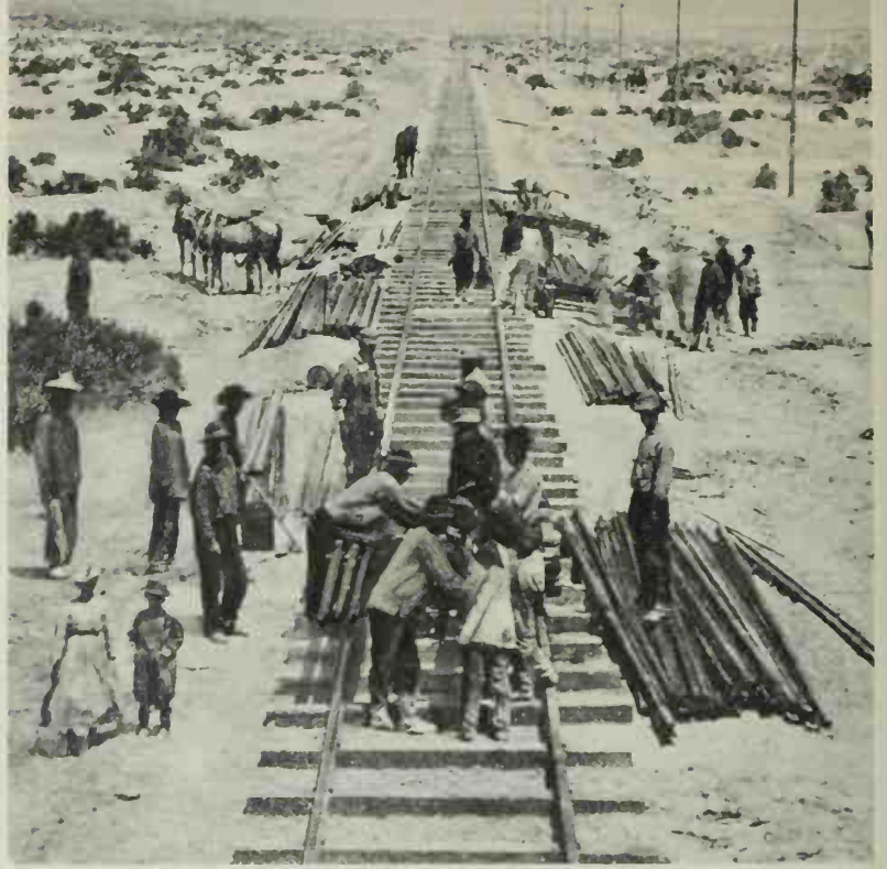
Telegraph lines were strung on poles as the Central Pacific laid its tracks to the East. SOUTHERN PACIFIC
