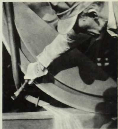
Sand and fuel for modern diesels are stored beside the track. An engineer checks to make sure that an even stream of sand flows in front of the wheels. RAILROAD MAGAZINE
