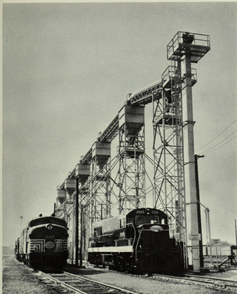
Sand and fuel for modern diesels are stored beside the track. An engineer checks to make sure that an even stream of sand flows in front of the wheels. RAILROAD MAGAZINE
