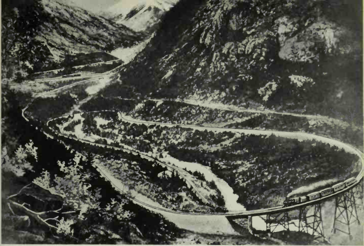
The track of the famous Georgetown Loop in Colorado started in the bottom of a canyon, wound around, climbed the hill, and finally crossed over itself on a bridge.
