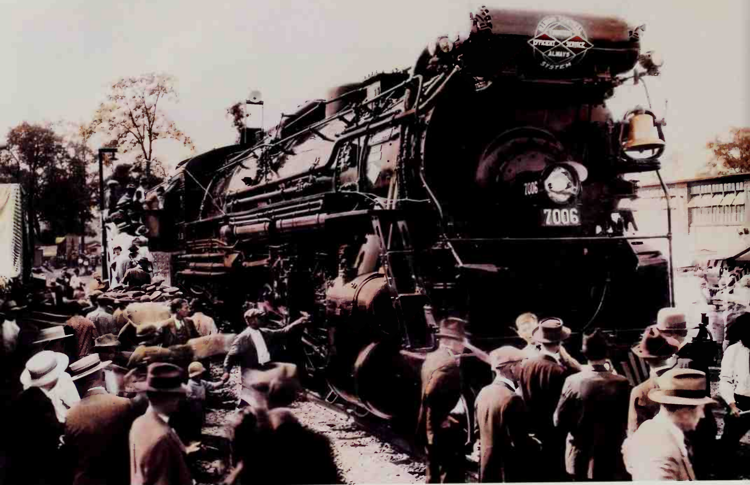
ABOVE. This Chicago exposition featured classic railroad equipment, including this IC 2-8-4 Mountain built by Lima in November of 1926. Large offset brass bell and old red and white IC logo on the overhead feedwater heater makes the locomotive distinctive. Rich Gajnak collection
