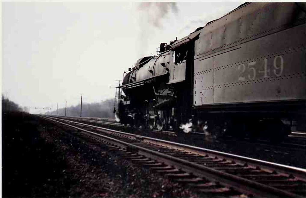
Locomotive #2549 bears down on the high iron in a scene repeated day after day on the IC. This locomotive received its boiler from #2909, rebuilt in 1942. Mountains, such as this unit, were assigned pools and were under the jurisdiction of one single IC shop for maintenance. Jerry Carson
