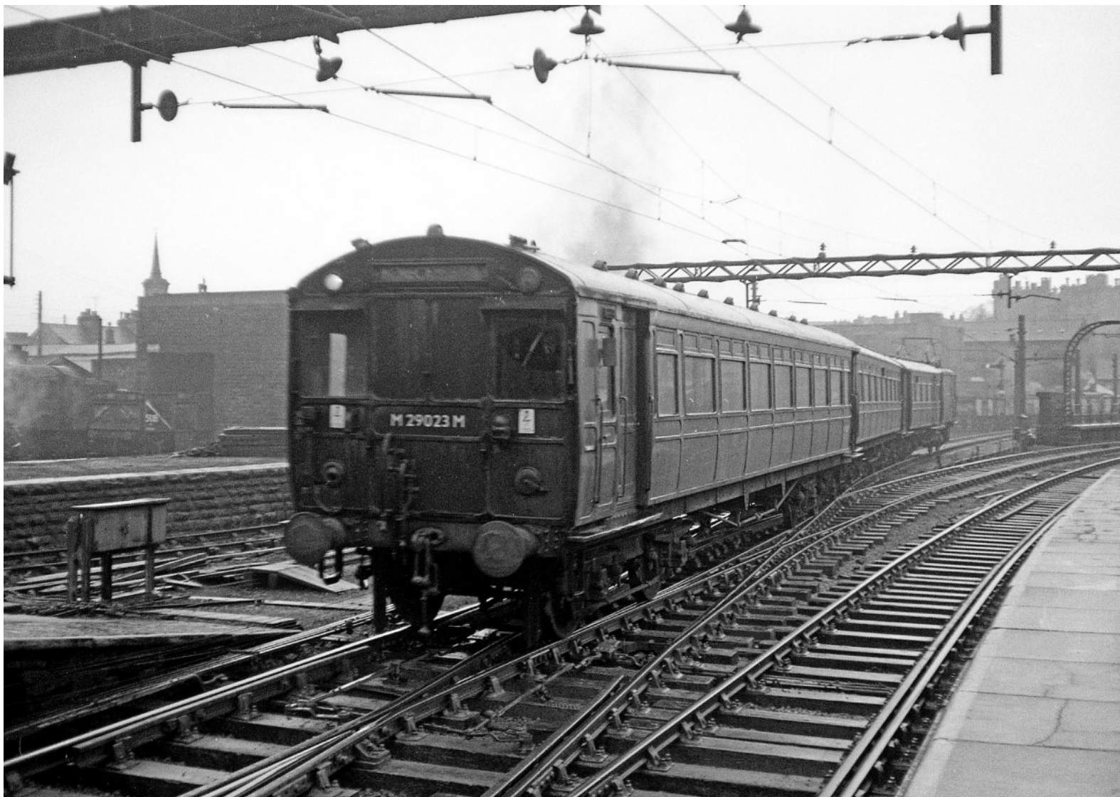
The Midland Railway was a pioneer in electric traction, such as on its route in the North West between Lancaster and Morecambe, which ran alongside the River Lune. In BR days, a fleet of four three-car EMUs (set Nos. 19-22) was created by converting former fourth-rail stock from the London area to overhead supply instead, and these were classified AM1. They survived in traffic until April 16, 1966 when the line was closed and all services to Morecambe concentrated on the former LNWR route via Bare Lane, which is still open today. Pictured on that final day is set No. 21 (with Driver Trailer Standard Open No. M29023M leading), arriving at Lancaster Green Ayre from Lancaster Castle.
