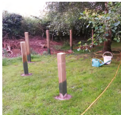
In readiness to start; the bags of 'Postcrete' are located close to the site.
