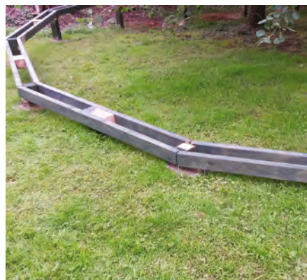
All the inner cheeks on; inner faces were painted and outer support blocks screwed on.
