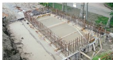
Above: The west end of Corwen Central platform 2 as complete with rear wall and space awaiting infill. GEORGE JONES/LR
