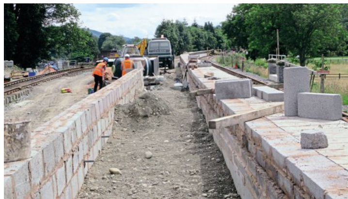
Above: The west end of Corwen Central platform 2 as complete with rear wall and space awaiting infill. GEORGE JONES/LR
