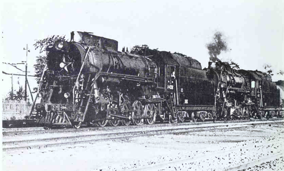
71. Two L class oil-burning 2-10-0s on heavy freight train
