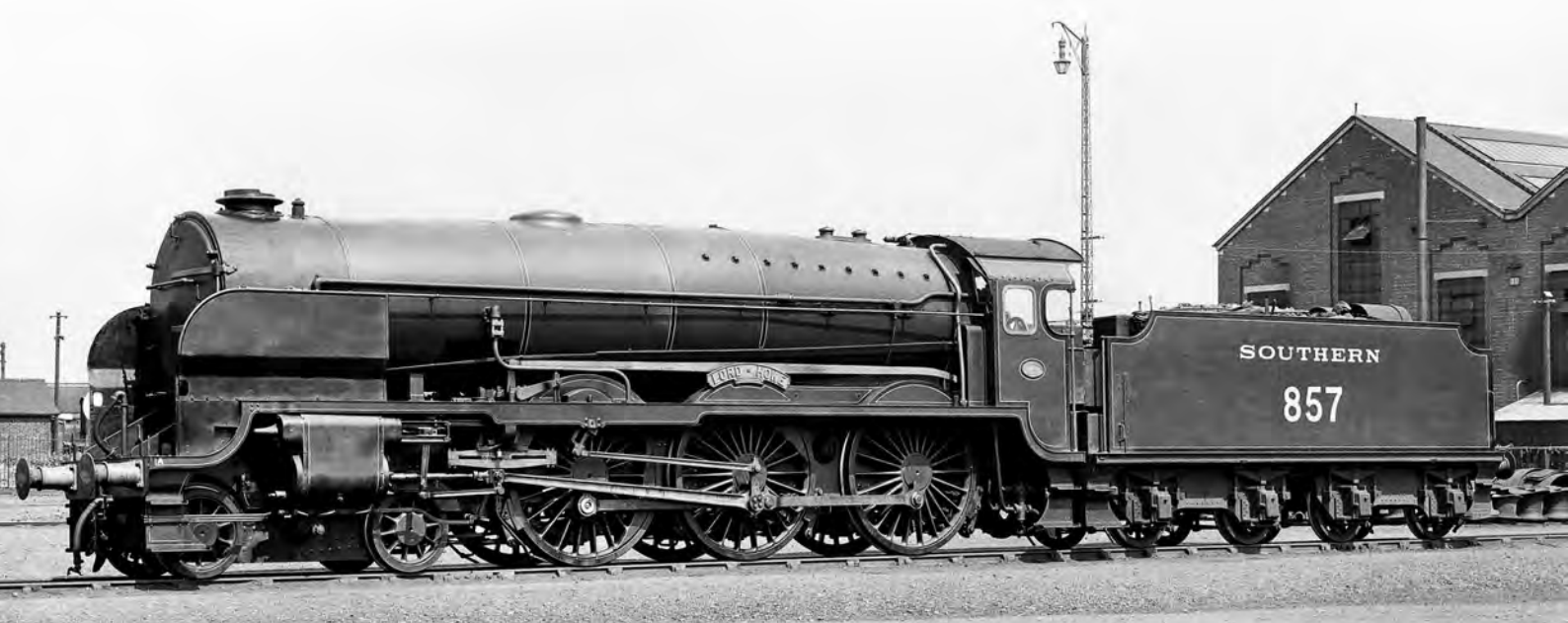
'Lord Nelson' class No 857 Lord Howe is seen outside Eastleigh Works in June 1937, a few months after being fitted with its experimental taper boiler. On account of the increased smokebox diameter, the smoke deflector plates now had to be 'cranked' accordingly. O.J. Morris/Rail Archive Stephenson
