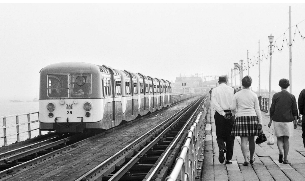
Seen from the wooden walkway of Southend Pier, cream and green-liveried electric-powered pier train No 28 makes its way along the longest pleasure pier in England. The stock illustrated was introduced in 1949, was designed to look like the then current London Transport trains and was built by AC Cars of Thames Ditton in Surrey. The new stock comprised four trains of seven cars, and each train could carry up to 260 passengers. At a top speed of 18mph, the journey took four minutes each way, and during peak periods a train ran every five minutes, continuing until 11pm. The record for passengers carried in one day stands at 55,000.
