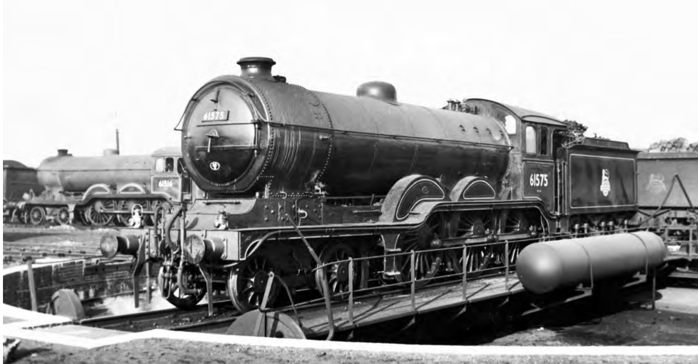
The purchase of a 70ft vacuum-operated turntable for Southend Victoria shed from Cowans Sheldon was authorized in October 1934, and it was installed on built-up ground between the coaling plant and water softening plant. On 11 March 1956 'B12/3' class 4-6-0 No 61575 of Cambridge shed is in the process of being turned, and in the background is another member of the class, No 61516. No 61575 was built by Beyer, Peacock and entered traffic in September 1928 as LNER No 8575; its withdrawal came in April 1959 from Cambridge shed. P.J. Lynch/Kidderminster Railway Museum
