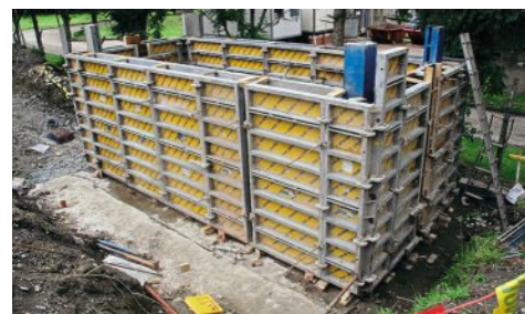
Right: The base for the Corwen Central signalbox rapidly taking shape.
