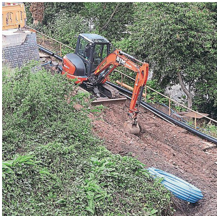
Work to install services along Donkey Gallop to the new refreshment room under construction on Bridgnorth Station's platform 1. SVR
