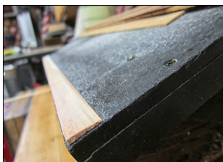
7. The first (bottom) row is a solid \frac{1}{2} " strip, thinned on one edge to a taper.
