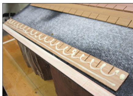
8. Glue is carefully applied to the back of the shingle strip.
