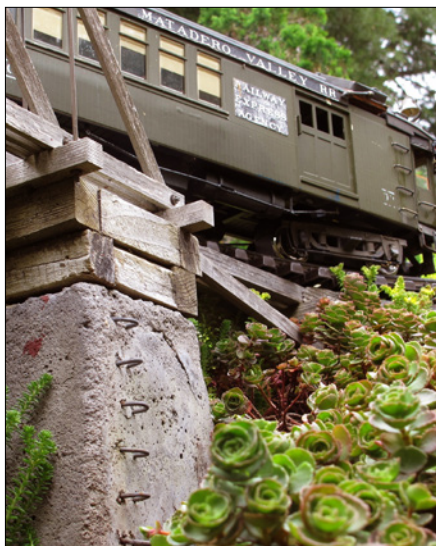
8. A few hours after pouring your abutments, while the concrete is still in the green stage, remove the molds and carefully hammer in some wire staples. These 10-year-old piers on Roger Samuelsen's Golden Bear Railroad have zinc-plated gate staples for rungs. Square-head Romex staples will also work.
