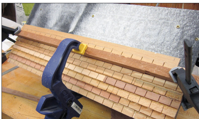
11. The process is repeated, each new strip being clamped in place until it has set. The saw cuts between the shingles were offset on each layer.
