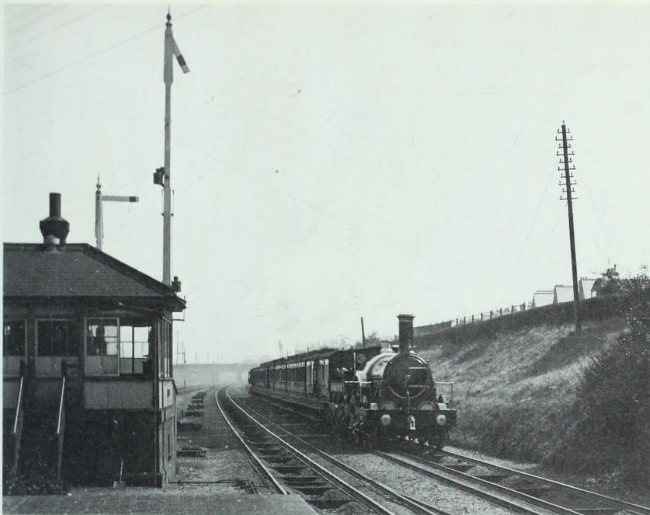
The Flying Dutchman in the last days of the broad gauge passing Ealing. Note 'mixed gauge' track, and early form of tall signal, with arm working in a slot in the post.
