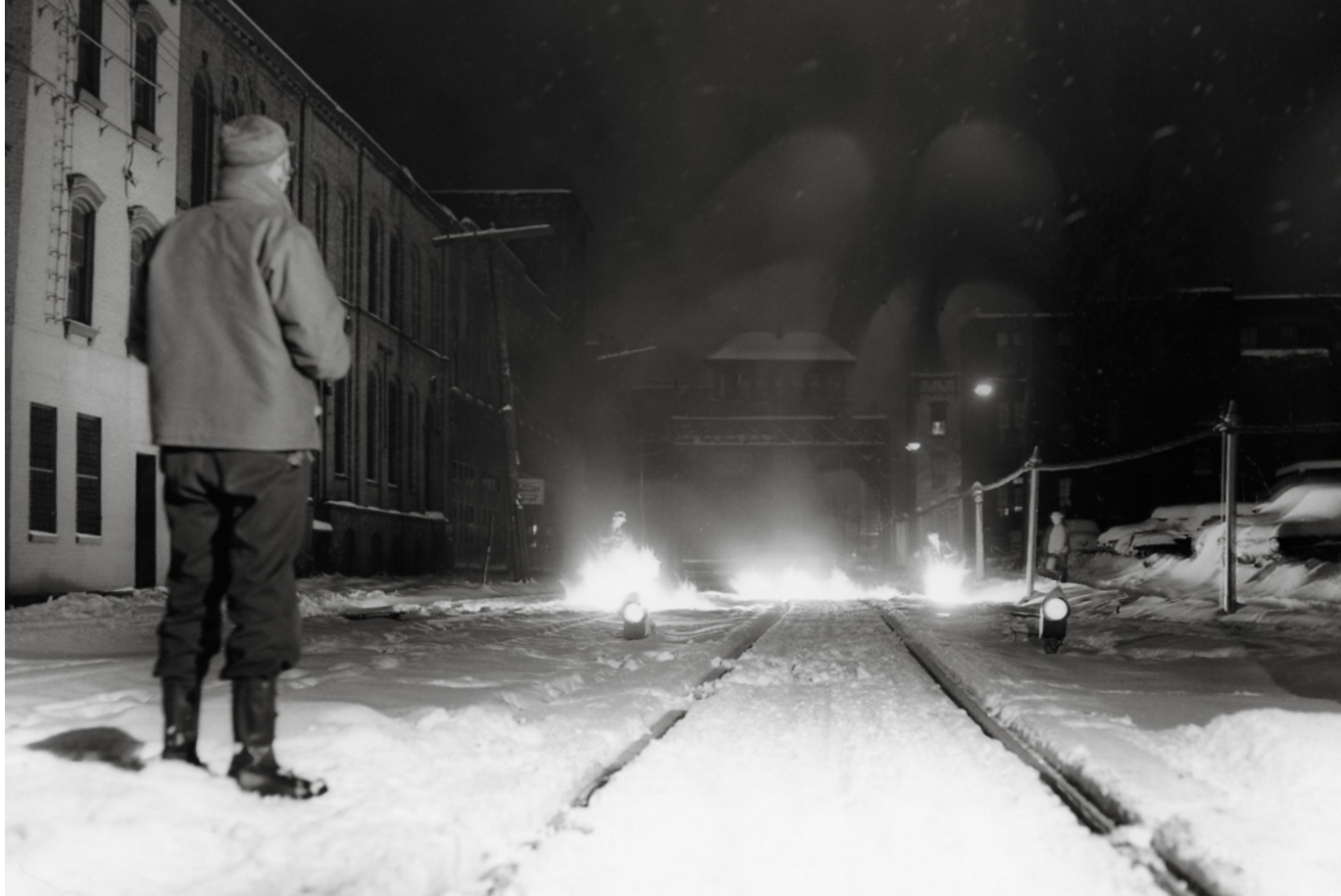
On a night when most parents would rather stay at home, my father drove me through a heavy storm so I could photograph the snow-clearing operations at Troy Union Station. Here he watches a track gang “burn out” the switches at one end of the station complex.
