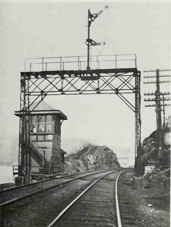
Interlocking signals and tower. (Courtesy of New York Central System, collection of the author)
