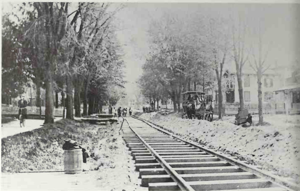
Laying trolley tracks, ca. 1908. (Photo collection of the Huntington, New York, Historical Society)
