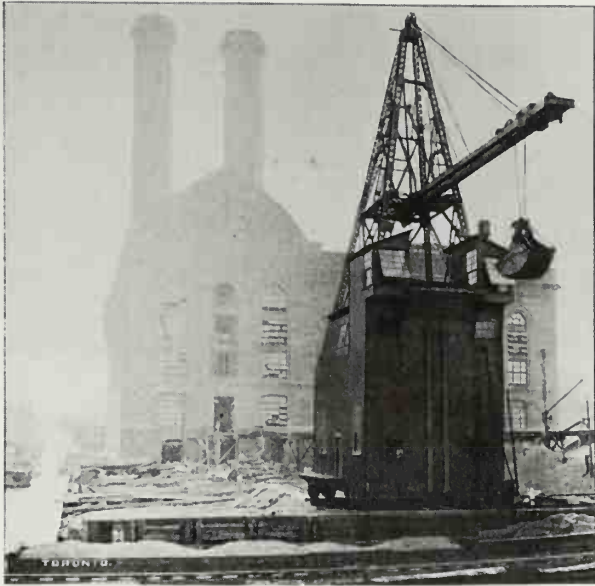
Central station coal-handling equipment with clamshell cranes. (Collection of the author)
