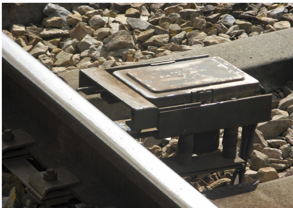
A mechanical treadle switch surviving in traffic on Adelaide's Port line between Bowden and Croydon may well end the reign of these devices, when current works lowering the adjacent station, and the associated upgrading of signalling systems, are complete. Graham Vincent
