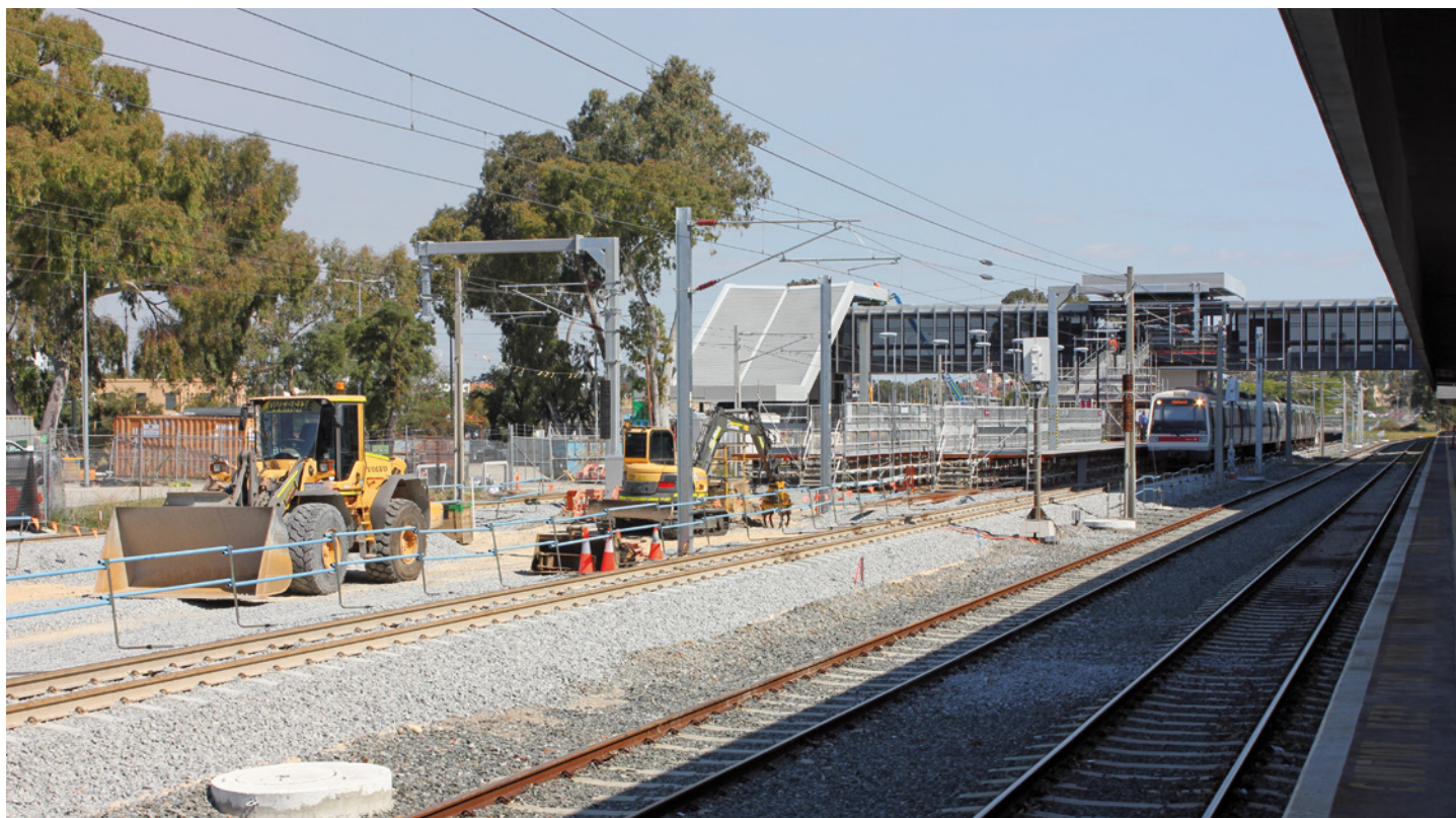
East Perth station on Wednesday 4 October showing the temporary platform extension at the Down end and the new overhead walkway where lifts are being installed. Much of the original platform, and a temporary extension at the Up end, was removed from 22 - 25 September, along with the footbridge. Temporary ramps for access to the platforms now link into the overhead walkway. Down signal 153, which was moved due to the platform extension, is visible. (See report on page 49.) David Whiteford
