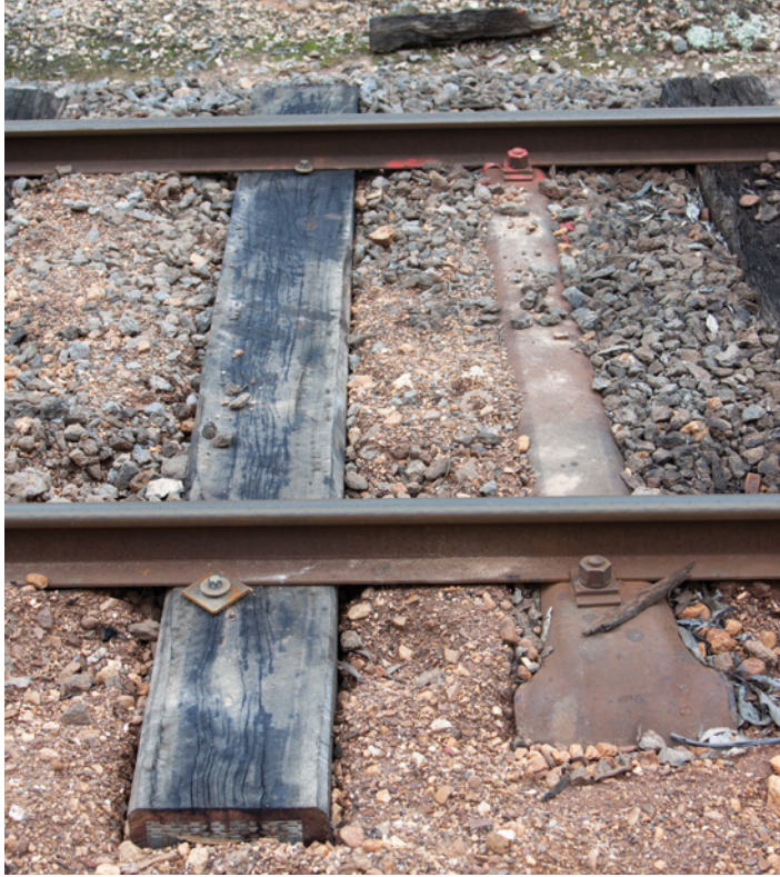
A steel sleeper interspersed with timber. Note the gang nail across the end of the timber sleeper to try and prevent cracking and splits. Adrian Ponton
