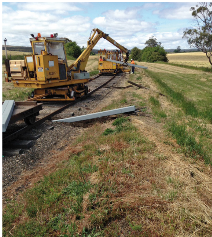
Traditional mechanical insertion methods in use. Insertion by hi-rail excavator with grab clamp also proved successful. Russell Trevaskis
