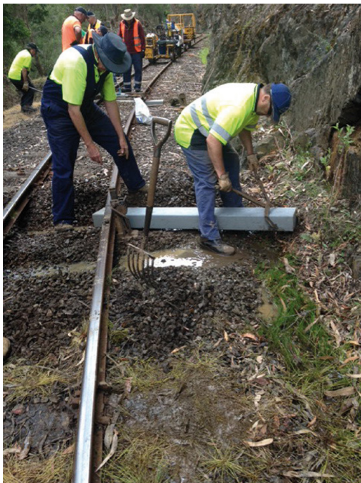
Plastic sleepers being inserted manually in the same manner as for timber sleepers. Russell Trevaskis
