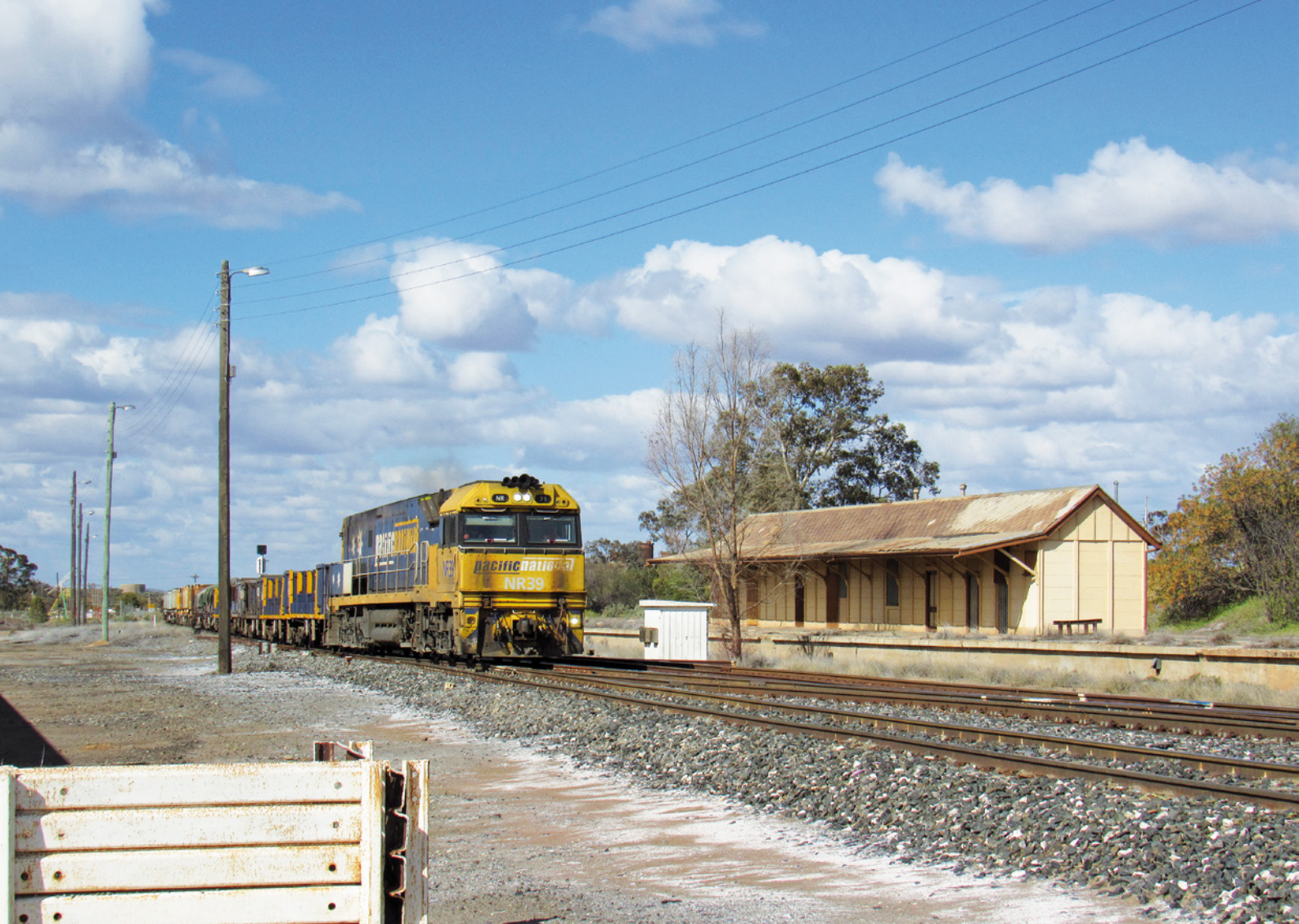
NR39 passes the old Crystal Street Station at Broken Hill with NY3 Newcastle–Whyalla steel train on Tuesday 4 October 2016. The station is a good example of pre-cast concrete slab construction once used in New South Wales and Queensland for railway buildings. Larry Zanker
