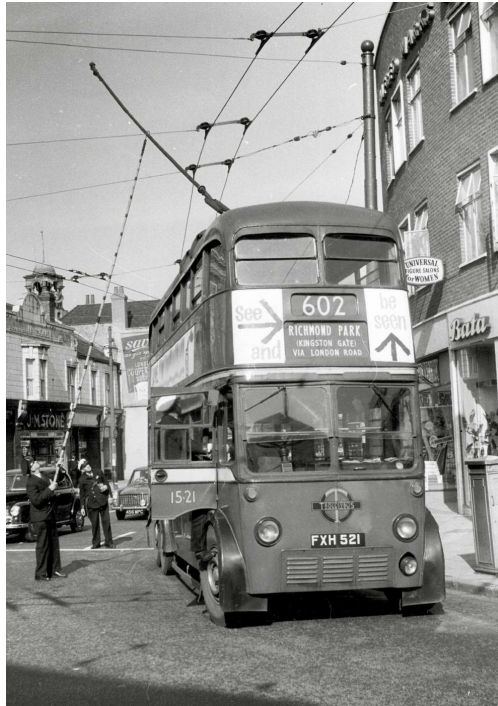
Trolleybus 1521 made the final passenger journey for London Transport on the night of 5/6 May 1962. A few days earlier it demonstrated one of the common problems with trolleybuses: dewirement at a busy road junction. Here an inspector is using the bamboo pole kept underneath the bus to push the booms back on the wires. More than fifty years later 1521 is still running at the East Anglian Transport Museum.
