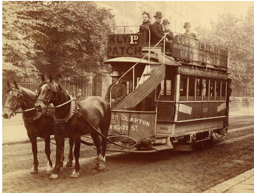
A typical North Metropolitan horsecar in Hackney, north London c.1888. It has its original back-to-back 'knifeboard' seating on the upper deck.
