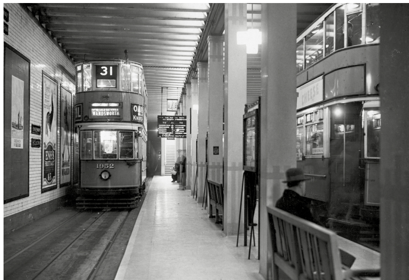
The Kingsway Subway in London was enlarged to take double-deck trams in 1931. This is the underground tram station at Holborn. The subway closed in 1952 but most of it survives almost intact and the northern ramp in Southampton Row still has conduit tram track in place.
