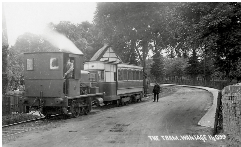
The Wantage Tramway was more like a light railway than a tramway, running alongside a road in rural Berkshire. It was the first tramway to use steam power in 1876, but later used a variety of second-hand rolling stock, as shown in this view c.1914.
