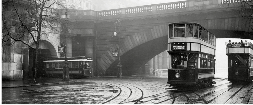
The Kingsway Subway linked the London County Council's northern and southern electric networks from 1908. This is the subway entrance below Waterloo Bridge on the Embankment, showing the unique LCC conduit system with a central slot rail, chosen to avoid using unsightly overhead power lines.
