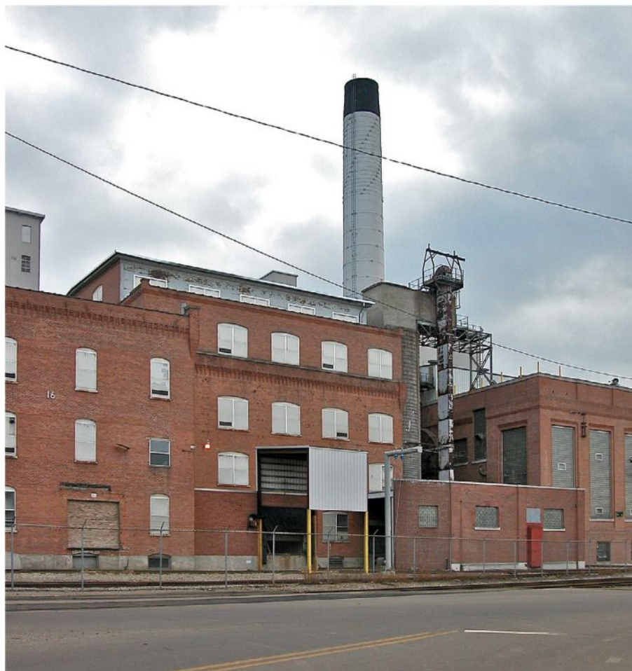
This is the north side of 16 Building (center) and the corner of 16A at left, with spot 9 boarded over; spot 9½ is out of sight to the left. At right-center is covered spot 19½ for unloading coal for the powerhouse. Between 6 Building (right) and 16 is a coal storage silo and tall stack. The track in the foreground leads to spots on the north side 17 and 18 Buildings. Stan Sienicki photo
