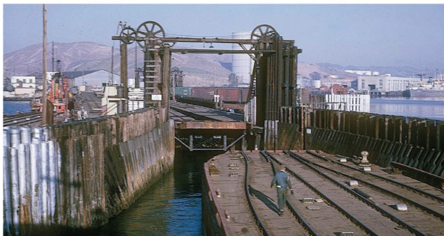
Although taken at Ferry Point in 1962, this photo shows the same kind of apron hoist used at Alice Street, and the three tracks on the car float squeezing together to meet the closely spaced tracks on the apron. Jack Whitmeyer photo
