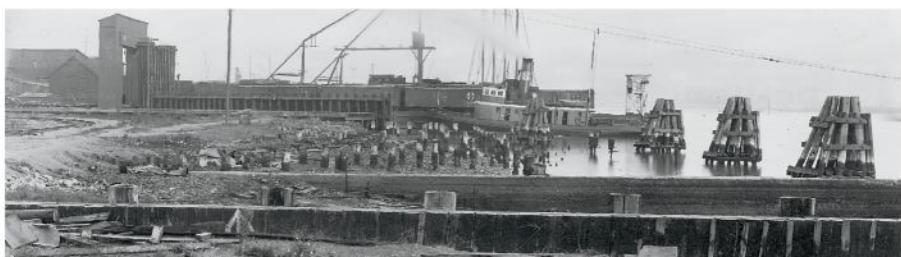
Looking south along the Oakland waterfront, car float No. 3 is tied up at the Alice Street slip along with the Santa Fe tug Richmond . The tall structure to the left is the hoist house that adjusted the ferry apron's height. Vernon Sappers collection photo
