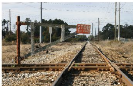
This smashboard crossing gate at a CSX-Norfolk Southern diamond at Dock Junction in Brunswick, Ga., photographed in February 2010, could serve as a prototype for an interesting, possibly operating, trackside detail at a dummy crossing.
