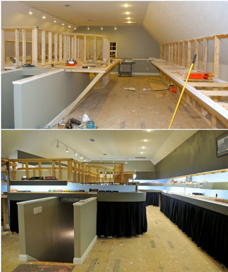
6. An under-construction photo (top) shows the 6-foot-high knee walls and the helix above the stairwell. The same view (bottom) at a later stage of construction shows the fascia, valance, and skirting.
