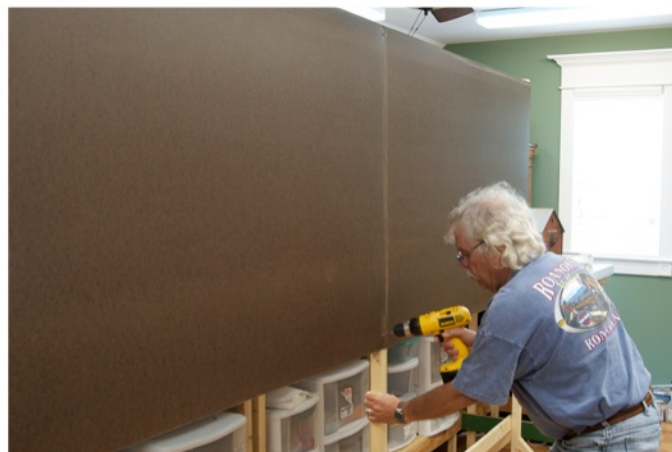
Lou erected a self-supporting framework for the backdrop that fits between the two halves and attached a laminate of \frac{1}{8} " tempered hardboard and \frac{1}{8} " PVC panels to both sides. Nothing is attached to the room walls.
