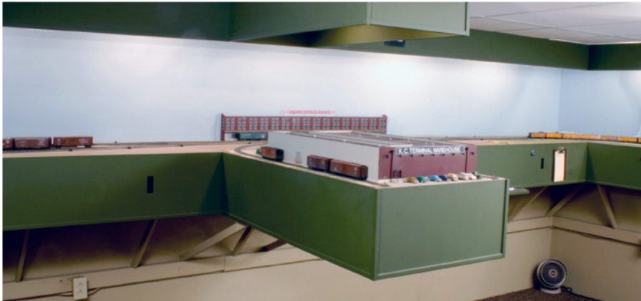
The KC Terminal Warehouse on Chuck's railroad extends 4 feet into the aisle, which required sturdier cantilevered bracing than the 3-foot peninsula.
