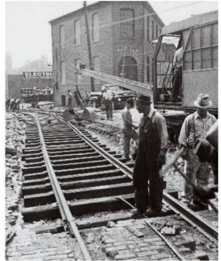
The Tar Branch included some stretches of street running. In this 1967 photo, crews are repairing tracks laid in Wachovia Street, three blocks from the WSS freight house. The triangular building in the background is the Fries Power Co. substation. Photo courtesy of Forsyth County Public Library photograph collection, Winston-Salem, N.C.
