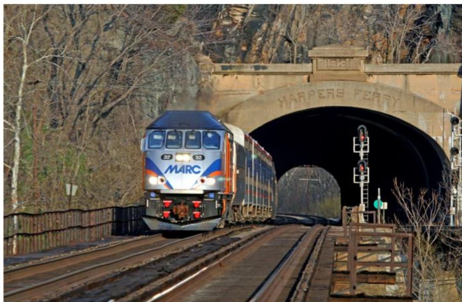
MARC 32, a westbound evening commuter train from Washington, D.C., crosses the Harpers Ferry Bridge on April 4, 2011. Four MARC trains and Amtrak’s Capitol Limited will pass by during the week between 5 and 7 p.m. The bridge’s hump is the result of projects to improve clearance by lowering the tunnel floor.
