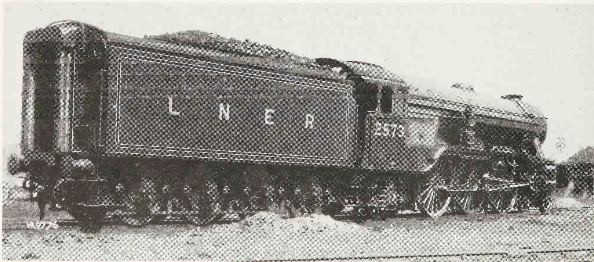
View from rear of No 2573 showing the corridor tender connection
