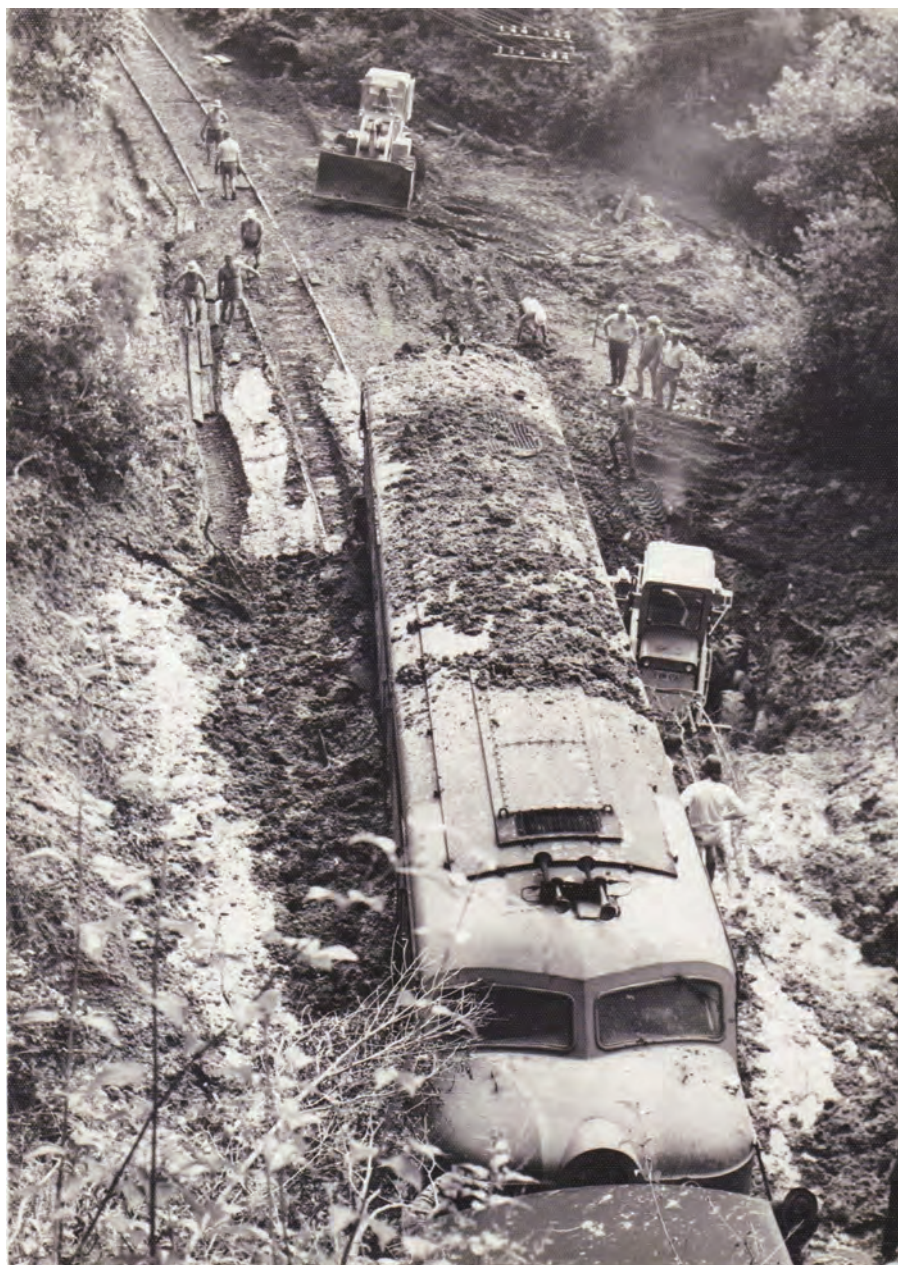
Looking down on the stranded locomotive 4450 after the clean-up had commenced. By this stage, most of the mud from the landslide had been cleared away and re-railing of the locomotive was about to commence. COURTESY THE LATE CEC COX
