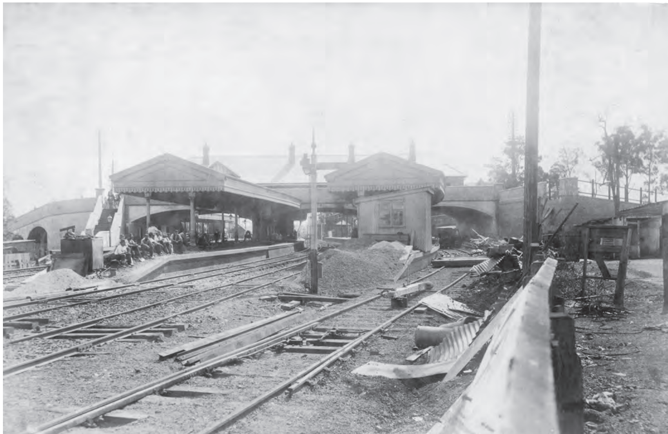
The reconstruction of Strathfield Station being undertaken circa 1900. The use of reinforced concrete for the overhead bridge on this project was a pioneer use of this technology, but in this instance it was not successful. ARHSNSW RAILWAY RESOURCE CENTRE, 113525
