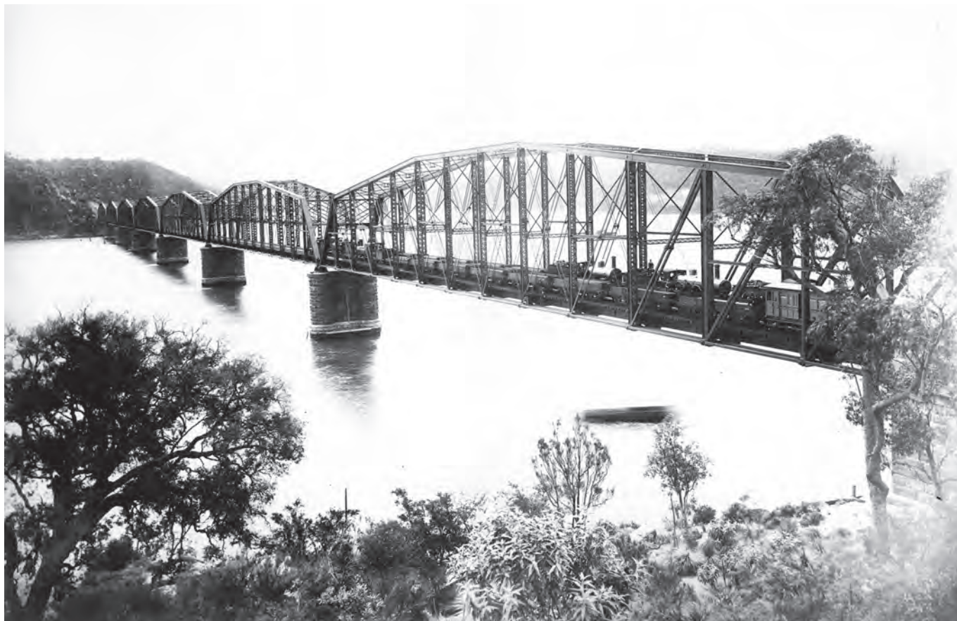
Testing the Hawkesbury River Railway Bridge with locomotives and wagons, 20 April 1889. NSW GOVERNMENT RAILWAYS PHOTO, ARHSNSW RAILWAY RESOURCE CENTRE, 038844.
