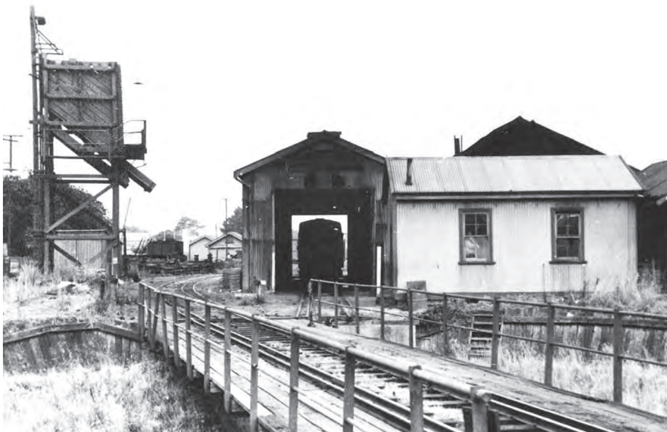
The old Mount Gambier Locomotive Depot from the western end, with the 75 foot turntable in the foreground and the 15-ton coaling stage on the left. NATIONAL RAILWAY MUSEUM PHOTO
