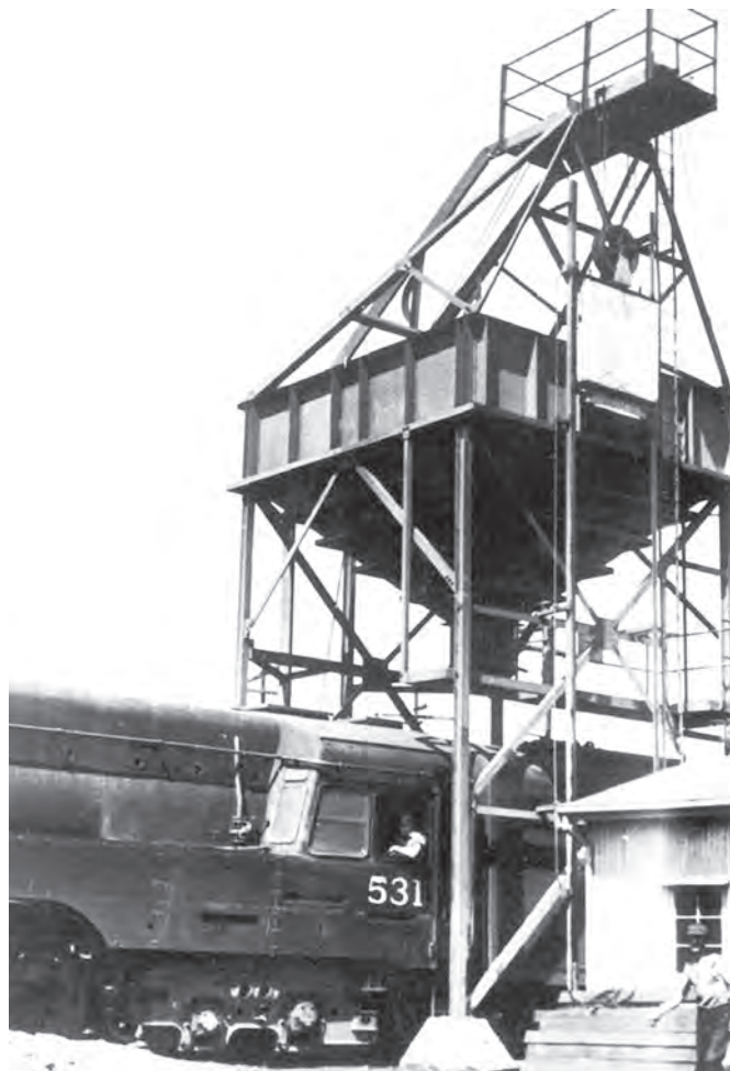
SAR 520 Class 4-8-4 locomotive 531 being coaled at the 45-ton coaling plant at Naracoorte in the 1950s. NATIONAL RAILWAY MUSEUM PHOTO
