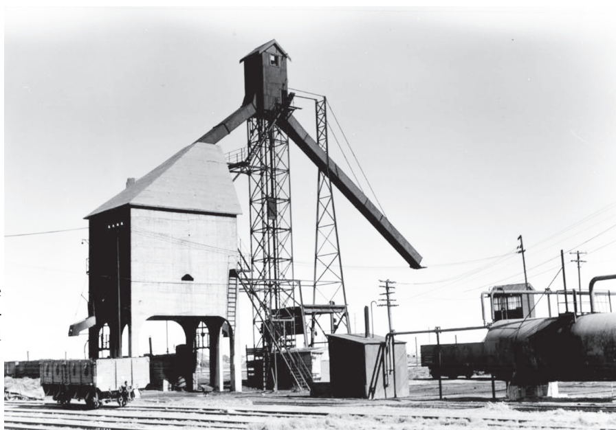
The 500-ton coal plant at Port Pirie loco depot in June 1952. The area beneath the chute to the right was an open coal floor, but coal was in short supply at Port Pirie in the 1950s, so many steam locomotives at the depot were oil-burners—narrow gauge and broad gauge. Standard gauge locomotives were rare visitors to Port Pirie. DOUG COLQUHOUN PHOTO
