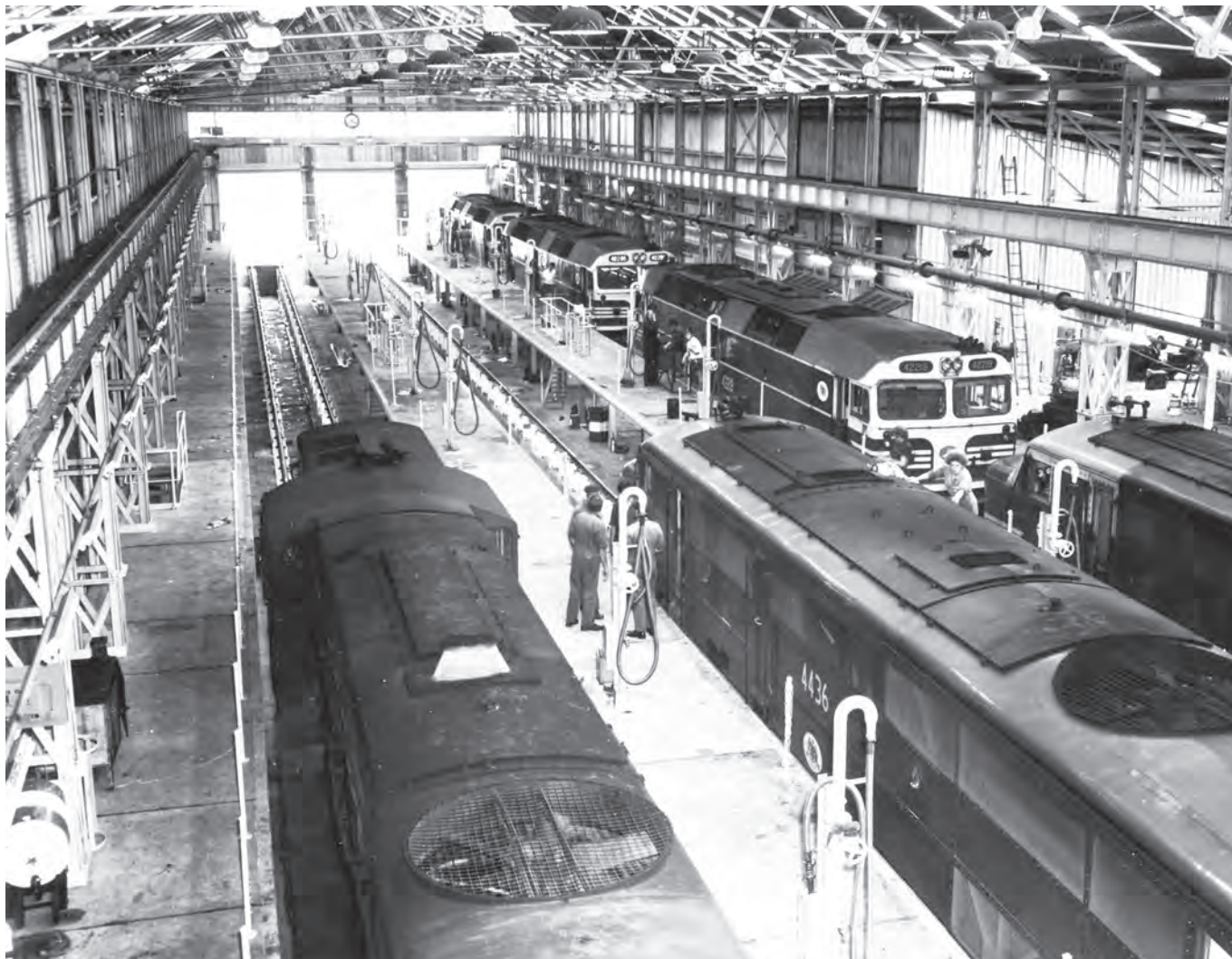
Overview of the service area at DELEC with a 45 and 4436 on the two through casual inspection roads not scheduled for regular maintenance. The locomotives on the third row are receiving more intensive scheduled inspection and maintenance in this March 1971 photo. NSWGR PHOTO, ARHSNSW RAILWAY RESOURCE CENTRE, 022288
