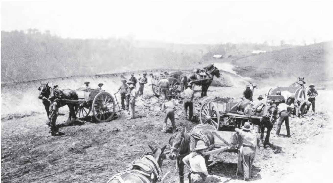
Construction workers preparing the trackbed at Megan on the Glenreagh to Dorrigo Line circa 1915.
