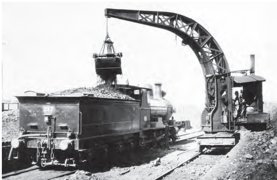
SAR Rx Class locomotive No. 217 being coaled by Cowans Sheldon coaling grab crane (B/No. 2905 of 1908) at Mile End Depot c1925. SAR PHOTO, R HORNE COLLECTION
