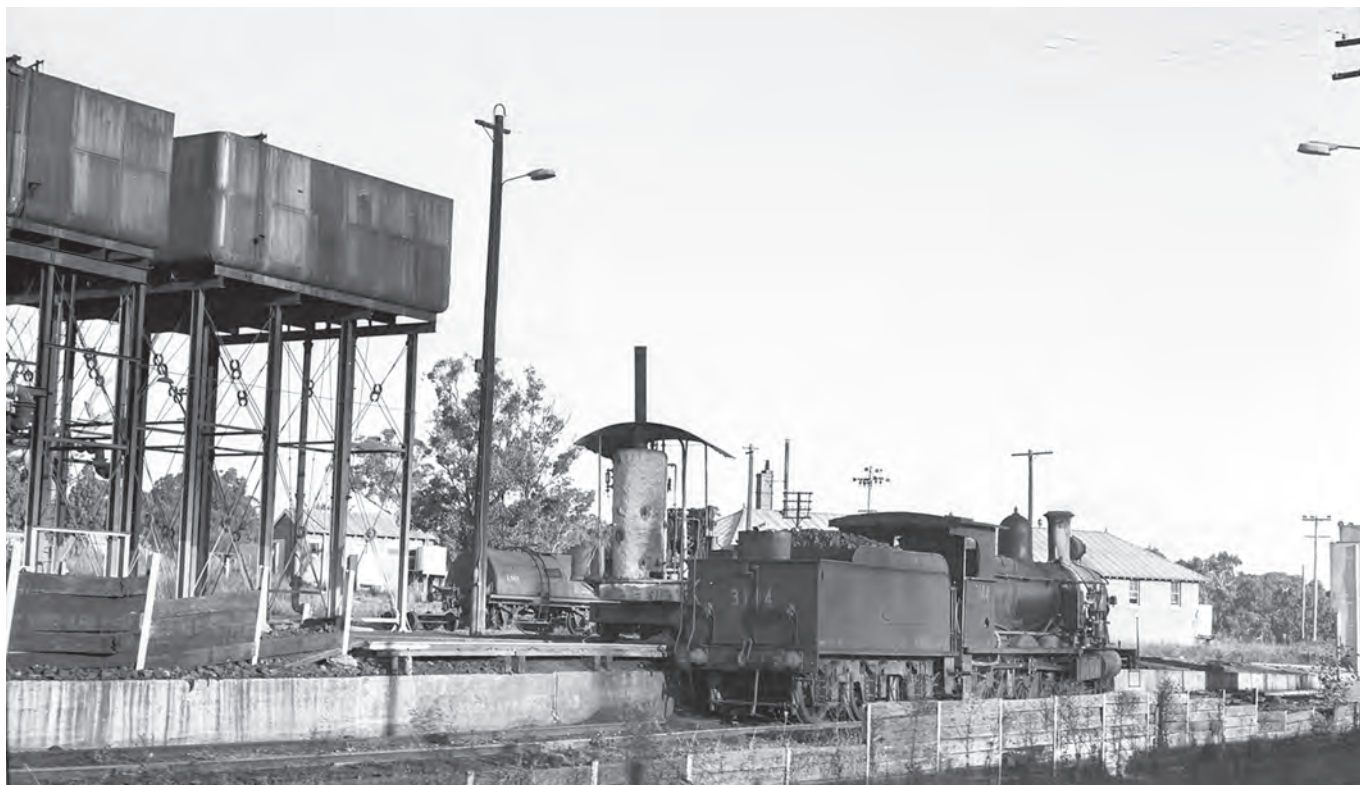
Binnaway locomotive depot on 12 March 1967 with steam grab No. 1057 coaling the 30T Class locomotive 3144. The crew barracks are in the right background. ALEX GRUNBACH PHOTO, ARHSNSW RAILWAY RESOURCE CENTRE, 200961
