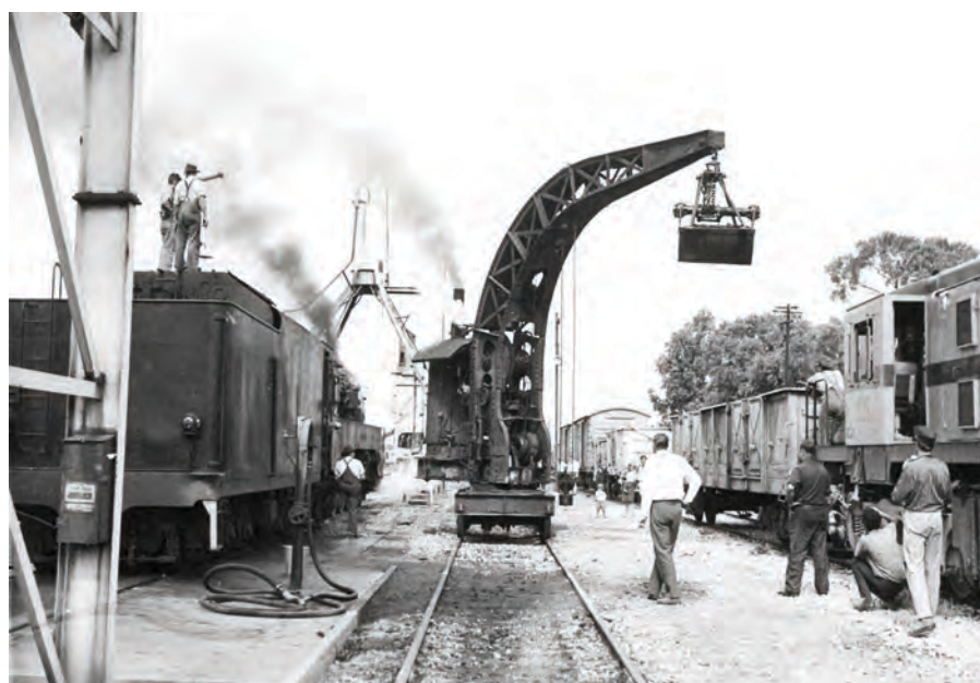
Tour train steam locomotive 520 is coaled at Taillem Bend, as in days of yore, by means of a rail-mounted grab crane, as at the time in the early 1970s the coaling plant was no longer in use. At the larger depots these grab cranes were generally used to muck out ash pits. NATIONAL RAILWAY MUSEUM COLL ALX14461
