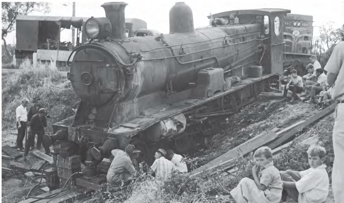
Breakdown gangs use branch line diesel-electric locomotive 4917 to haul locomotive 3378 up the embankment at Coonabarabran for re-railing on 17 November 1965. Locomotive 4917 still operates with the Southern Shorthaul Railroad. G BANFIELD PHOTO, ARHSNSW RAILWAY RESOURCE CENTRE, 503471
