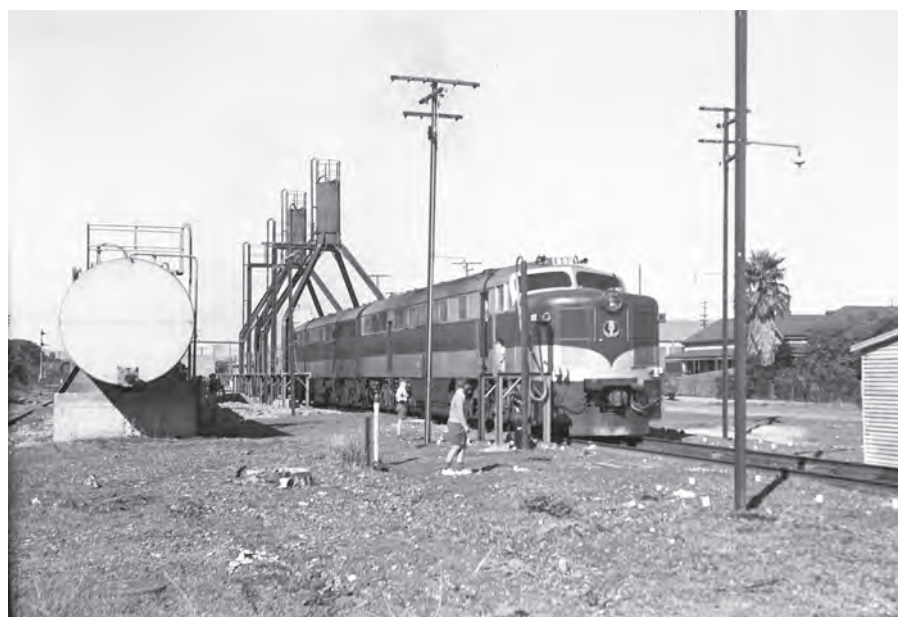
This temporary depot was set up in 1950 to service the new diesel-electric locomotives on a single track immediately adjacent to the Mile End Station. Note the pair of distinctive sanding towers straddling the 900 Class locomotives. WAL JACK COLLECTION, NRM, 01865
