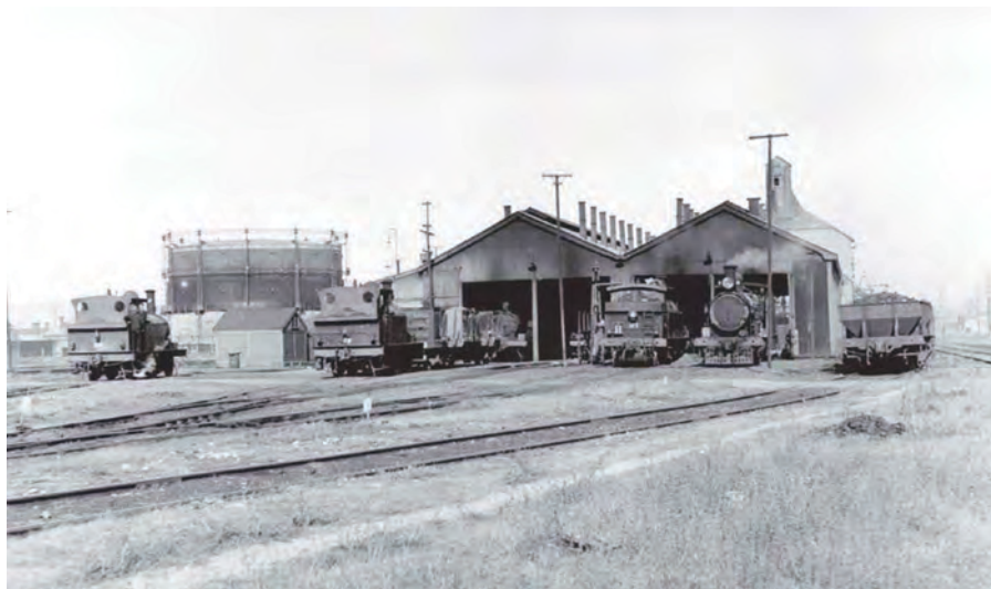
The old straight running sheds at Port Adelaide locomotive depot in 1952 with F, P and Rx Class steam locomotives awaiting their next roster. This running shed comprised a paired gable structure with a lean-to annex on the left. The 150-ton coaling tower dominates the background. DOUG COLOQUHOUN PHOTO
