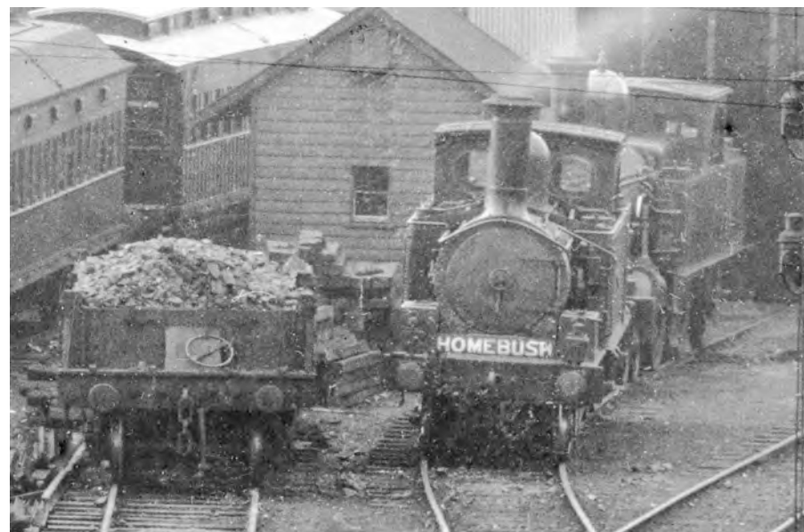
Also from the large c1905 image, an E Class 2-6-4 tank locomotive stands outside the old Sydney engine shed with a 'HOMEBUSH' board and a CC Class 4-4-2 tank locomotive behind. ARHSNSW RAILWAY RESOURCE CENTRE, 432453D
