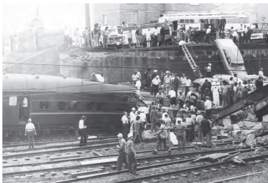
The collapsed Bold Street road overbridge and crushed carriages at Granville following the January 1977 disaster. ARHSNSW RAILWAY RESOURCE CENTRE, 505956
