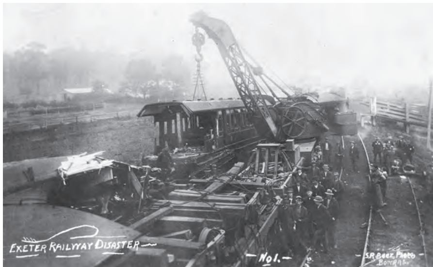
A large breakdown crane lifts a damaged carriage following the head-on collision between the Temora Mail and a goods train at Exeter on 13 March 1914. . S R BEER STUDIO, BOWRAL, ARHSNSW RAILWAY RESOURCE CENTRE, 006903B
