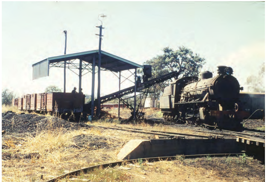
W Class 4-8-2 locomotive No. 943 at Boyup Brook locomotive depot with its coal conveyor and 60ft turntable on 12 January 1968. P HOPPER PHOTO, RAIL HERITAGE WA, P11831
