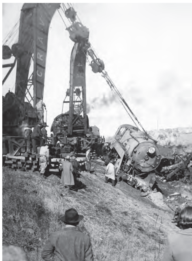
Two heavy Craven breakdown cranes lift locomotive 3817 back onto the track following the mail train derailment at Rocky Ponds on 30 June 1948.
