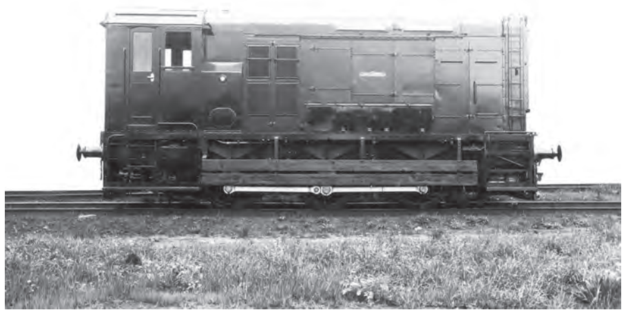
F310, the Victorian Railways class leader of the 0-6-0 diesel-electric shunting locomotives based on a successful Briting design and built by English-Electric entered service in 1951. VR PHOTO, ARHSNSW RAILWAY RESOURCE CENTRE, 243950
