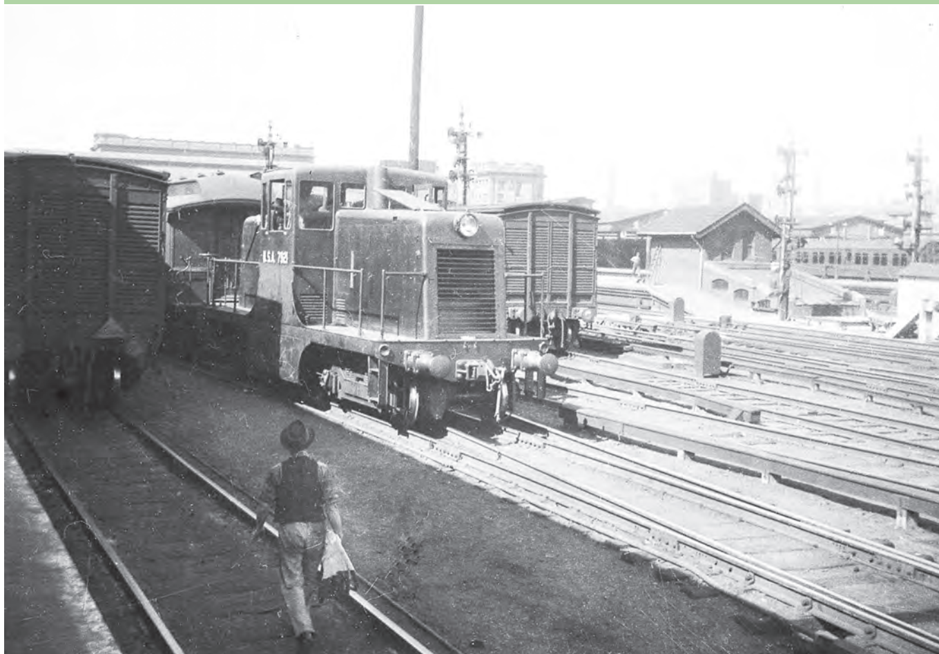
Australia's first diesel-electric locomotives were four former US Army Bo-Bo 380hp (279kW) locomotives imported by the Commonwealth Department of Munitions in 1943. By 1946, 7923 was on shunting duties at Sydney Terminal Station. R B McMILLAN COLLECTION, ARHSNSW RAILWAY RESOURCE CENTRE, 214006
