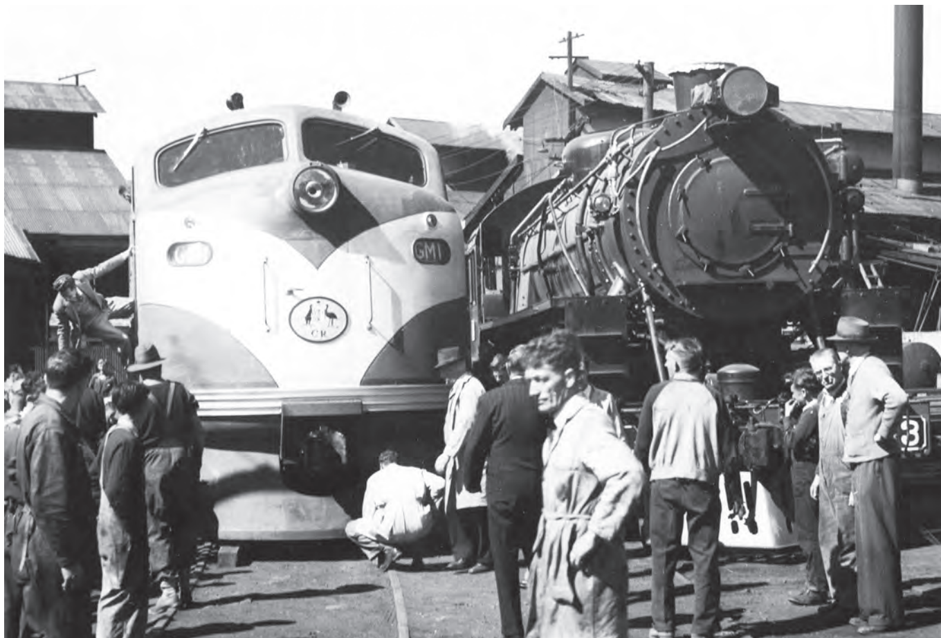
New and old: Commonwealth Railways motive power in the builder's yard of Clyde Engineering at Granville in New South Wales in 1951. GM1, the first Commonwealth Railways mainline diesel to enter service is being checked out on the left, alongside is 2-8-2 L83, one of the final steam locomotives to work on the CR. R J GUTHRIE PHOTO, ARHSNSW RAILWAY RESOURCE CENTRE, 022468
