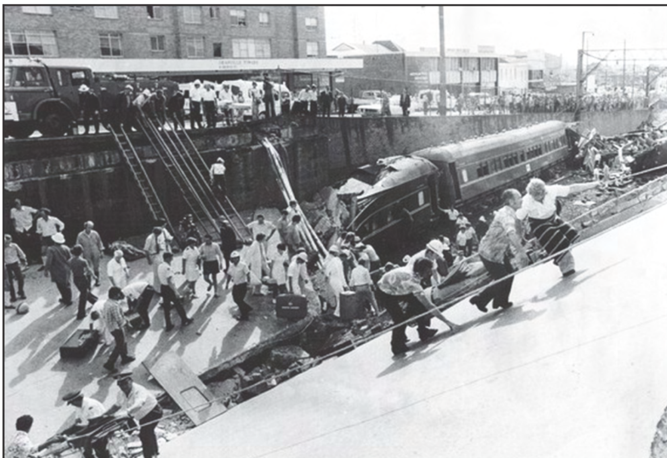
Rescuers setting ropes to lift the Bold Street overbridge from the crushed carriages using MFD hydraulic jacking equipment. BOB O'LOUGHLIN PHOTO
