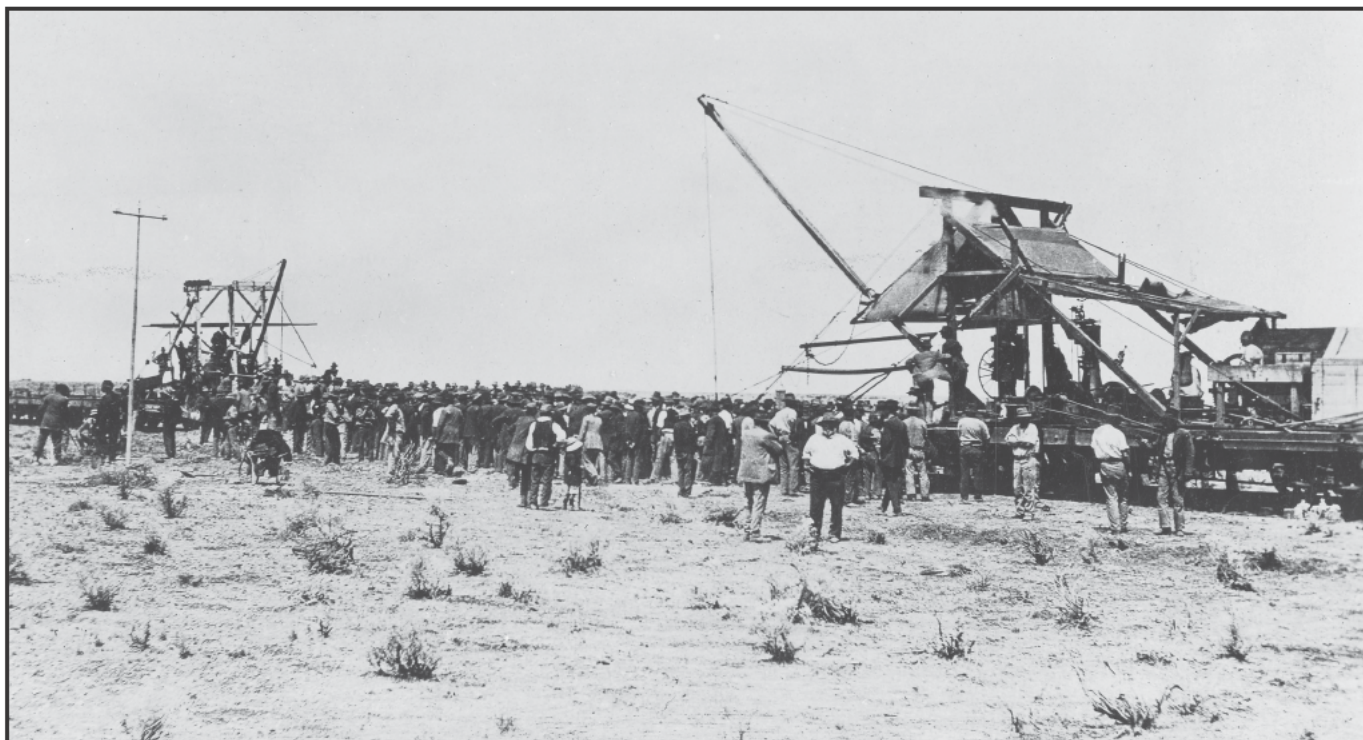
The meeting of the track-laying gangs at Ooldea on 17 October 1917. There were two flat wagons R3 and R20 fitted with these crane assemblies to lay the rails on the manually laid sleepers. Wagon R3 worked westward from Port Augusta while R20 worked eastward from Kalgoorlie. TRANS-AUSTRALIAN RAILWAY POST CARD, ARHSNSW RAILWAY RESOURCE CENTRE, 446627
