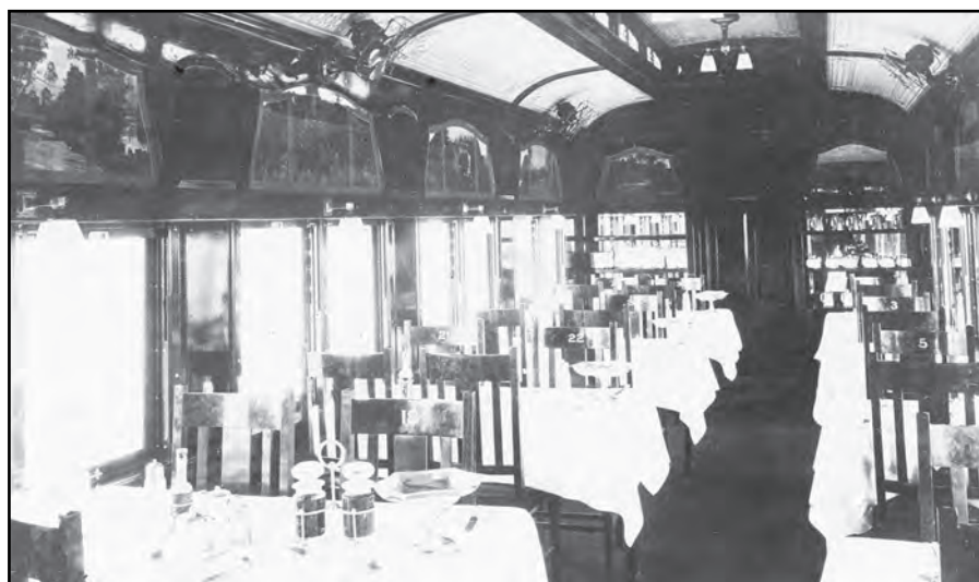
An interior view of a D Class dining car in the condition that it entered service. The two and one across seating provided for only 30 passengers and was insufficient so in 1920 the dining saloon was changed to two and two across providing for 40 diners.
