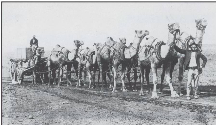
Reliable fresh water was essential for the construction camps in the desert. A team of camels haul a wagon with a loaded water tank during the TAR construction period. TRANS-AUSTRALIAN RAILWAY POST CARD, ARHSNSW RAILWAY RESOURCE CENTRE, 446617
