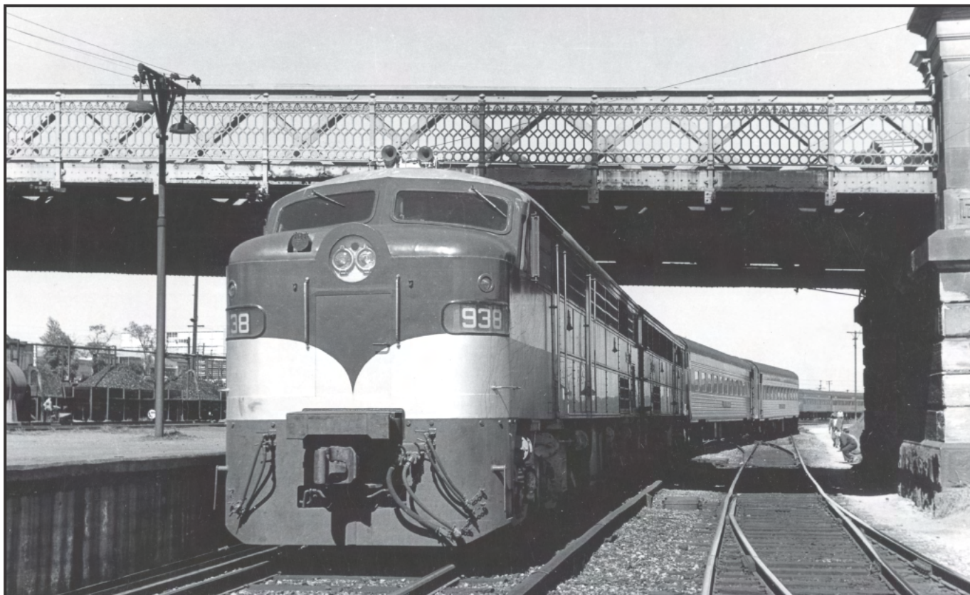
Goodwin-Alco 930 Class diesel-electric locomotive and a sister unit head The Overland train into Adelaide Station in the 1960s. RAILWAY TRANSPORTATION PHOTO, ARHSNSW RAILWAY RESOURCE CENTRE, 024641
