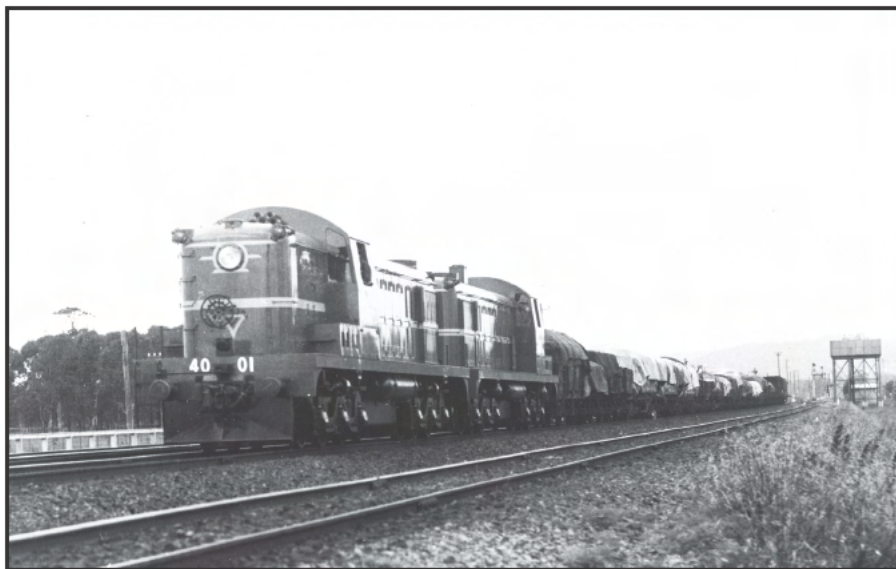
Pioneer 40 Class diesel-electric locomotives 4001 and a sister unit head a Down mixed goods train at Tuggerah in the early 1950s. NSWGR photo, ARHSnsw Railway Resource Centre, 017866
