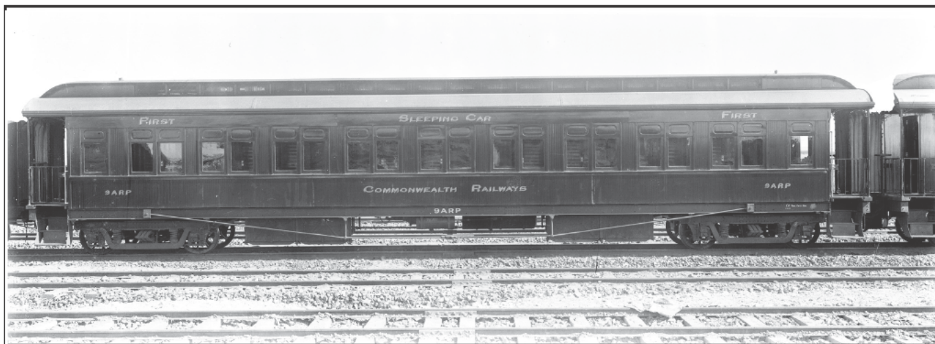
First Class Sleeping Car ARP9 photographed around the time of the opening of the line. The car is in the original red livery which was used until the early 1920s when both the endplatforms were in place. This was not one of the cars that had one endplatform enclosed to enable the installation of showers. In the 1910s passenger cars lettering followed Victorian Railway practice placing the car number in front of the code. PHOTOGRAPH CHRIS DRYMALIK COLLECTION
