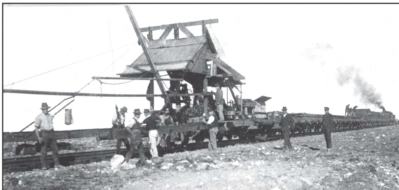
The Roberts tracklayer R20 working from the west advances towards the border from Kalgoorlie on the world's longest straight stretch of railway circa 1916. The wagons are loaded with steel rails and sleepers. COURTESY DAVID BURKE COLLECTION
