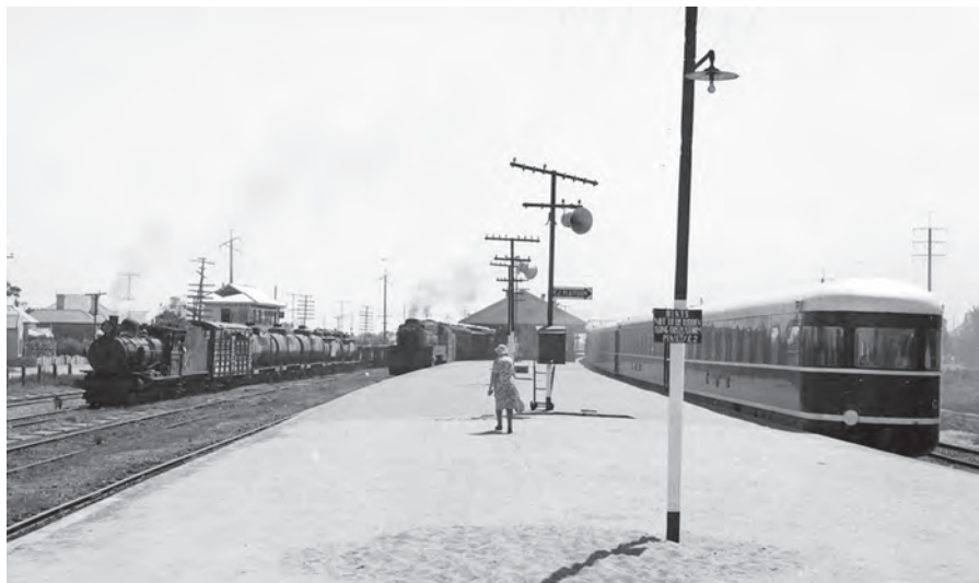
Movement on three gauges at Port Pirie. From the left, a narrow gauge T Class locomotive on a Peterborough-bound freight train, a broad gauge 520 Class 4-8-4 on the Adelaide-bound connection from Perth and to the right, the observation car on the rear of the modern standard gauge Trans Australian Express service. NATIONAL RAILWAY MUSEUM PHOTO, AZ21650.
