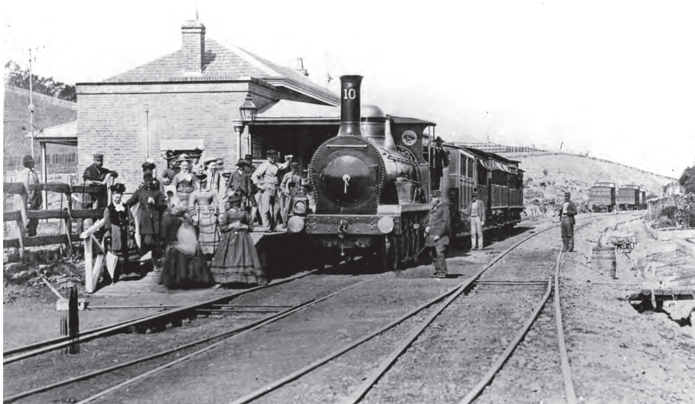
Thomas Firth came to New South Wales as an engineer with the contractors Peto, Brassey & Betts in January 1859 as a manager on their contract to extend the Great Southern Railway from Liverpool to Picton. Here 2-4-0 tender locomotive No. 10, built by the NSW Railways workshops in June 1870, stands at Picton Station with a passenger train circa 1874.
