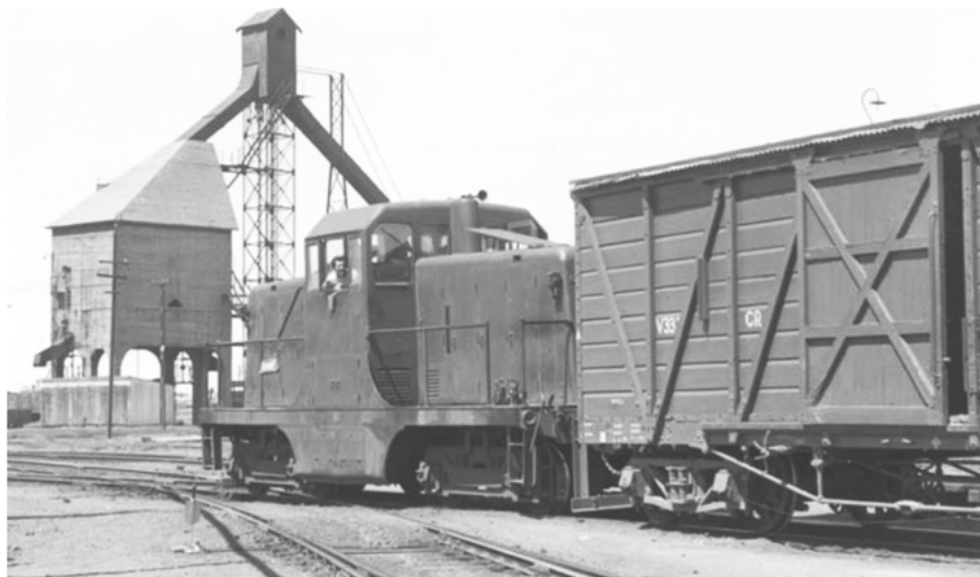
Commonwealth Railways standard gauge Bo-Bo diesel-electric shunting locomotive DE91 shunting in Port Pirie yard on 28 January 1958. The locomotive is passing over a diamond crossing, while the coaling tower at the SAR locomotive depot dominates the background. DOUG COLQUHOUN PHOTO
