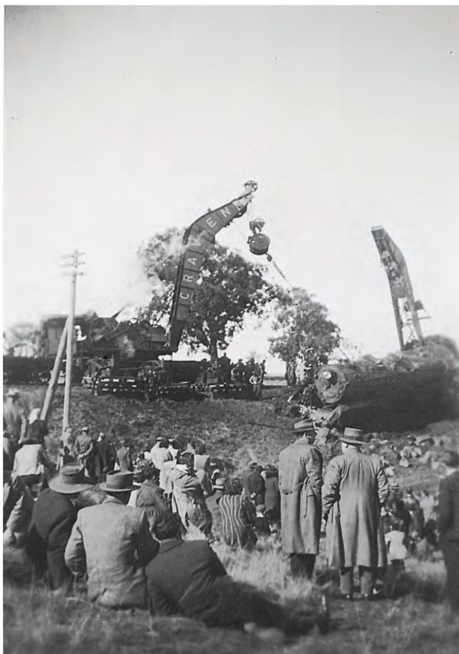
With spectators watching on, Keith Chiplin's Broadmeadow breakdown crew on crane 1072 (at left) work in combination with the Enfield breakdown crew on crane 1073 to recover locomotive 3817 at Rocky Ponds on 2 July 1948. Despite the saturation newspaper coverage this accident attracted, the recovery of the locomotive was achieved without incident and received little attention from the papers. 12
