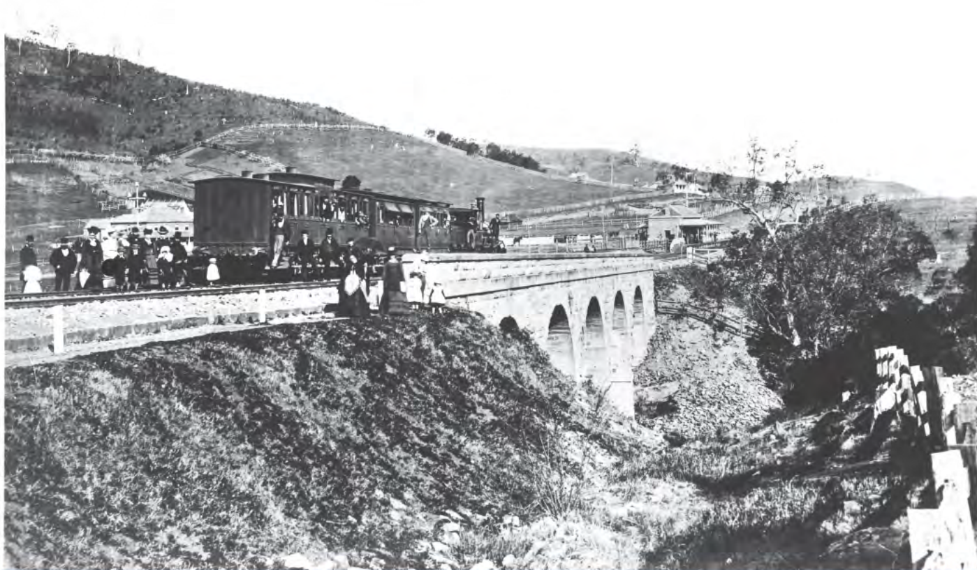
A passenger train on the Stonequarry Creek viaduct at Picton in 1897 with the station in the background. Passengers of both sexes have detrained to pose for the camera. Thomas Firth was supervising engineer for construction of the line from Liverpool to Picton. C C SINGLETON COLLECTION, ARHSNSW RAILWAY RESOURCE CENTRE, 005139
