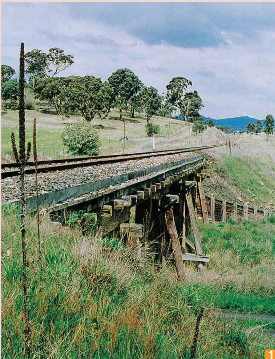
A Whitton-era ballasted deck timber trestle bridge on the Queanbeyan to Michelago section of the Cooma line, photographed by the author on 15 October 1999.
