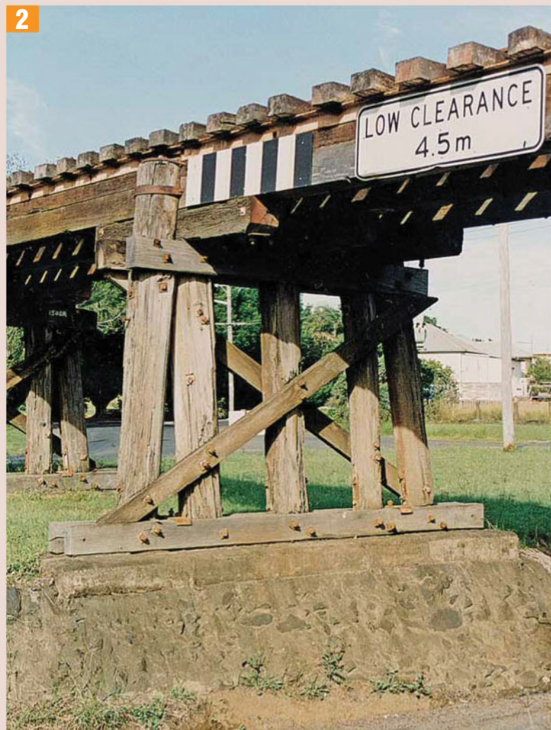
A transom top timber trestle bridge with double-girder spans, requiring a five-pile pier, secured by a concrete base on the trestle bridge spanning Union Street on the now closed Murwillumbah line at North Lismore on 1 May 1995. Photo by the author.
