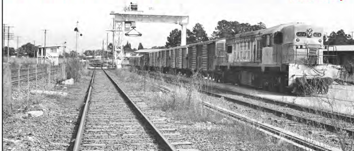
QR GM loco 1474 and covered (or box) wagons photographed on the 1970s-built dual-gauge siding in the Salisbury depot in 1979. The closer gantry line siding was 1435mm gauge as was the run-around line in foreground. The signal cabin is on the left. GREG CASH IMAGE
