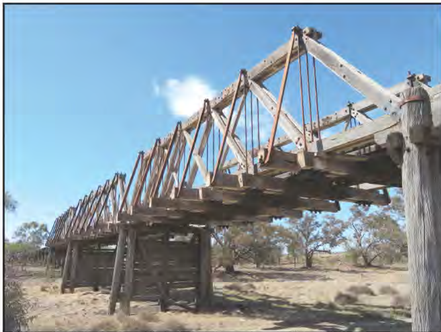
The timber truss bridge over Two Mile Creek near Walgett. Built in 1908, this bridge had three through truss spans, each 60 feet in length, together with 20 x 24ft and 10 x 24ft timber girder approach spans. The lack of rain is evident in this August 2017 view.
