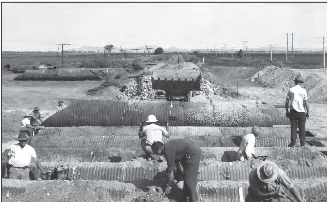
Bridge gang restoring Armco pipe culverts between Gunnedah and Narrabri in 1971. FRANK JOHNSON IMAGE
