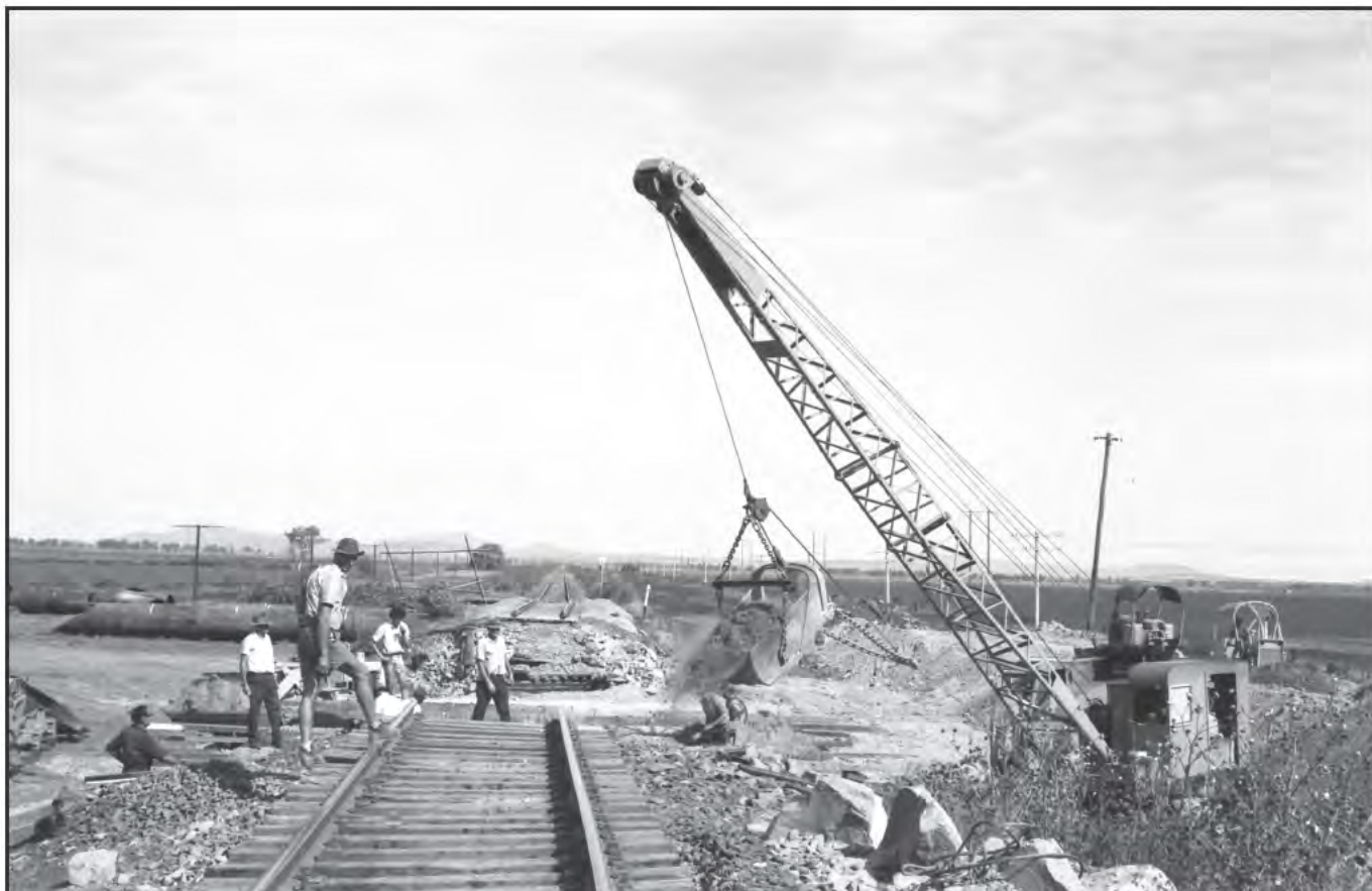
Bridge gang and earthmoving equipment restoring the Armco pipe culverts between Gunnedah and Narrabri in 1971.
