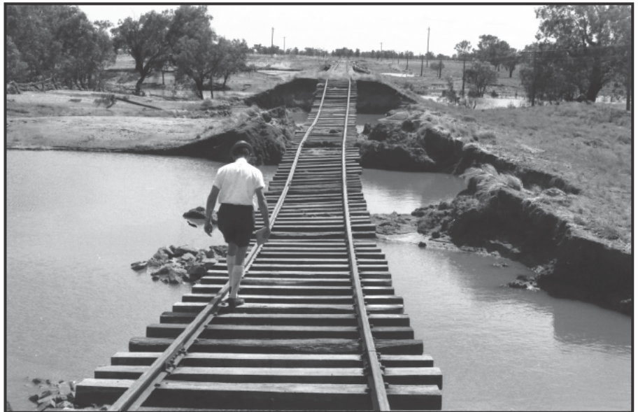
Inspecting Engineer Ken Swan inspecting a washaway between Narrabri and Bellata in January 1971. FRANK JOHNSON IMAGE
