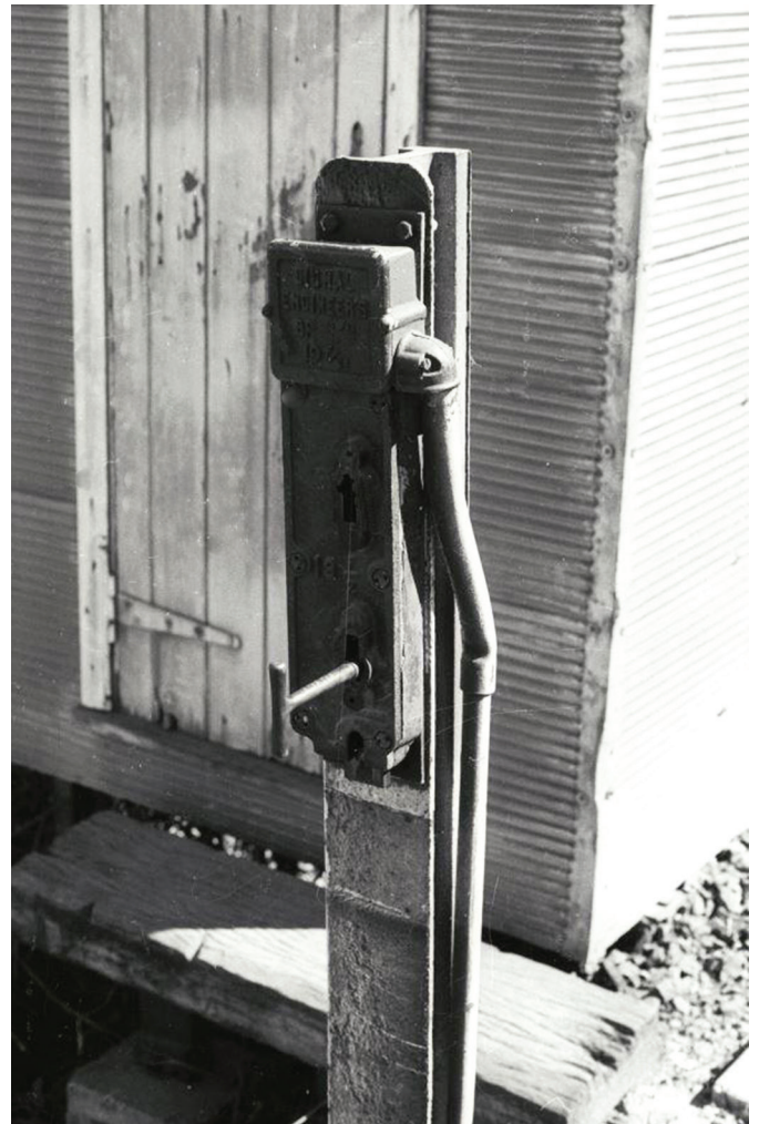
The Duplex Lock B at Salisbury with its Annett key plus electrical connections on top in 1982. P BARKER IMAGE
