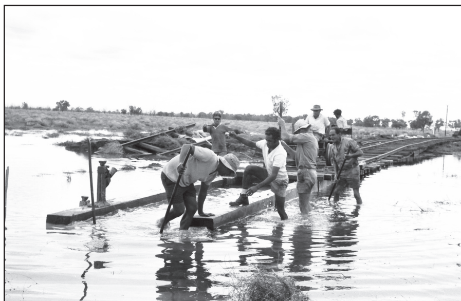
Members of the local track gang working in flood waters to construct the new deviation near Cryon in March 1971. FRANK JOHNSON PHOTO
