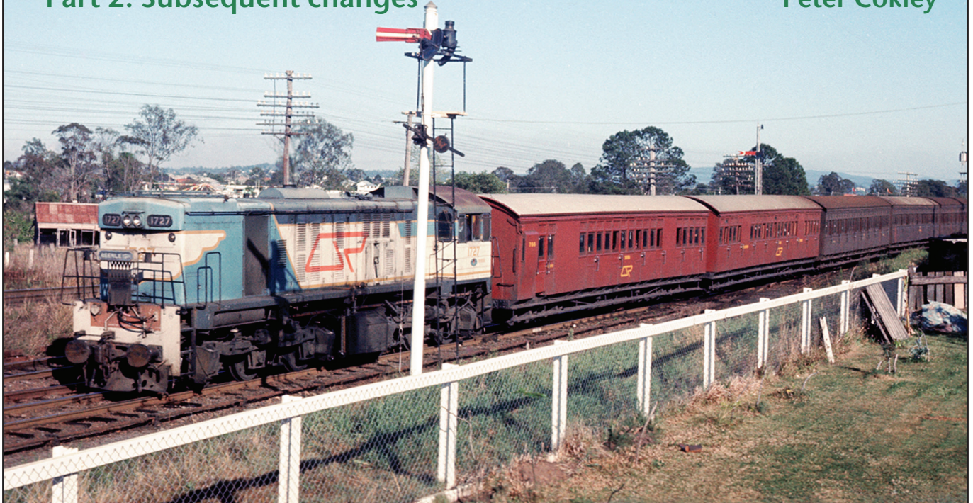
A standard NSW signal passed by a QR Beenleigh bound train near Salisbury yard in the late 1970s. The prominent NSWGR shunting signal No. 3B Sidings to Main is explained in the text. GREG CASH PHOTO
