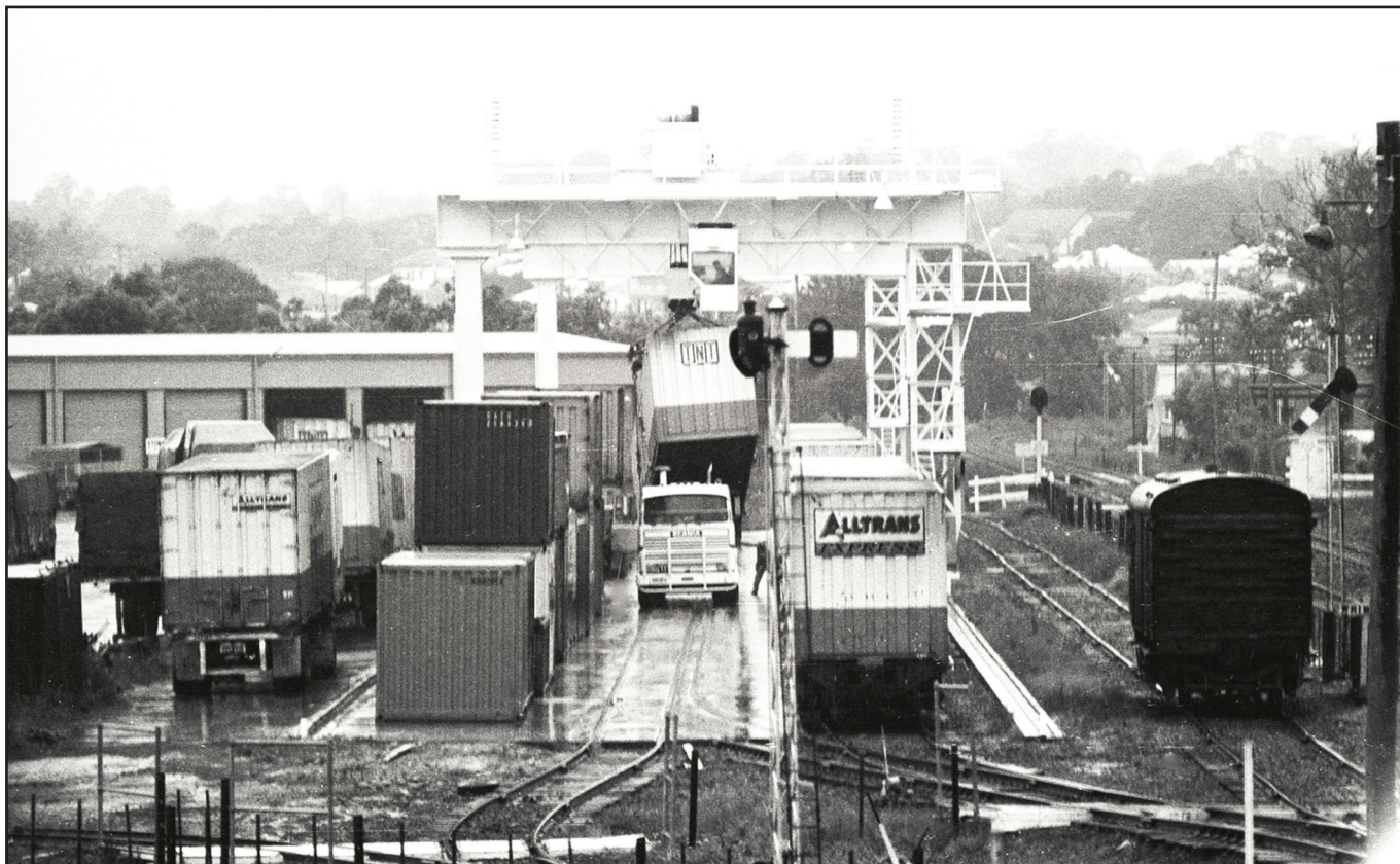
A TNT container is loaded onto a motor truck standing on the dual gauge track by the overhead gantry at the TNT Salisbury container facility in 1978. GREG CASH PHOTO
