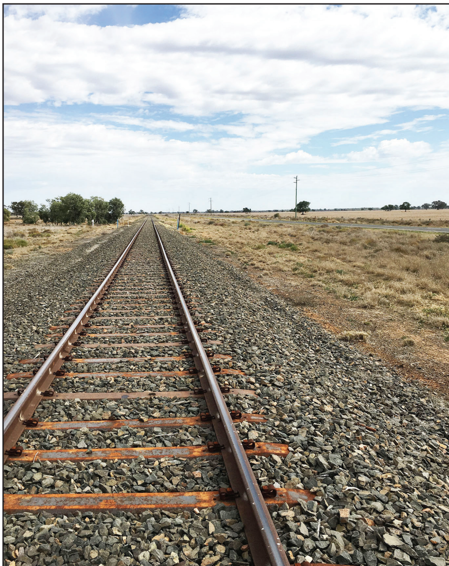
Upgraded track at Bugilbone between Burren Junction and Walgett with steel sleepers and new stone ballast in September 2017. FRANK JOHNSON PHOTO
