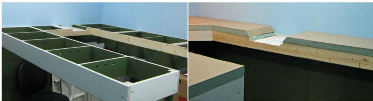
These two photos show the basic construction Tom used to build the GNRR: conventional grid benchwork with wiring holes overlaid with 2"-thick extruded-foam insulation board. The notched areas are for the creek and river sections.
