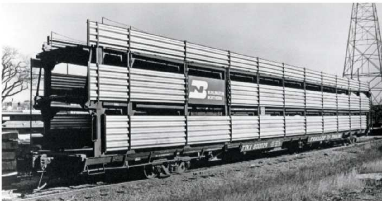
12 This hinged-end, 89'-4" tri-level was fitted with corrugated side panels by the early 1970s. The Burlington Northern herald on a smooth panel takes the place of a corrugated panel. Trains magazine collection
