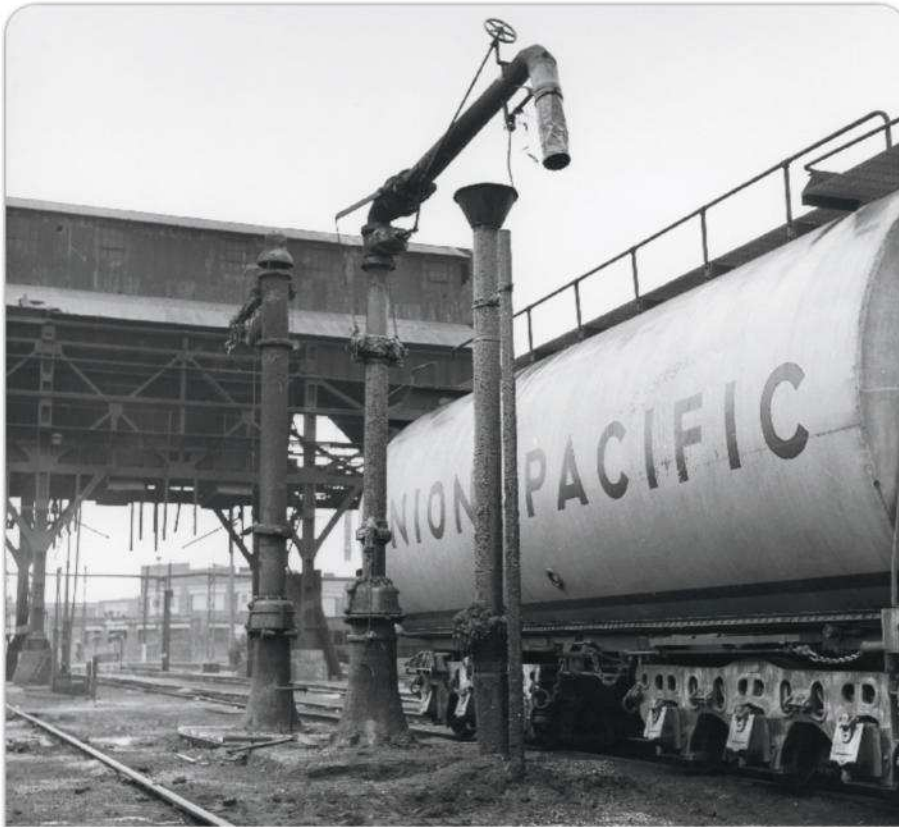
The middle standpipe in this photo is a fueling stand that used to serve oil-burning steam locomotives in Union Pacific's yard in Cheyenne, Wyo. The far standpipe is a water column. David P. Morgan Memorial Library collection
