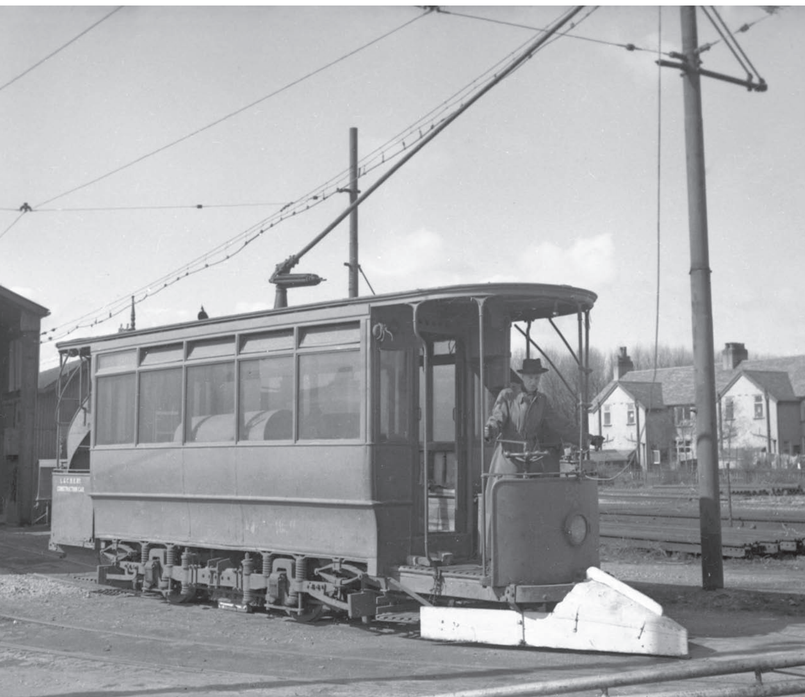
No 23A had been converted to a railgrinder by Bournemouth Corporation in 1921; the L&CBER acquired the tram for works duties in 1936. R.W.A. Jones/Online Transport Archive
