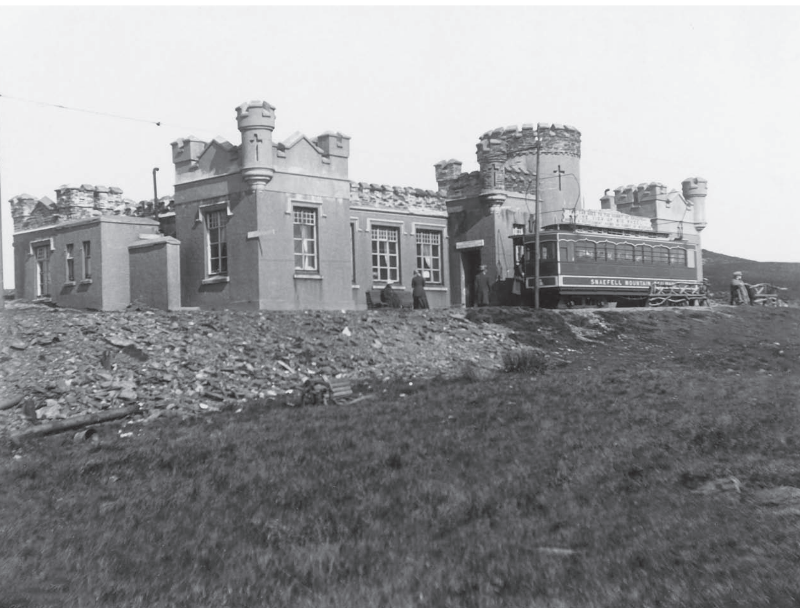
Snafell Mountain Railway no 4 pictured at the Summit hotel. When the line was opened in 1895 a simple wooden structure was built for passengers. Very quickly as passenger traffic increased, this basic structure proved insufficient and so a new stone-built castellated structure was completed in 1902. This is the building featured in this view; however, this was to be destroyed by fire in 1982 and it was not until 1984 that a replacement building was completed. Barry Cross Collection/Online Transport Archive
