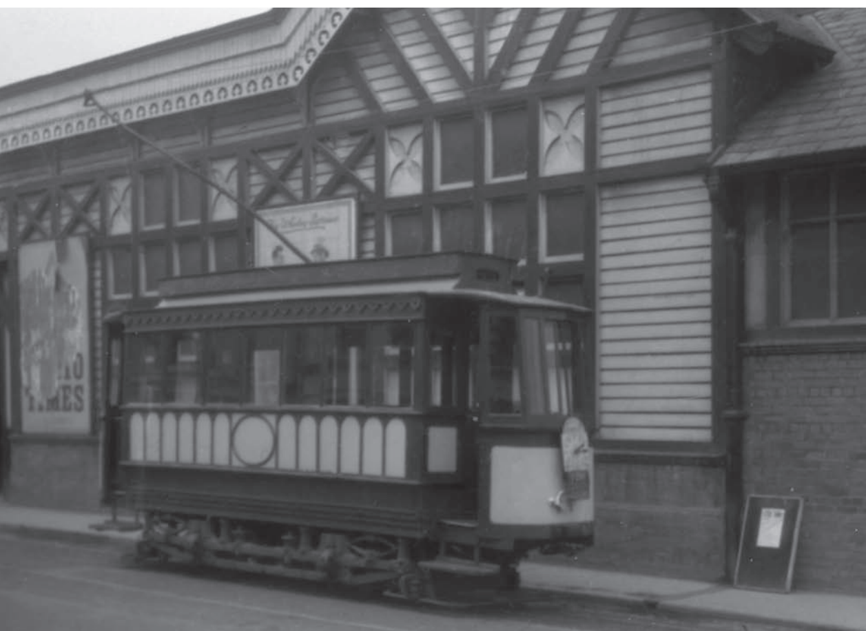
Giant's Causeway No 9 is pictured at Portrush on 7 June 1948; this is after the car was modified through the use of the ornate side panels recovered when No 3 was dismantled. John Meredith/Online Transport Archive
