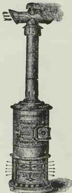
Anti-Clinker Car Heater and Ventilator, for Anthracite or Bituminous Coal.
