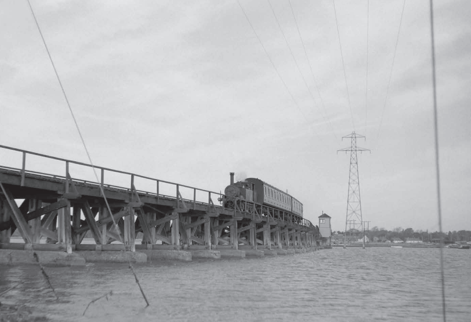
A beach level view of the viaduct showing the timber construction of the structure and the signal box, controlling the swing bridge, taken from the North Hayling side. (Online Transport Archive)
