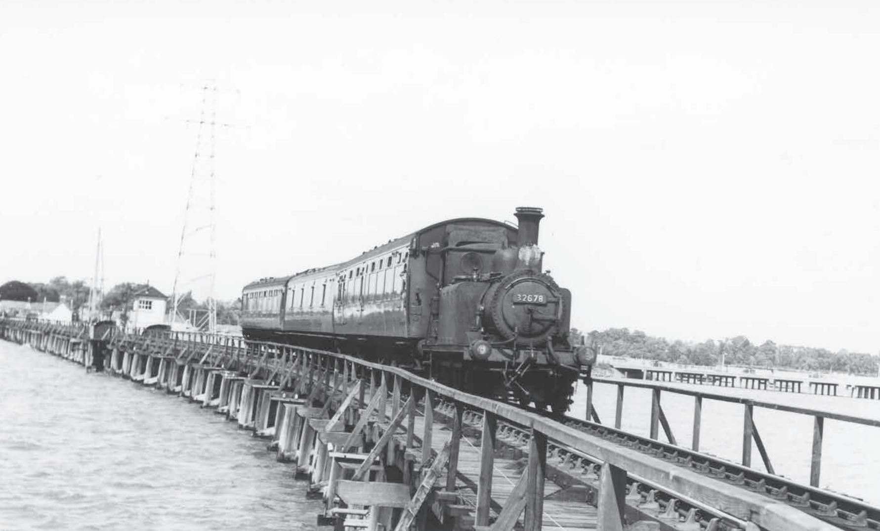
32678 heads a train of Maunsell and Bulleid carriage stock towards North Hayling, on 4 August 1962. This illustration shows in detail the complicated timber construction of this structure, which was a contributory factor in the line's closure. The need for renewals and the cost of maintenance almost guaranteed the line's eventual demise. Note the new road bridge in the distance, which could have been designed with a separate rail deck, to allow trains to cross on one side. (J.H. Aston)
