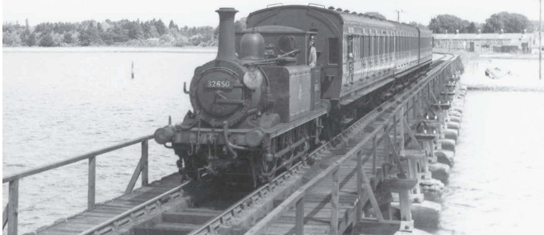
In this mid-1950s picture, 32650 heads a train of Ex-L&SWR non-corridor stock, across the timber viaduct. This picture shows the construction and design of the viaduct to good effect, detailing the decking and stanchions which, in Southern Railway days, were strengthened and set in concrete, to prevent rotting to the lower timbers. (Author's Collection)
