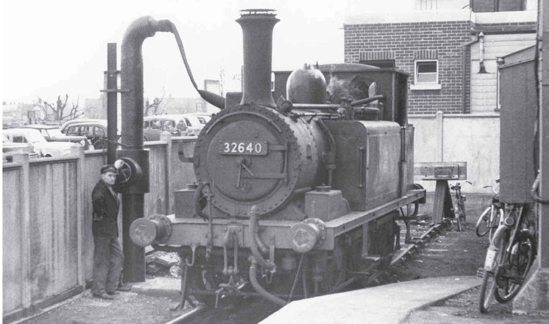
32640 takes water at the far end of Havant station on 6 April 1956, a study of the large size of the L&SWR water crane and the miniature Victorian tank locomotive. (Graham T.V. Stacey)
