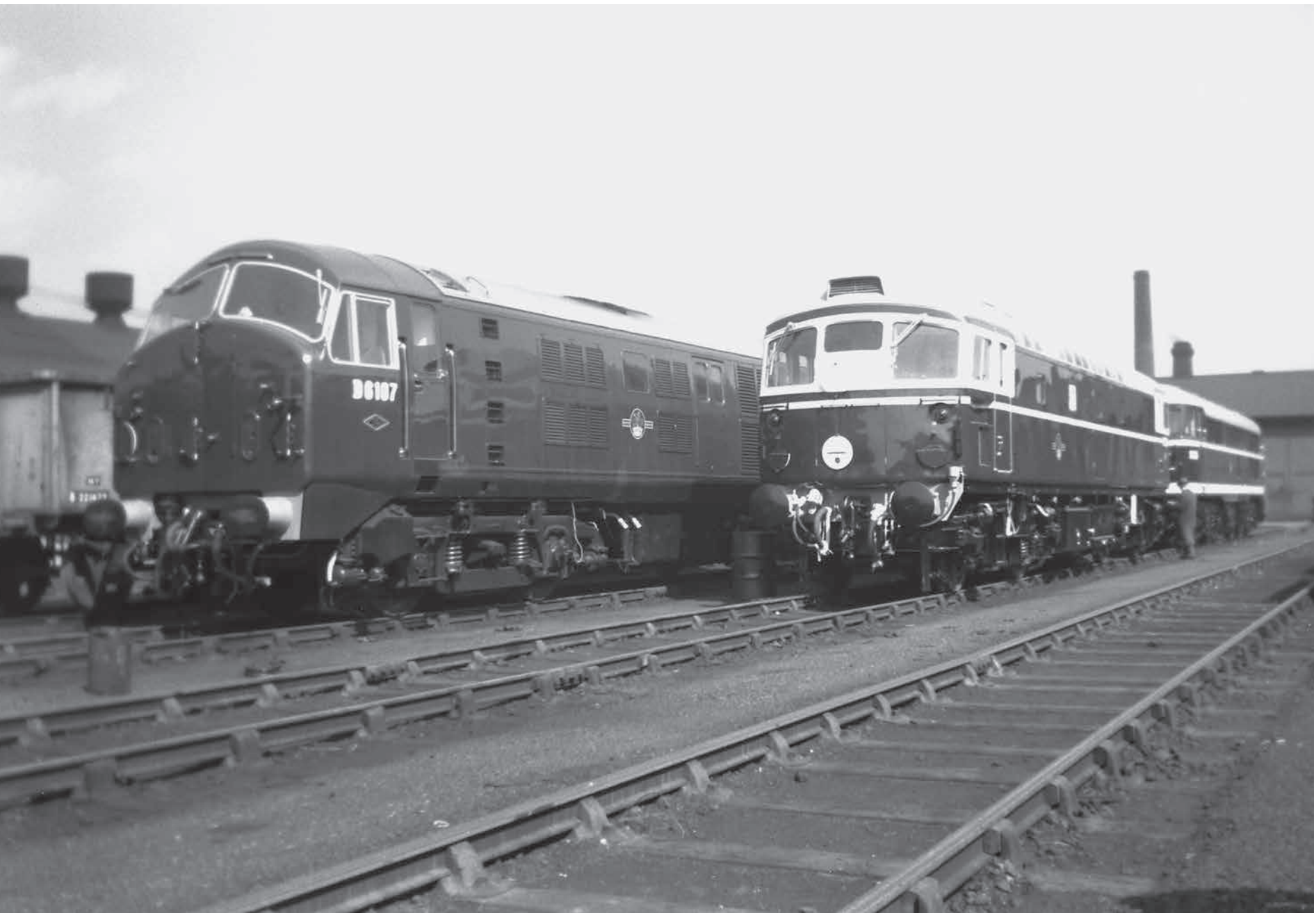
D6107, Doncaster Works, April 1959. D6107 undergoing acceptance testing prior to entry into traffic at Hornsey. It is fitted with the early style main radiator grilles just visible to the left of the BRCW Type 2 (Class 26). (Author's Collection)
