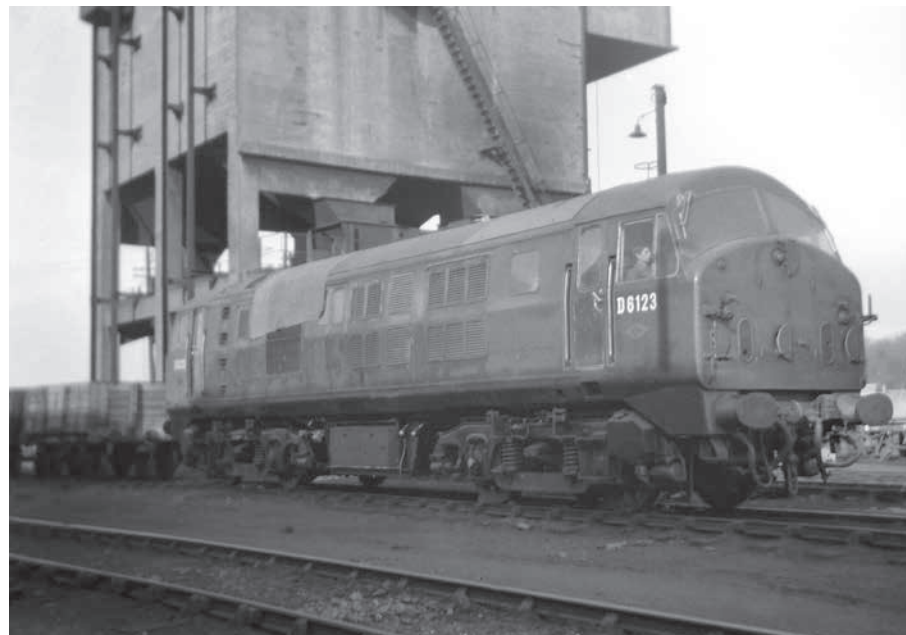
D6123, 12A Carlisle Kingmoor, Undated but presumed to be March 1963. After preparation work at St.Rollox Works, D6123 was transferred to Davey Paxman, Colchester for installation of the new Paxman 'Ventura' engine, stabling at Carlisle Kingmoor on route. The additional bodyside grilles and the guttering rails over the bodyside grille cluster have already been fitted. Self evidently, D6123 was one of the Class 21s which retained green livery without the yellow warning panels (and without 25kV warning signs) upto the point of conversion to a Class 29. (Howie Milburn)
