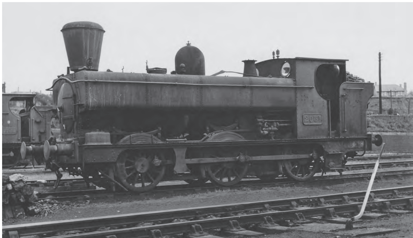
2051 , built in October 1898, and rebuilt as a pannier tank in 1923, at Kidderminster, fitted with spark arresting chimney, 12 November 1950. It was withdrawn from that depot in July 1951. (MLS)
