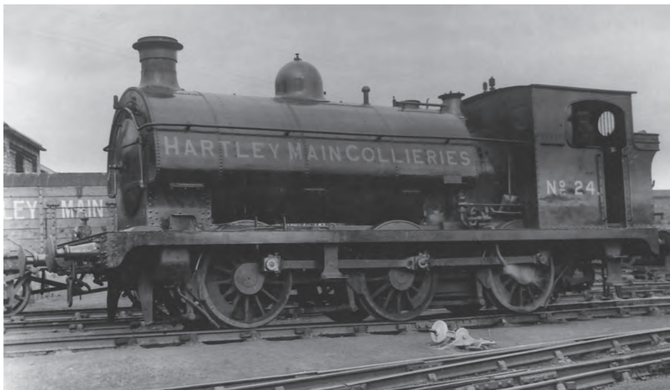
Barry 'F' saddle tank, formerly No.724, built in March 1900 and sold to the Hartley Main Colliery in May 1933, where it was renumbered 24. It was retained by the NCB and was scrapped in April 1960. (GW Trust /P.J. Reed Collection)
