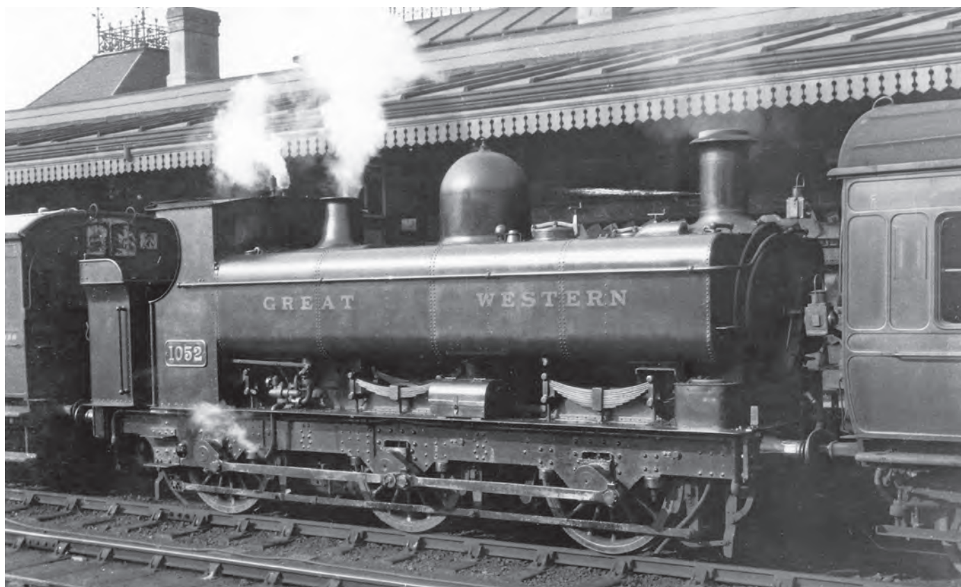
1052 , built in November 1870 at Wolverhampton, waiting at Cardiff General with a local passenger train, c1924. It had been rebuilt with pannier tanks in August 1923 and was withdrawn in September 1929. (John Hodge Collection)
