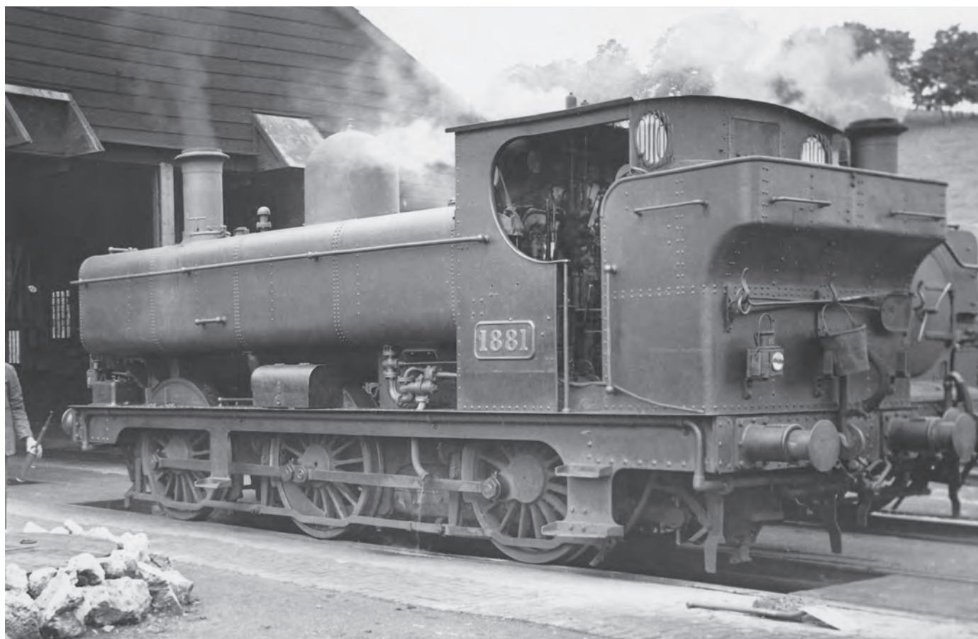
1881 , built in December 1890, rebuilt with pannier tanks in November 1918 and later with enclosed cab and enlarged bunker, at Yeovil, 13 July 1936. (F.K. Davies/John Hodge Collection)
