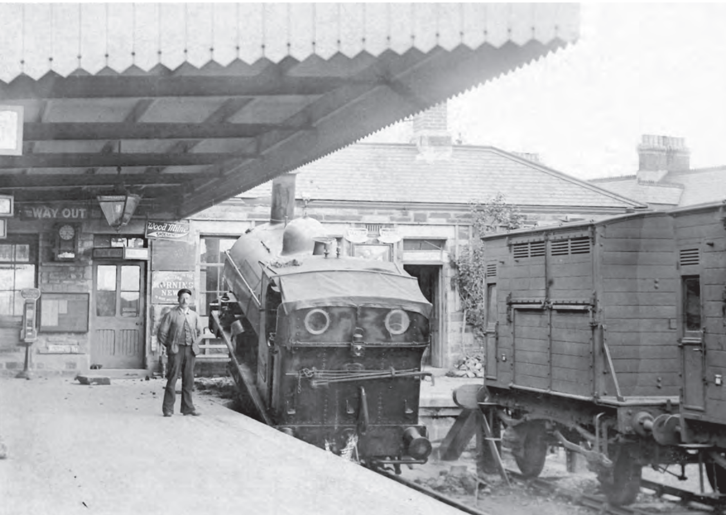
1905 , built in 1881, after collision with the buffer stops in the platform at Bodmin Town station, c1910. It was rebuilt as a pannier tank in 1926 and withdrawn from Laira in 1936. (GW Trust/P.J. Reed Collection)
