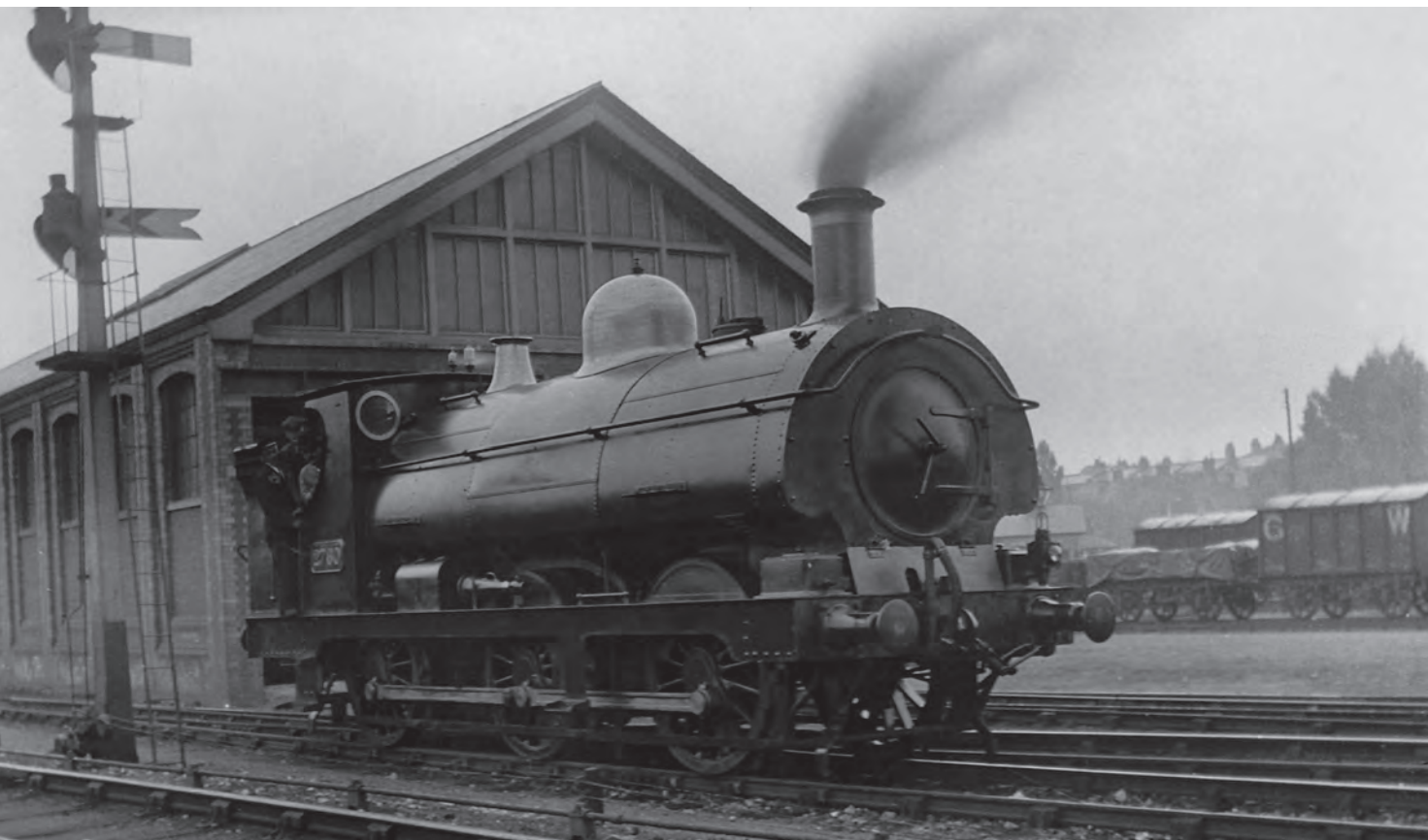
2760 , built as a saddle tank, in August 1899 at an unknown location before building with pannier tanks in March 1916. (MLS/T. Guest)
