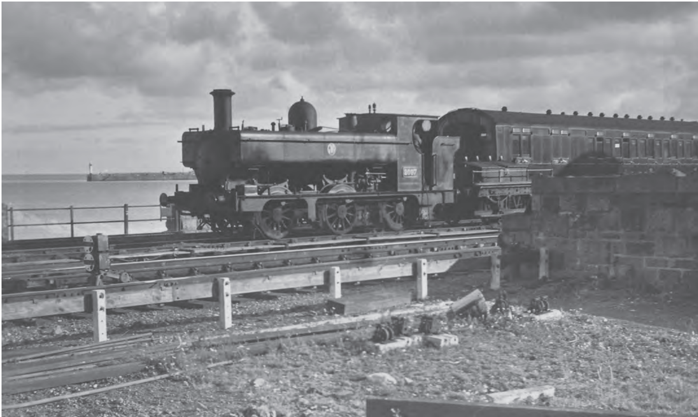
2097 , built in July 1901, rebuilt with pannier tanks, enclosed cab and enlarged bunker, shunting at Penzance, 12 July 1938. It was not withdrawn until March 1955. (MLS)
