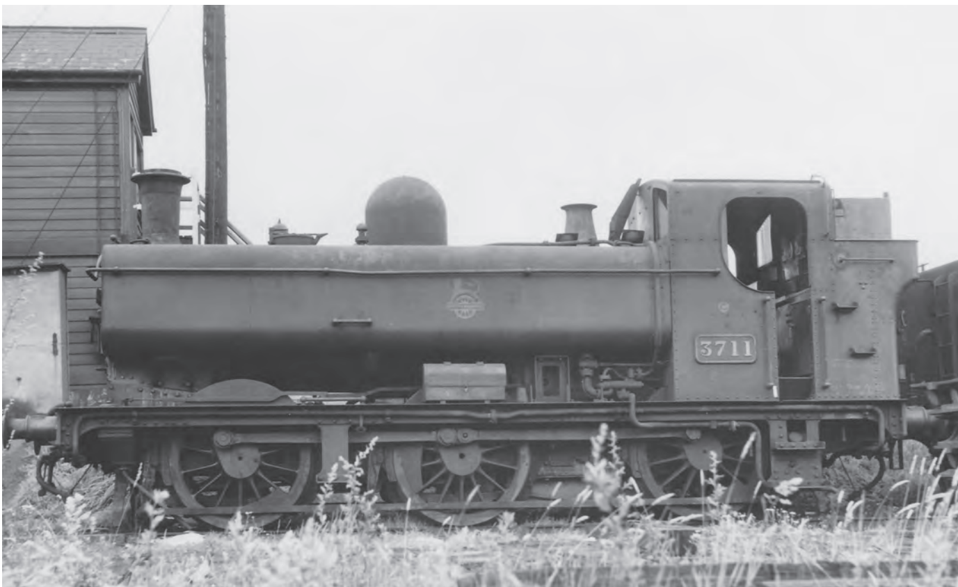
Aberbeeg's 3711 at Swindon Works after conversion to oil firing, 27 July 1958. It was then reallocated to Old Oak Common for trials on the empty stock working to Paddington. The oil tank is visible on the bunker. (MLS)
