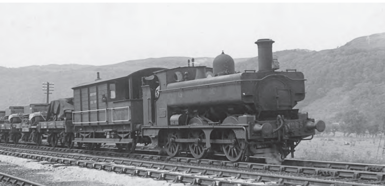
1985 , built in 1891 and rebuilt as a pannier tank in 1925, on a freight at Fowey, c1946. It was withdrawn from Laira in 1949. (GW Trust/P.J. Reed Collection)
