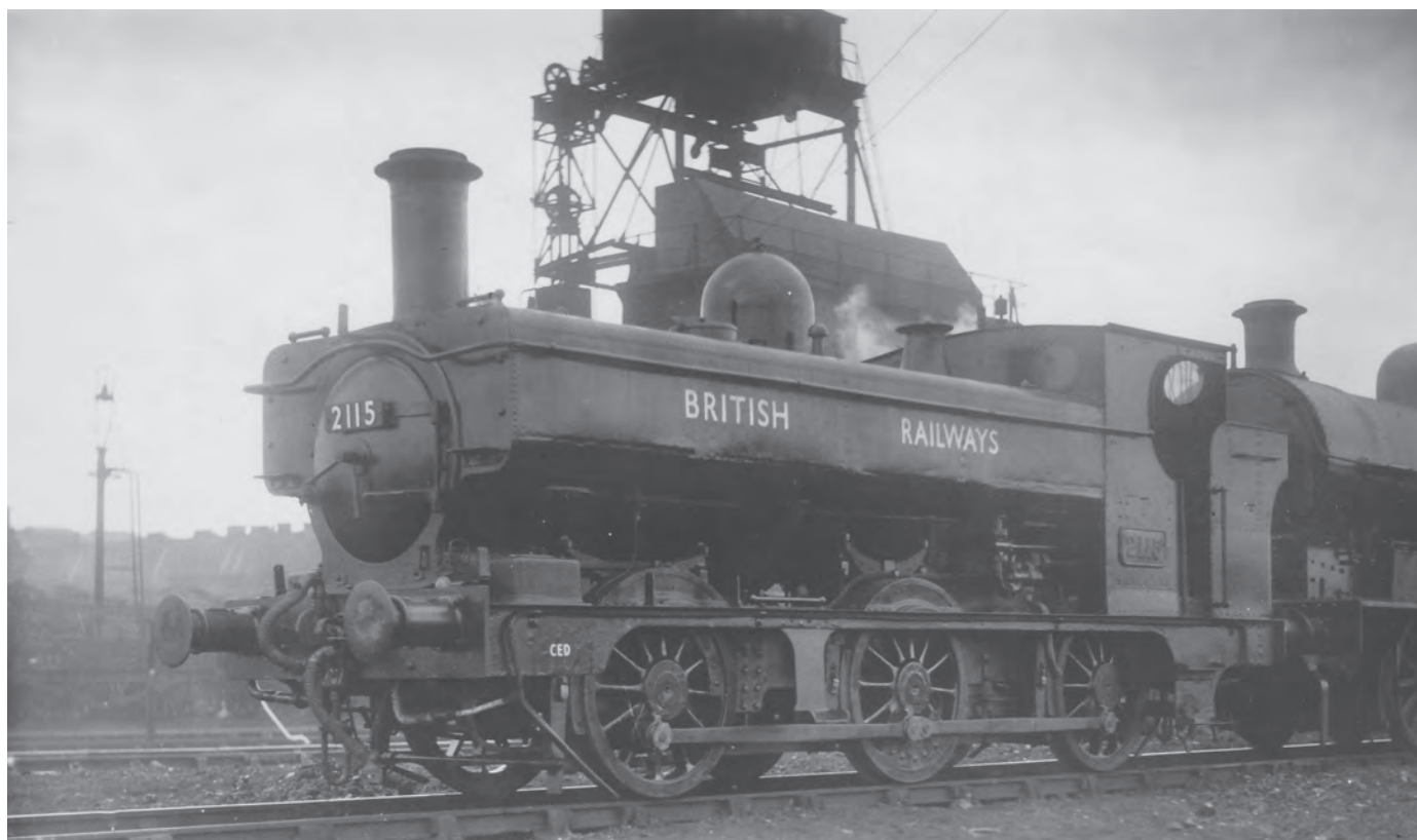
2115 , recently outshopped in BR livery, c1949. It is stabled next to a LNER 0-8-0 at an unknown shed location, probably Shrewsbury or Chester. 2115 was built in October 1902, rebuilt with pannier tanks, enclosed cab and enlarged bunker in March 1913 and was withdrawn in June 1952. (MLS)
