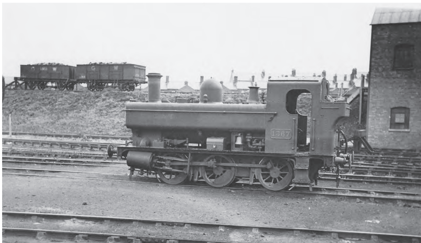
1367 at Weymouth with the dock warning bell clearly visible on the running plate under the pannier tank, 12 July 1936. (F.K. Davies/John Hodge)
