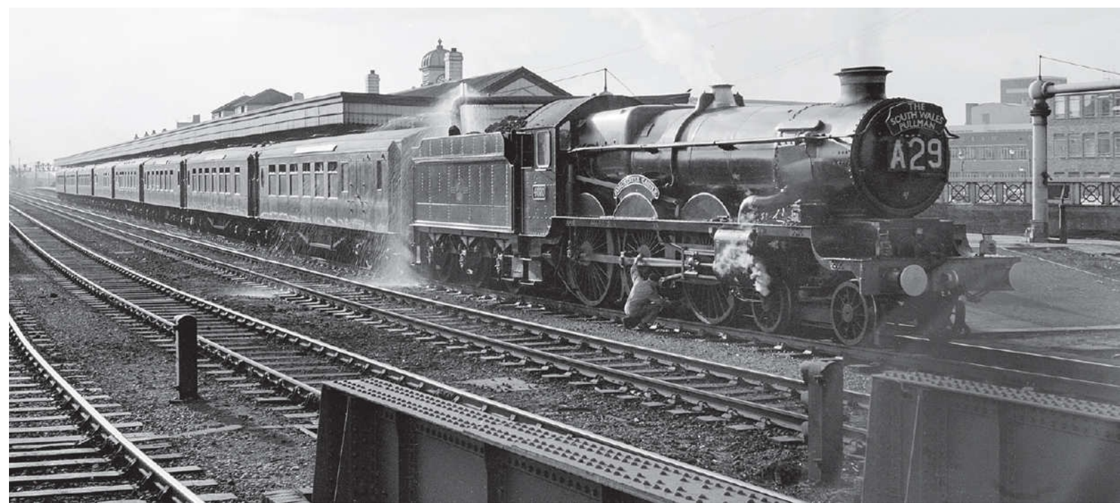
Double chimney GWR 'Castle' class 4-6-0 No 4090 DORCHESTER CASTLE takes water at Cardiff as it heads the last up steam hauled 'South Wales Pullman' on 8th September 1961. The duty fitter appears to be examining the off side brake gear. Note the extended smokebox, modified steam pipes, double chimney, external sandboxes, stepped inside cylinder cover and burnished buffers. Hugh Ballantyne/Rail Photoprints
