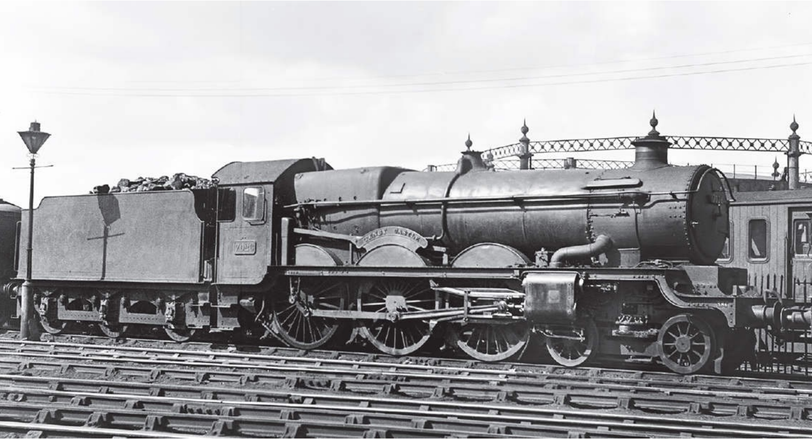
BR/WR ‘Castle’ class 4-6-0 No 7026 TENBY CASTLE is seen at Stafford Road (84A) in 1955. Note the Hawksworth 4000g tender without a logo and also the mechanical lubricator in the original position and un-stepped inside cylinder cover. Rail Photoprints Collection
