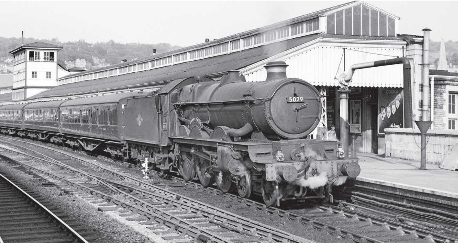
GWR ‘Castle’ class 4-6-0 No 5029 NUNNEY CASTLE calls at Bath Spa station with the 4.33 Salisbury – Bristol service on 31st May 1962. Note the low ended roof of the brake immediately behind the engine. Hugh Ballantyne/Rail Photoprints
