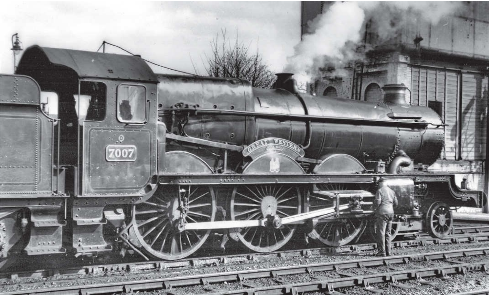
GWR ‘Castle’ class 4-6-0 No 7007 GREAT WESTERN is seen at Oxford station in 1959. Note the GWR crest on the centre wheel splasher below the nameplate, also the mechanical lubricator behind the modified style outside steampipe. David Anderson
