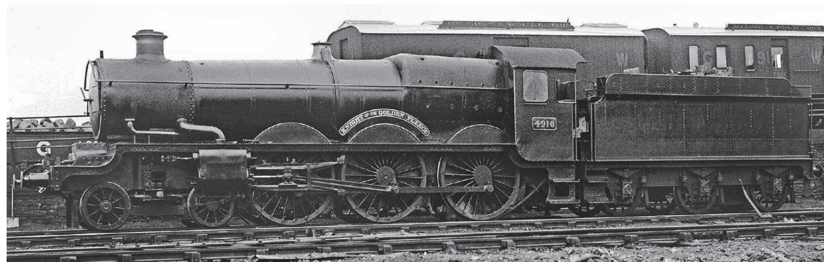
Re-built from a 'Star' 4-6-0 'Castle' class No 4016 KNIGHT OF THE GOLDEN FLEECE, is seen at Bristol Bath Road, circa 1933. Note the distinctive brass beading on the cab front edges, cab side windows, number/name plates and wheel splashers. This locomotive also had a cut out section in the bottom cab step support. Ray Hinton
