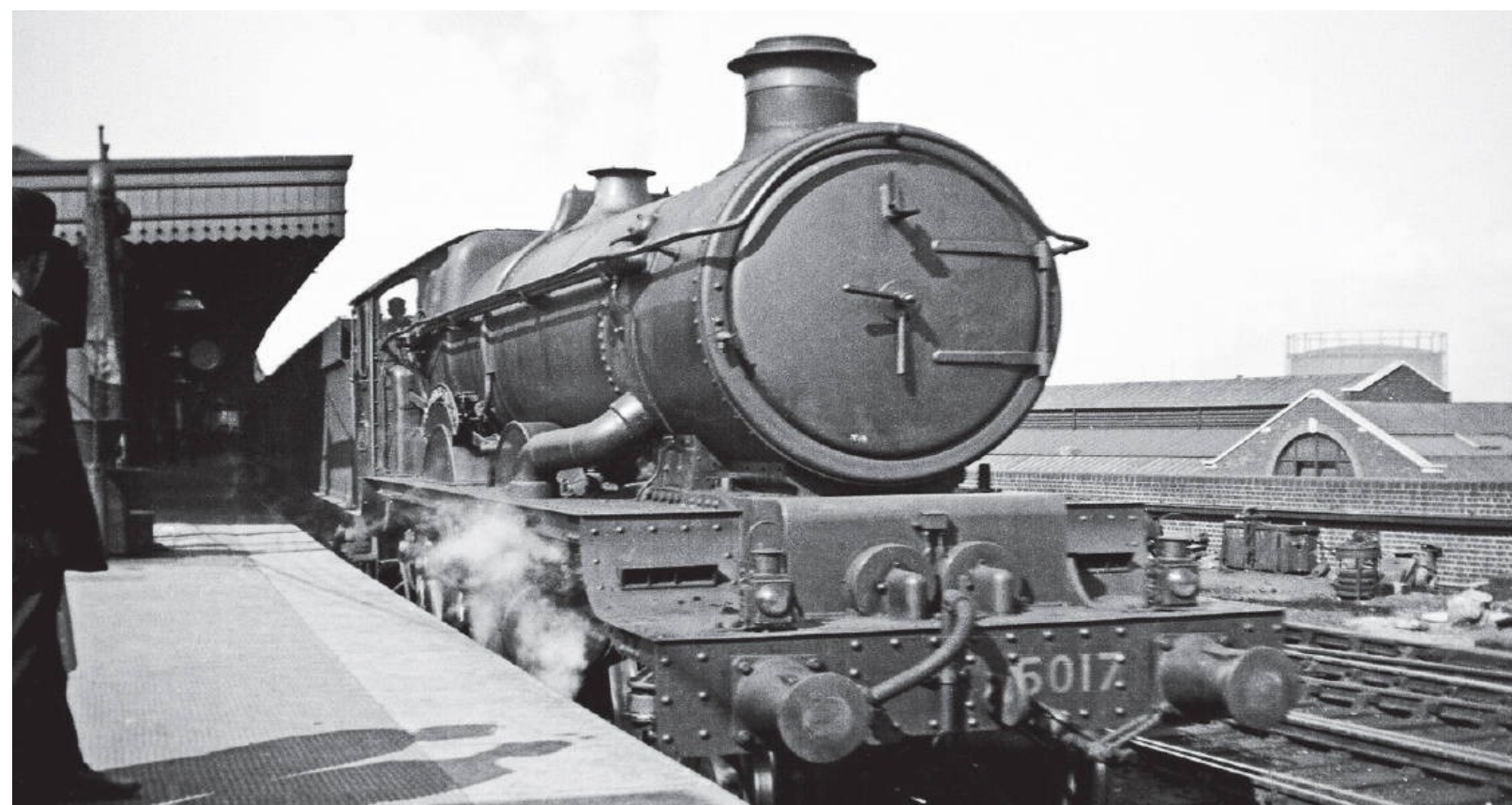
GWR 'Castle' class 4-6-0 No 5017 is seen at Bristol Temple Meads station as St DONAT'S CASTLE in this 1946 image. Note the number stencilled on the right hand front of the buffer beam and the solid looking GWR tapered barrel buffers and 'Box' style inside cylinder cover with round topped front edge. Cresselley Photos
