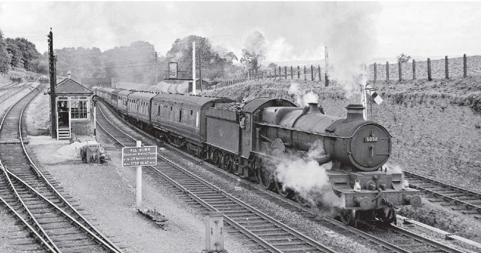
GWR ‘Castle’ class 4-6-0 No 5058 EARL OF CLANCARTY climbs past Dainton Tunnel signal box with a 10 coach Plymouth–Exeter excursion, on 7th August 1961. Note the down line sign instructing drivers of ‘Goods and mineral trains with 35 wagons or less to STOP DEAD’ at that point, in order that unfitted trains could pin down brakes. The large post mounted mirror beyond the up line (above 2nd coach) gave the signalman in the downside box a view into the tunnel. Hugh Ballantyne/Rail Photoprints
