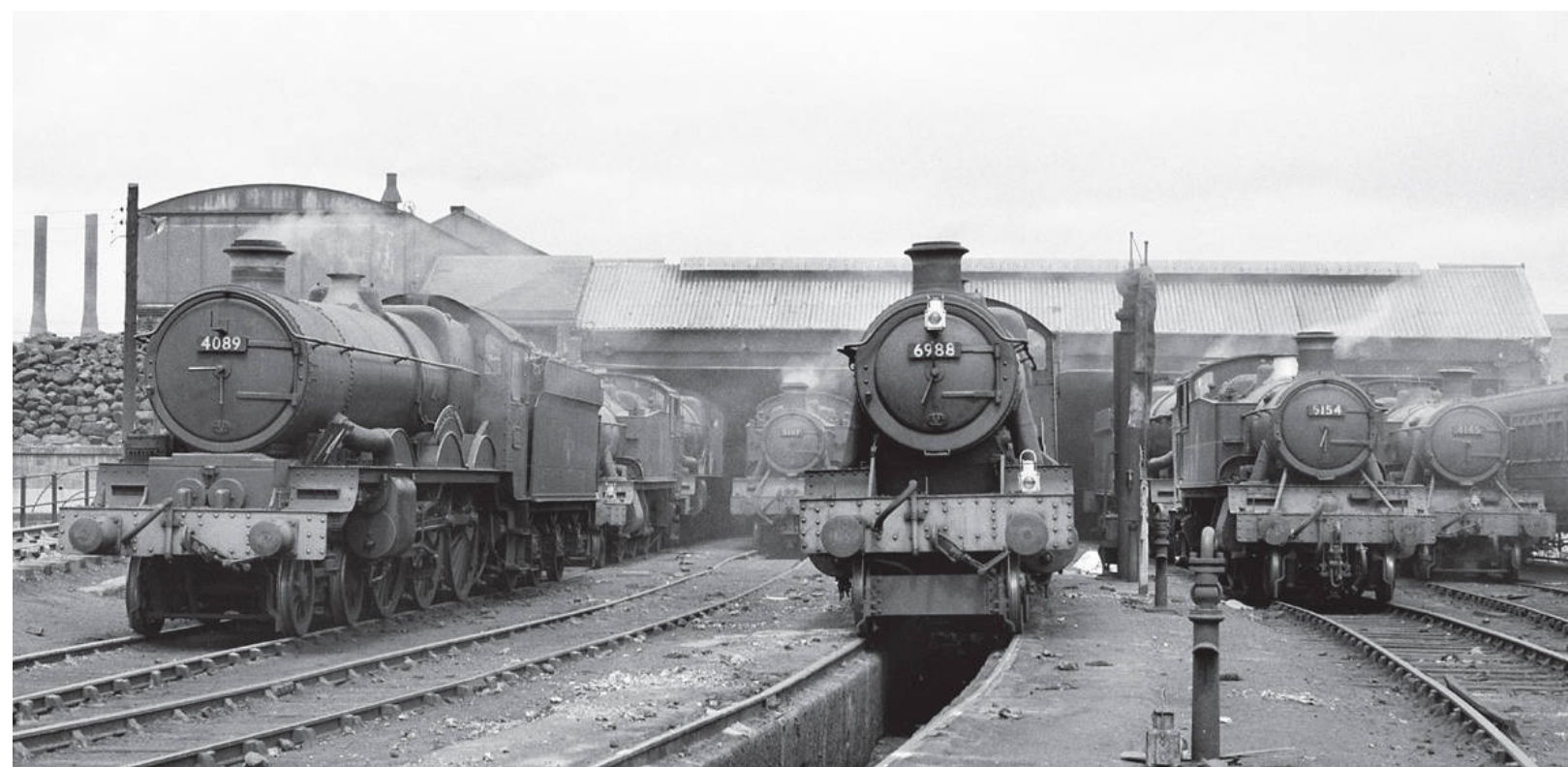
Newton Abbot Shed 18th May 1958, on the left GWR 'Castle' class 4-6-0 No 4089 DONNINGTON CASTLE, note the post modification stepped straight sided, inside cylinder cover. Hugh Ballantyne/Rail Photoprints
