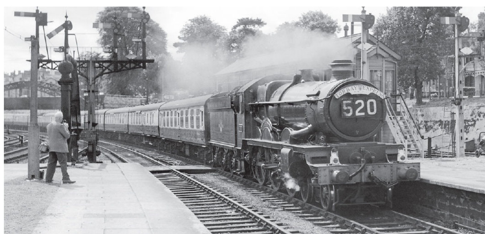
GWR 'Castle' class 4-6-0 No 7000 VISCOUNT PORTAL with a Collett 4000g tender is seen entering Newton Abbot with the up 'Torbay Express', 1959. The 'Torbay Express' London-Torquay-Paignton service was introduced by the GWR as one of its premier holiday trains. A similarly named service still operates in the present day (2014). Note the stepped inside cylinder cover. Rail Photoprints Collection
