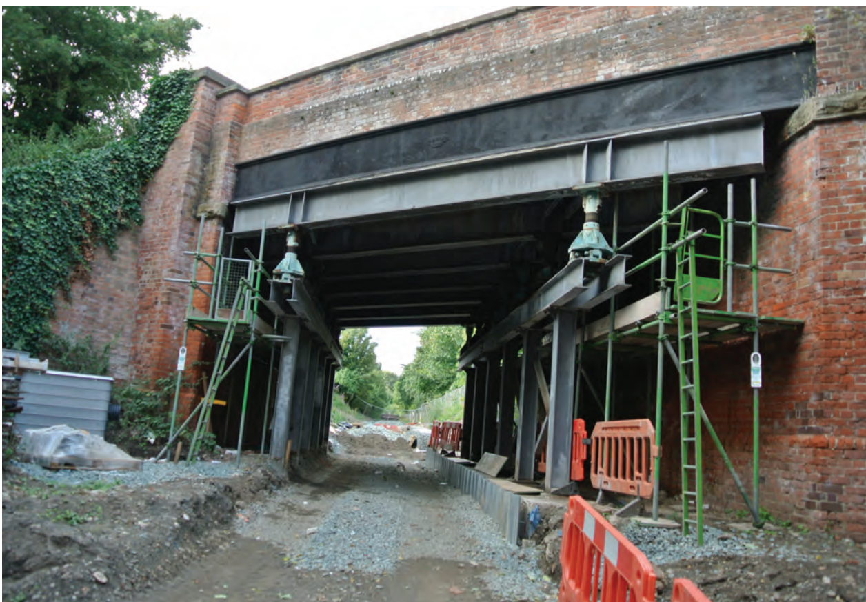
The Gas Works Bridge carrying the main road into Oswestry undergoing strengthening by the County Council to allow trains to proceed underneath to Western Wharf, 9 February 2018. (Paul Carpenter)
