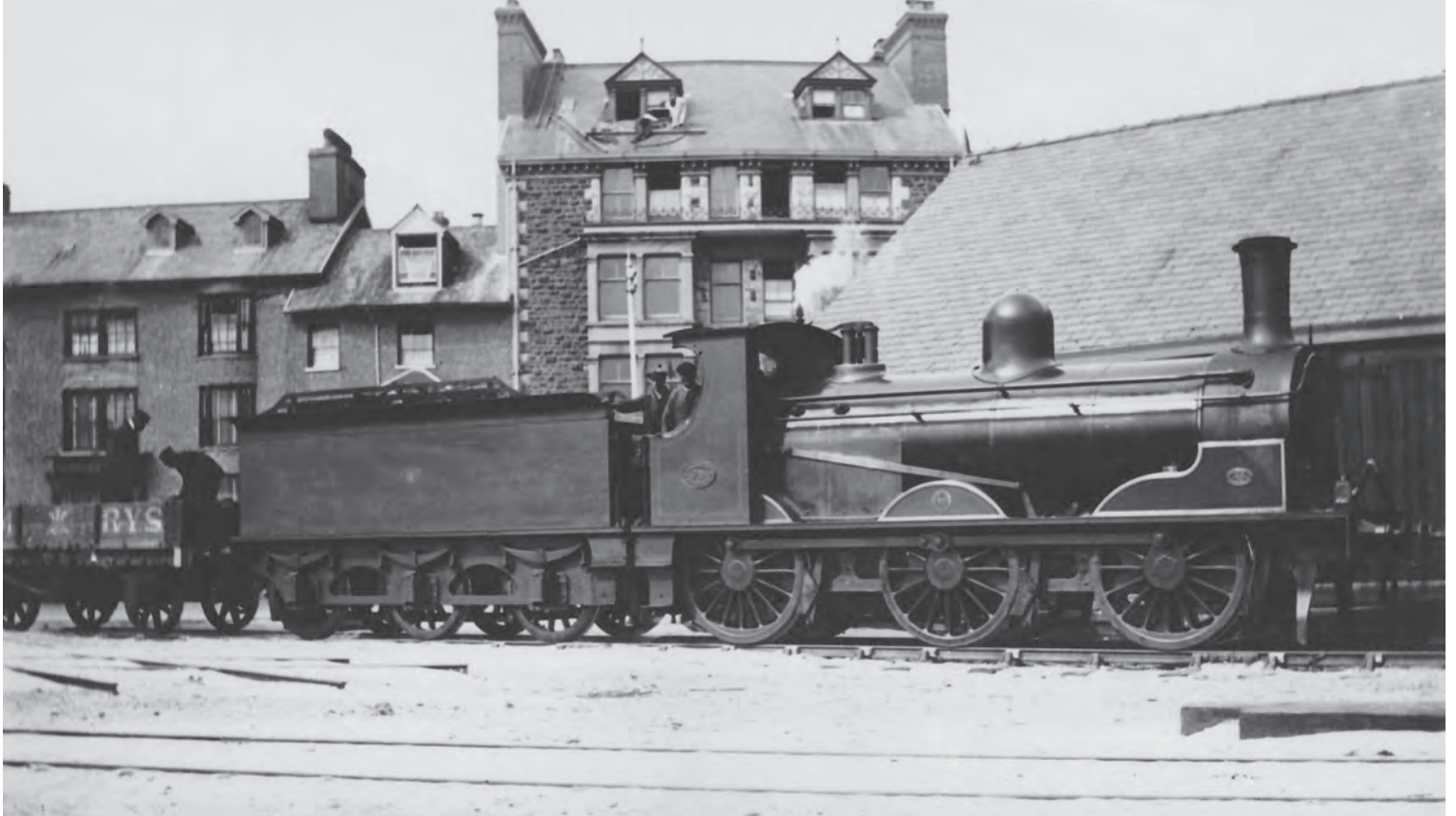
Vulcan Foundry class '73' 0-6-0, No.78, built in 1895, at Machynlleth, 28 June 1909. It was fitted with a superheated boiler by the GW in 1924 and received the number 881, being withdrawn in 1932. It was photographed shunting wagons on the Harbour branch at Aberdovey, c1911. (MLS/R.W. Miller collection)
