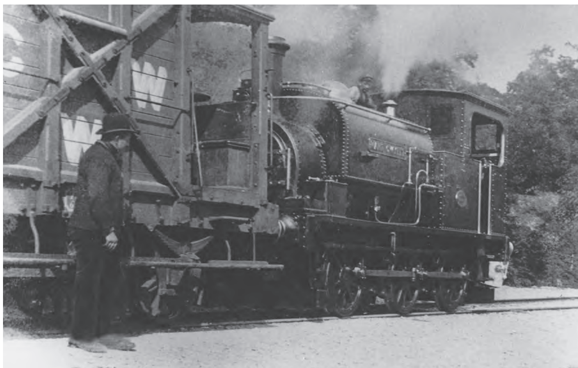
Hunslet Contractor's 0-6-OST Nantgwyllt built for the Elan Valley branch, with Mid-Wales Railway brake van, July 1904. (MLS/R.W. Miller collection)
