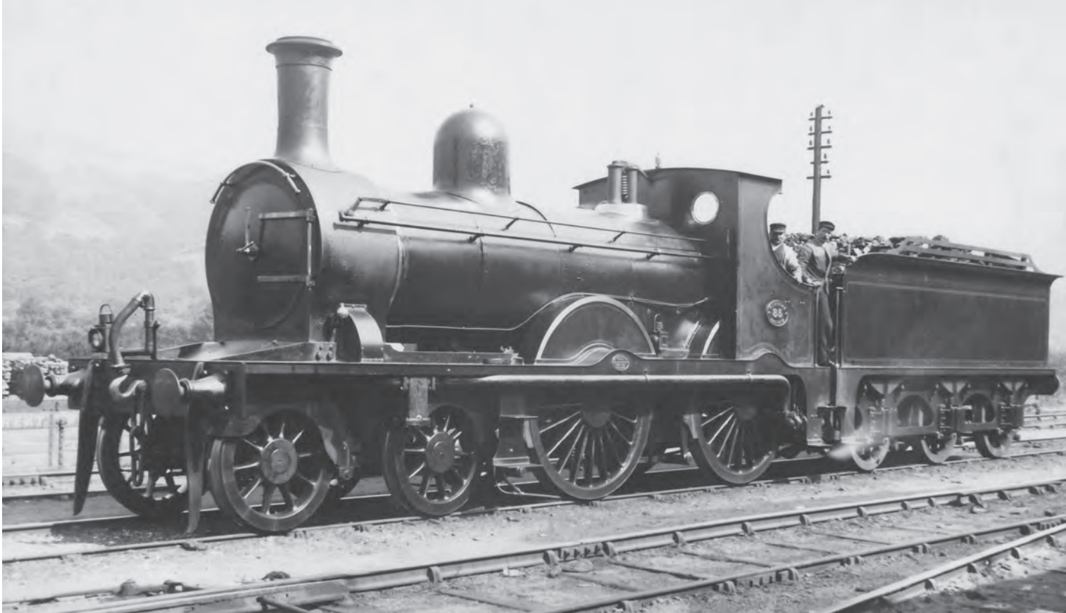
'Large Bogie' No.83, built by Sharp, Stewart in May 1895, reboilered in 1921, photographed shortly afterwards at Oswestry. This locomotive had an excellent reputation and was used for Cambrian Railways royals and was used on the Cambrian Coast Express when introduced by the GWR. As GW 1106, renumbered again as 1110 in 1926, it was the last survivor of its class, being withdrawn in April 1931, offered on the 'Sales List' and not scrapped until 1934.
