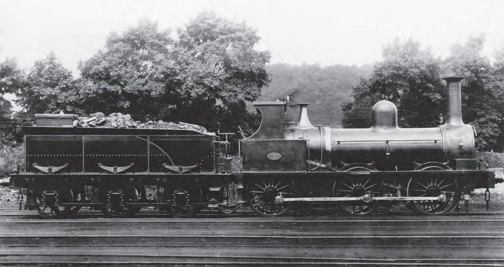
'Small Goods' Sharp, Stewart 0-6-0, No.1, initially named Victoria , built in June 1872, rebuilt in 1891 and seen here immediately afterwards at Oswestry.
