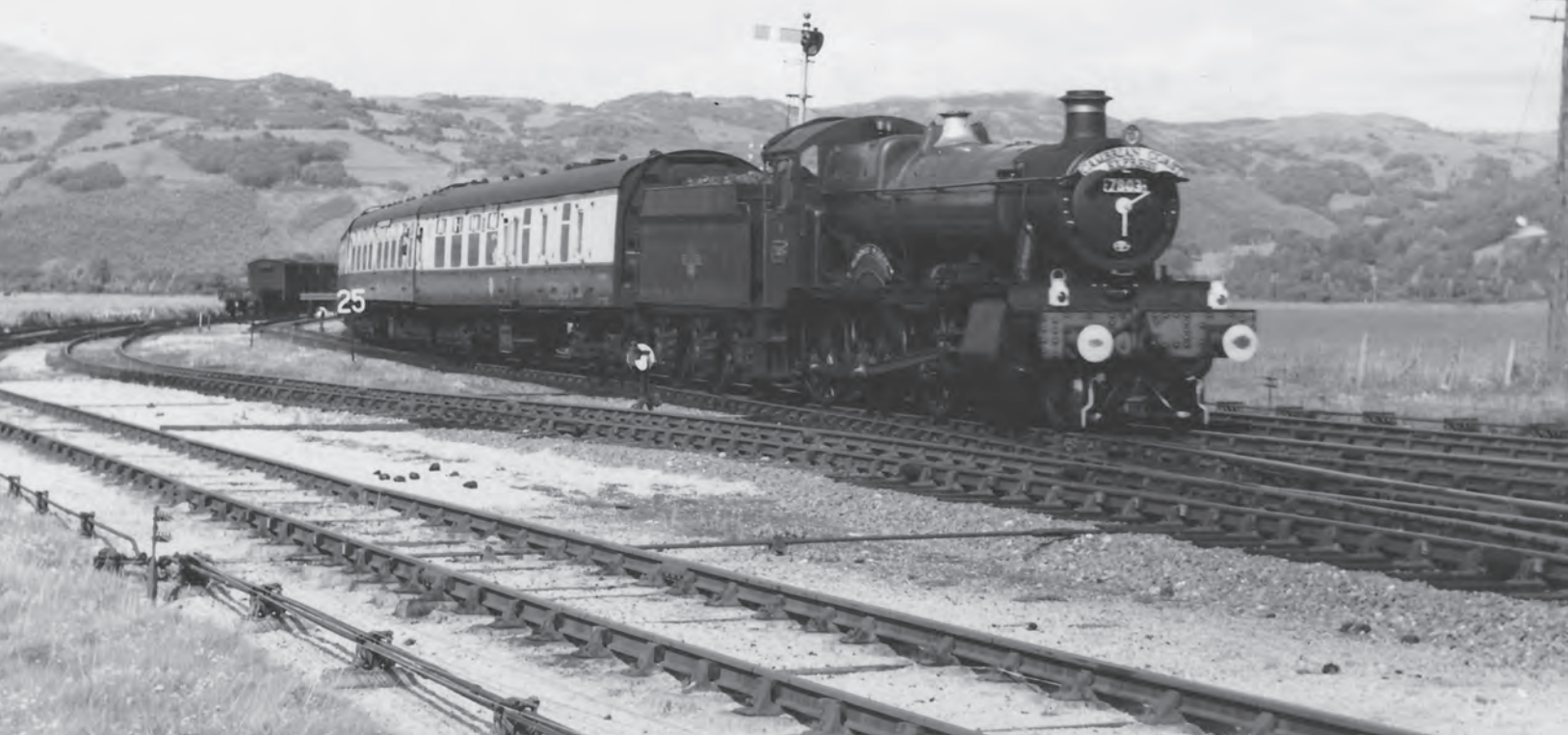
7803 Barcote Manor arriving at Dovey Junction with the Aberystwyth portion of the down Cambrian Coast Express , 24 August 1961. It is formed of Mark 1 chocolate & cream coaches, has the later headboard and 7803 sports a Collett 'intermediate' tender – unusual for a Manor. (MLS/R.W. Miller collection)
