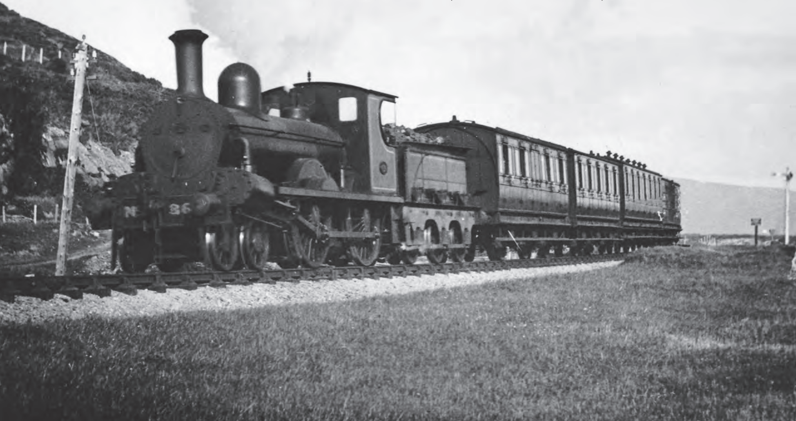
No.36, rebuilt 4-4-0 'Met Tank', on a Machynlleth-Barmouth local between Aberdovey and Towyn, c1920. (MLS/R.W. Miller collection/H.W. Burman)
