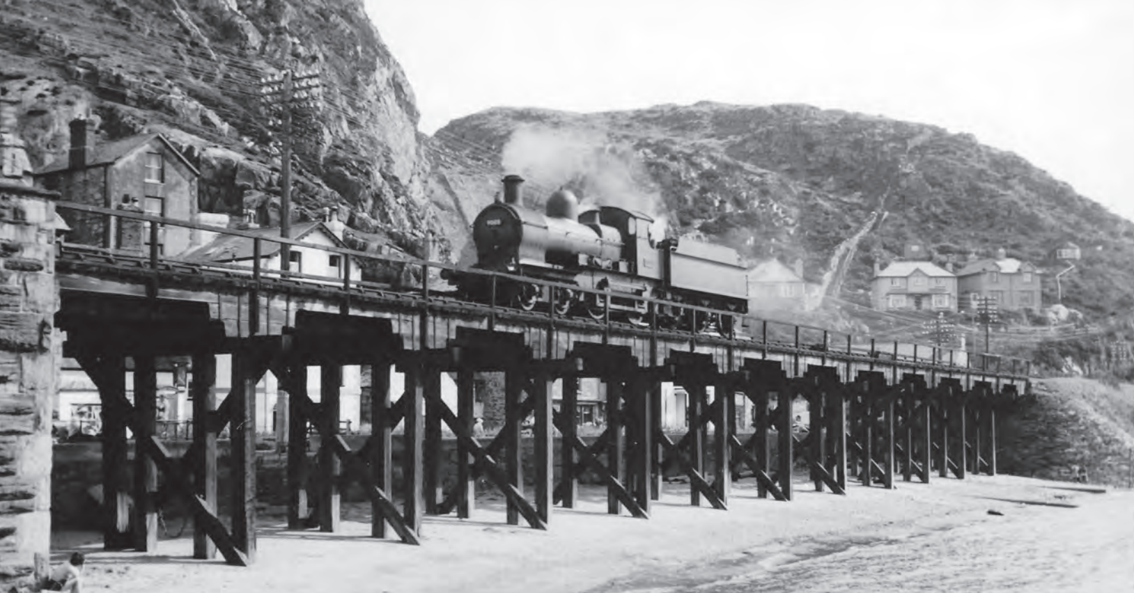
'Dukedog' 9005 runs light engine towards Barmouth station over the wooden trestle Old Chapel Bridge just before it was rebuilt using concrete instead of wood, 21 August 1951. (MLS/N. Fields)
