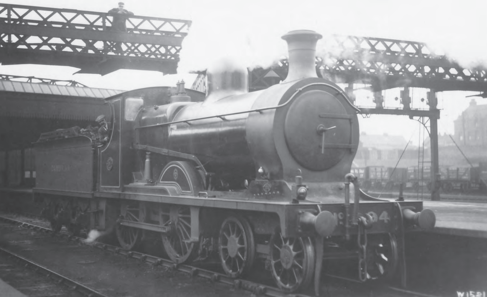
'Large Belpaire' 4-4-0, No.94, at Crewe station after reboiling in 1920. (MLS/R.W. Miller collection/ W.H. Whitworth)
