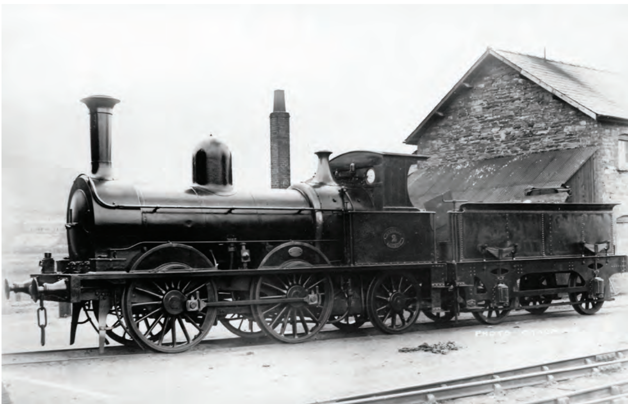
0-4-2, Mid-Wales Railway No.2, built by Kitson in November 1864, which became Cambrian Railways No.2 also when that railway operated the MWR in 1888 and was withdrawn in 1905. It was reboilered at BUILT in 1887, remained on the Mid-Wales section and is seen here at Brecon, c1888. (MLS/R.W. Miller collection)
