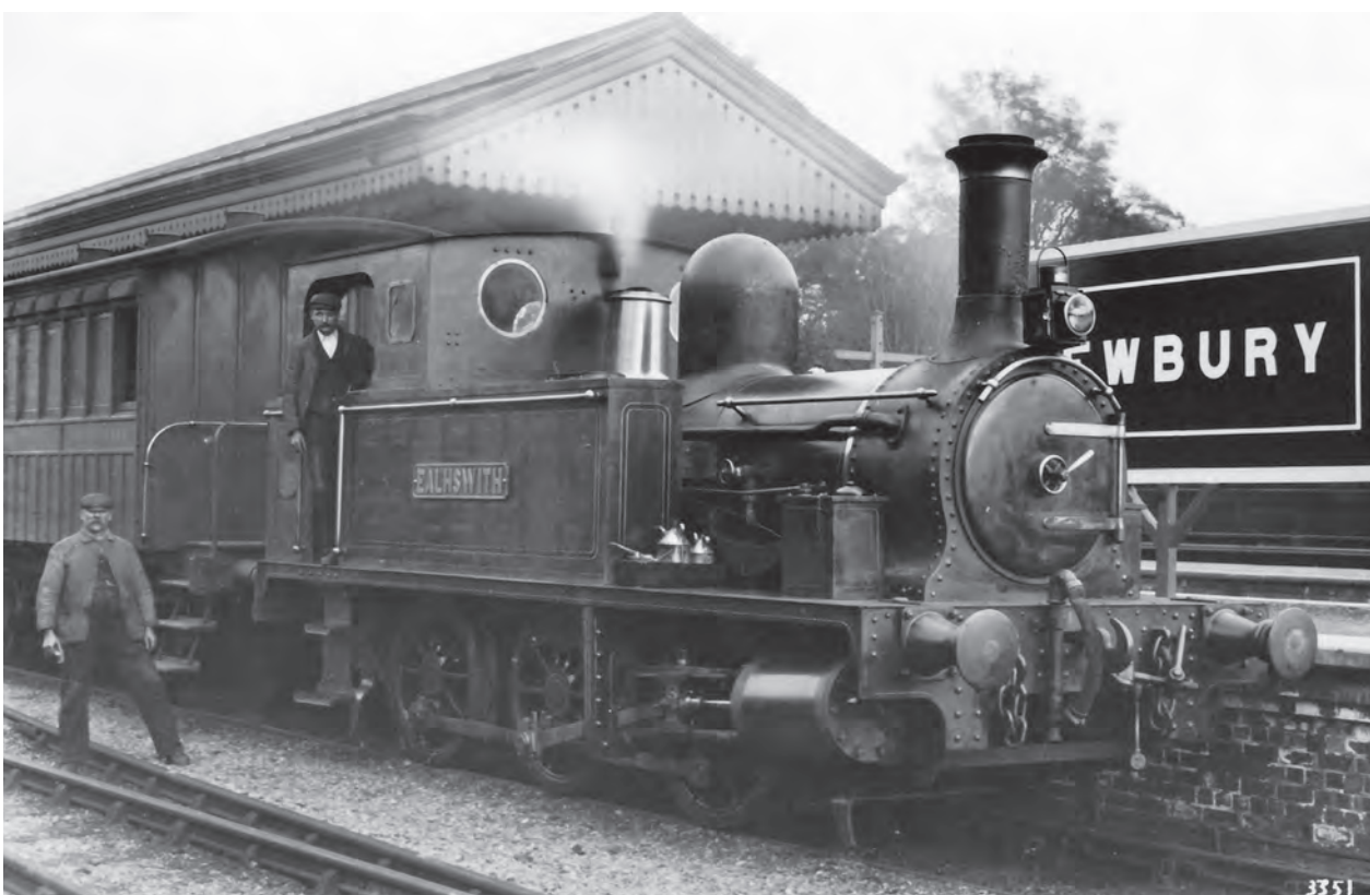
Former Lambourne Valley Railway 0-6-0T Ealhswith built by Chapman & Furneaux of Gateshead in 1898, one of three purchased by the Cambrian Railways in June 1904 for £2,000. It had 12x20in cylinders, 3ft 7in diameter wheels, 150 lb boiler pressure and weighed 23 tons 10 cwt. It was photographed at Newbury, c1900, before purchase, with 1898 built Brown Marshall rolling stock. It was renumbered by the Cambrian Railways as No.26. This locomotive took the number of a scrapped engine, and was later renumbered 820 by the GWR, being sold to Mells Collieries near Frome in March 1931. It was broken up by George Cohen's at Wood Lane in 1945. (MLS/F. Moore)
