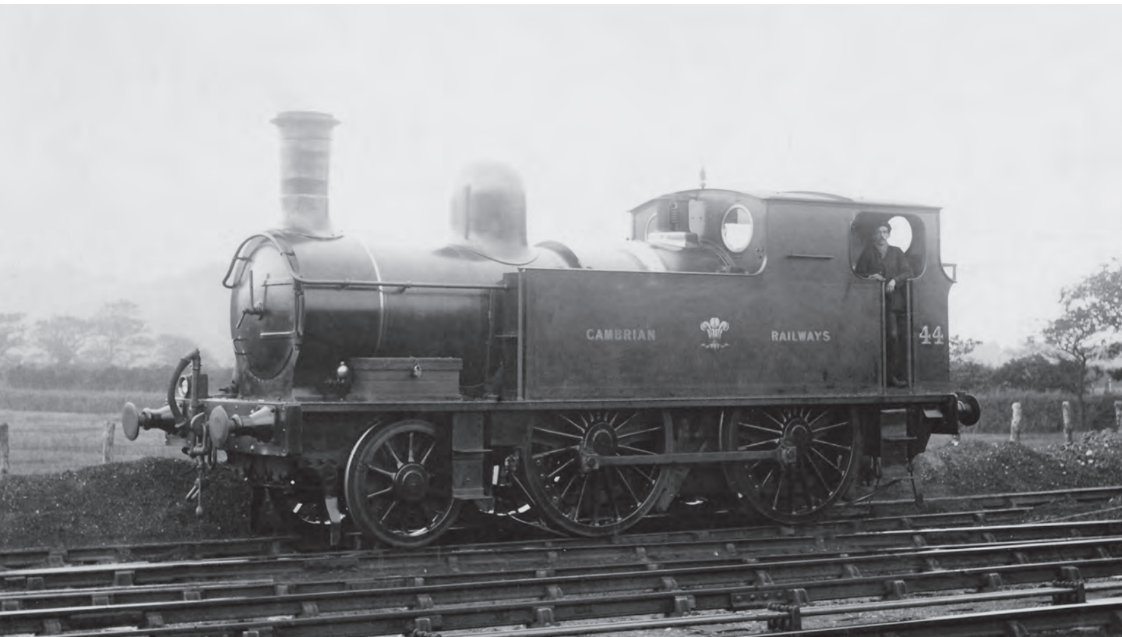
1865 built 2-4-0 No.44 Rheidol , which was placed to store in 1906 and, with No.56, was converted in 1907 at Oswestry Works to a 2-4-0 side tank locomotive for auto-working stopping passenger trains between Machynlleth, Aberystwyth and Barmouth. The frames were extended to hold cab and bunker, but the engine was otherwise unaltered. It was withdrawn in July 1922.
