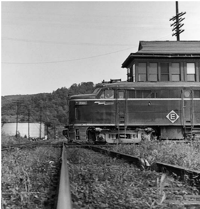
An A-B-A set of Baltimore & Ohio Alco FAs wearing the as-delivered two-tone blue leads a westward freight at Creston in east-central Ohio in the mid-1950s. B&O operated a moderate-sized fleet of Alco FA/FB-2s built between 1950 and 1953. Rated at 1,600 horsepower, these were nominally more powerful than Electro-Motive's F7, which was a more common type on B&O lines in the 1950s. J. William Vigrass
